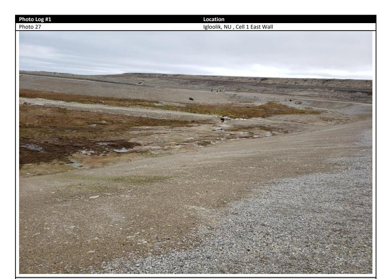
Foreground: Suspected leak of Cell 1 Sewage Lagoon. The leak prompted Spill Report 2021-372. Green streak down the side of the cell wall.
