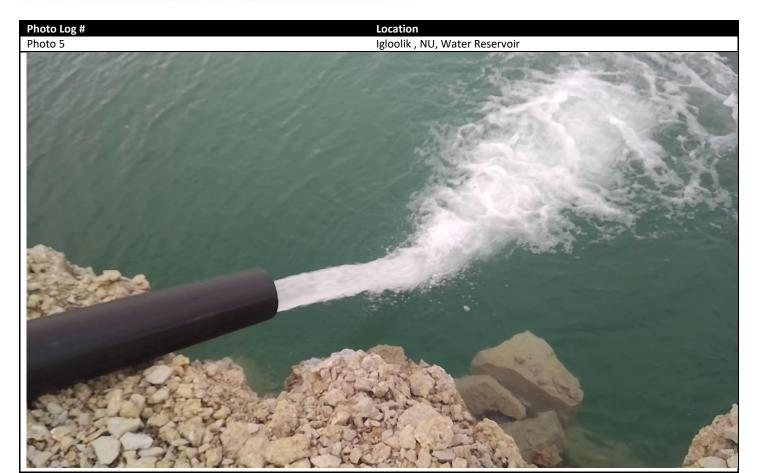
Description: High Water Pressure during the recharge of the Igloolik Water Reservoir is suspected by the hamlet of causing high turbidity. Water level very high in the reservoir.
