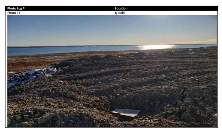
Description: The back side of the open pit burning. Non engineered walls. Fresh Gravel laid over migrating sludge first observed in 2020 inspection report.
