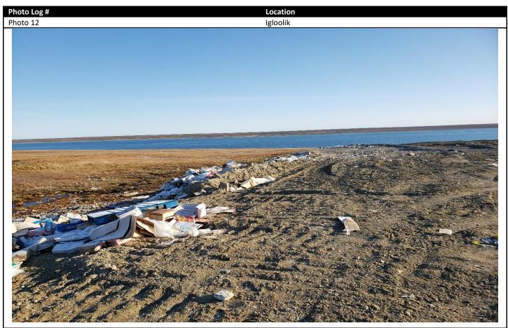
Description: Back side of open pit burning. No walls to contain waste. Ocean visible downgrade from exposed wall of burn and cap. Fresh gravel was place down on top to mitigate the spread of any windblown debris.
