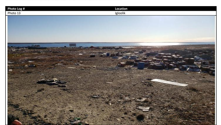
Description: Hazardous Waste Area #1, Old Waste Oil Drums within a bermed area – berm is full. Wall was taken down to allow for access. Drums being deposited there are being deposited further and further away from the bermed area. Water puddles litter the area, and the natural contours of the areas allow for migration into the hazardous waste area, then drains to a small pond downgrade of this site before reaching the ocean visible in the background of photo..
