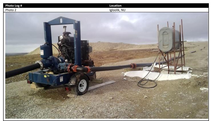
Description: Second water pump (mobile), connects half way from water source to water reservoir to aid in the recharging of the water reservoir. A berm was installed to house the fuel tank when operating.
