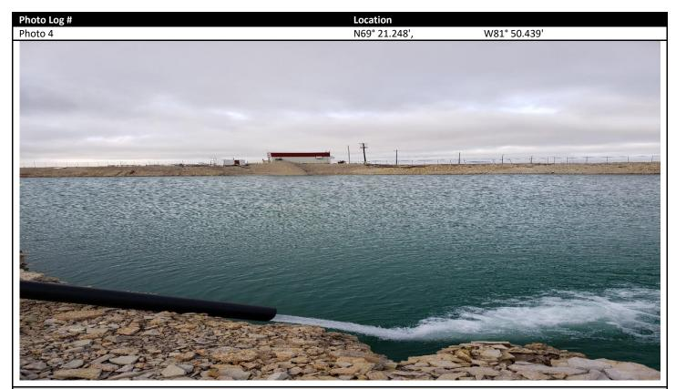
Description: Water Reservoir, recharge pipe in the foreground. Old pump house (left) in the background, decommissioned, but still operational in case of emergency. New Water Treatment/Pump Station/(right). Water Reservoir recharging at the time of inspection.
