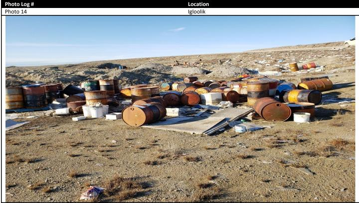
Description: signs of Water around the hazardous waste disposal area. Surface water migrates from background of photo to within hazardous waste storage facility.
