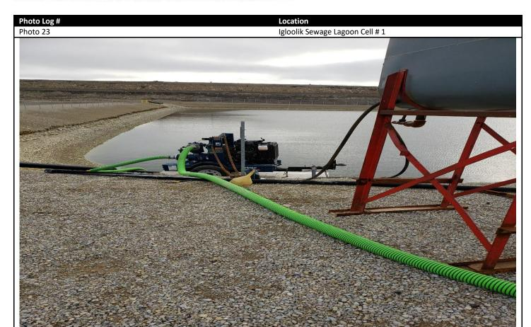
Description: Decanting at the Cell#1 Lagoon. Structural Integrity possibly compromised. Doubled walled storage tank to fuel a high intensity water pump.
