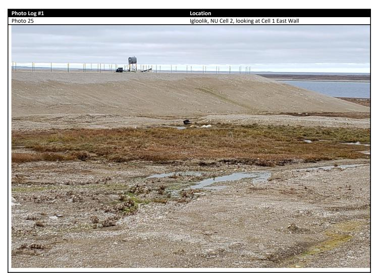
Background: Cell 1 East side of the sewage lagoon's wall. Source of suspected leak that prompted Spill Report 2021-372. Green streak down the side of the cell walls. October 26, 2021
