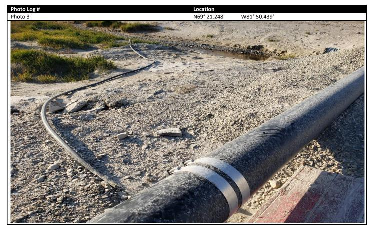
Description: The bypass hose installed at the low point, to bleed out any still water from freezing when not in use. GPS Coordinates: Latitude 69° 21.248'N, Longitude 81° 50.439'W.
