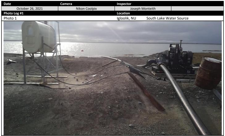
Description: South Lake Water Source. Water pump pipe end submerged held up by buoy. No indication of fish mesh screen. The 909 Litre storage tank, connected in non engineered secondary containment as well as the high pressure water pump.
