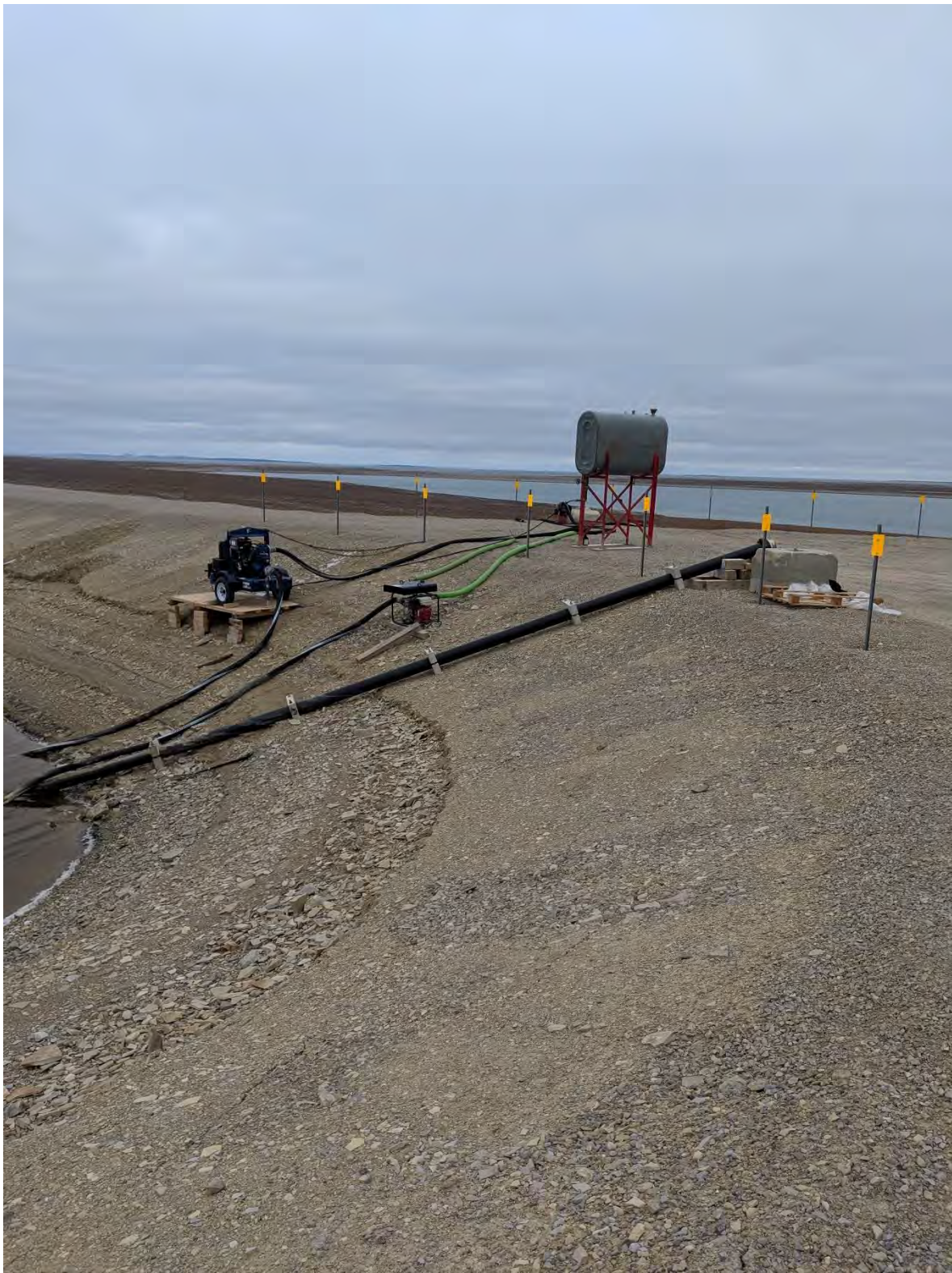
Photograph #2: Pumping operations.
