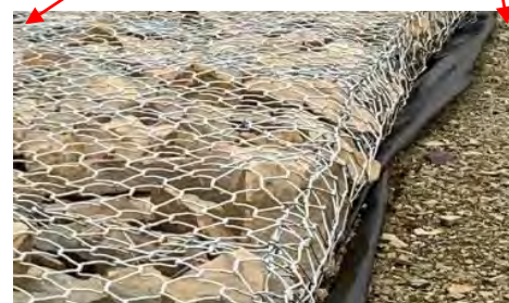
Riprap Downstream Slope - Details
