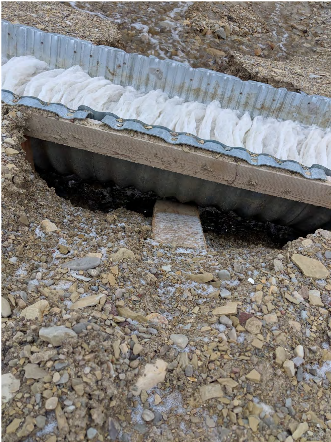
Figure 4: One of several washouts along the drainage trough.
