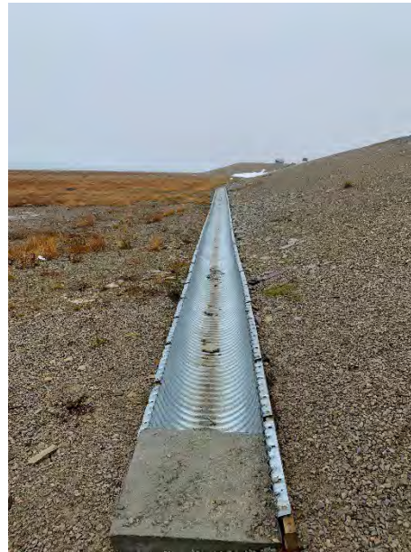
Dry condition at the end of the drainage trough.
