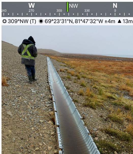
Water level in trough reduced to a dry condition at about 1/3 of the trough
