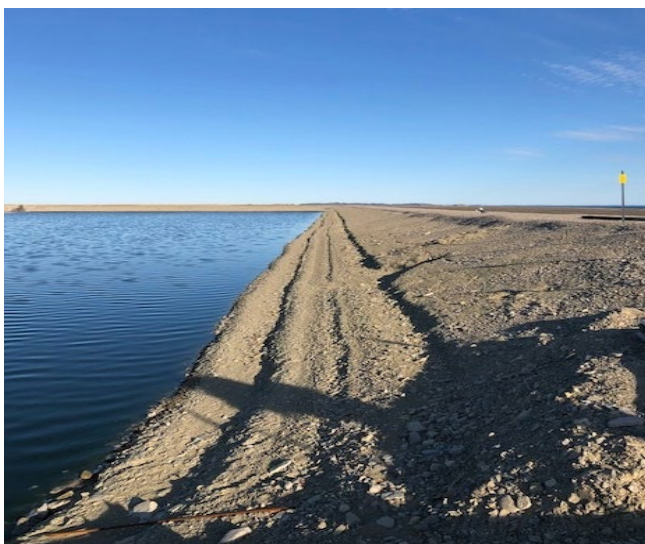
Collapsing interior berm soil within cell “A”
