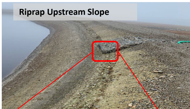
Riprap Upstream Slope - Details
