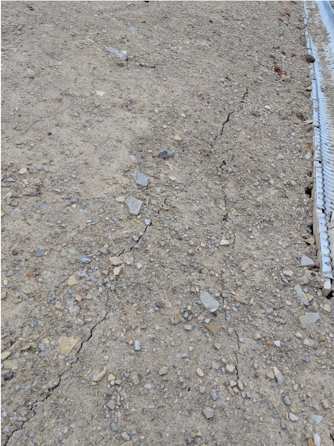
Photograph #1: Settlement Cracking of the soil around the lagoon.
