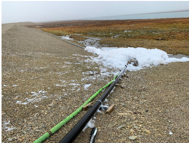
Decanting pump in operation Downstream - Outlet
