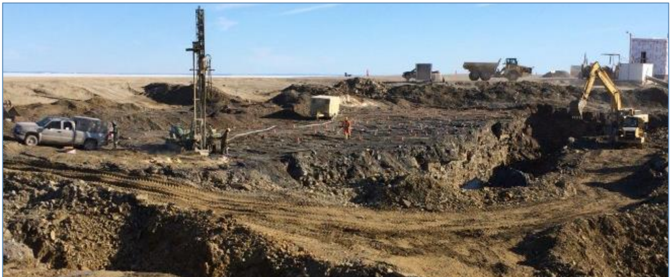
Photo 3: Drilling into the rock material to be blasted
