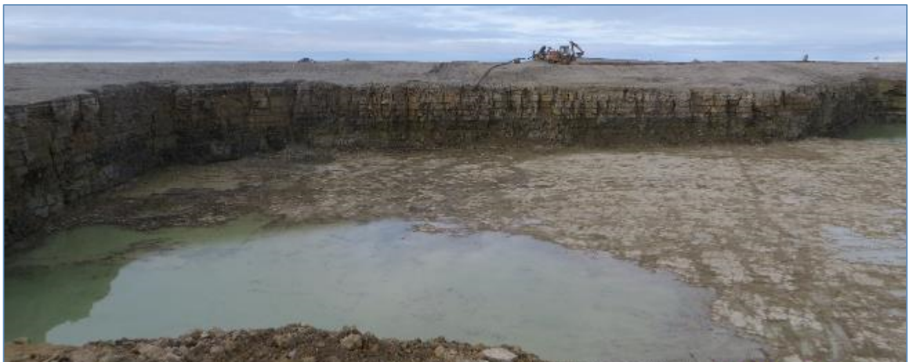
Photo 6: Reservoir base and walls in 2017
