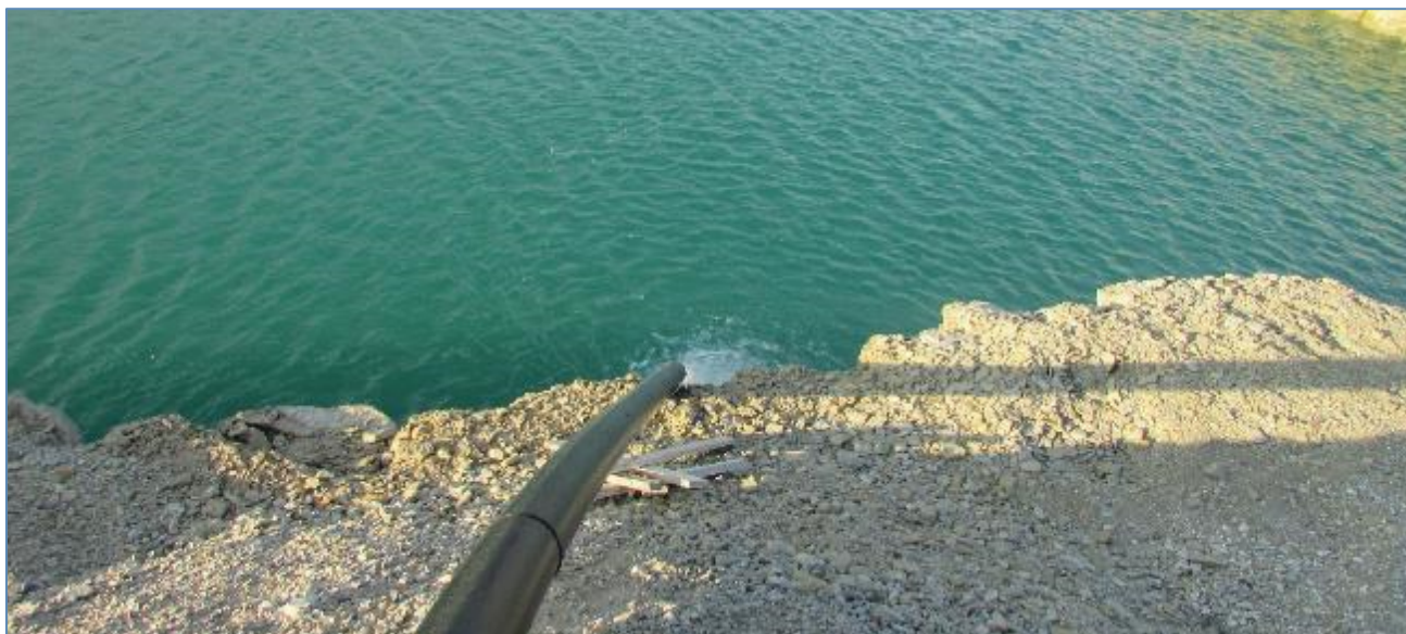
Photo 2: Water supply line discharging at the water reservoir
