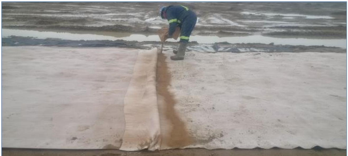
Photo 7: Connecting GLC segments
