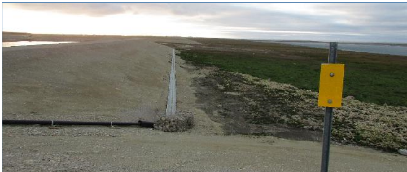
Photo 4: Distribution trough at the head of the vegetative filter strip wetland
