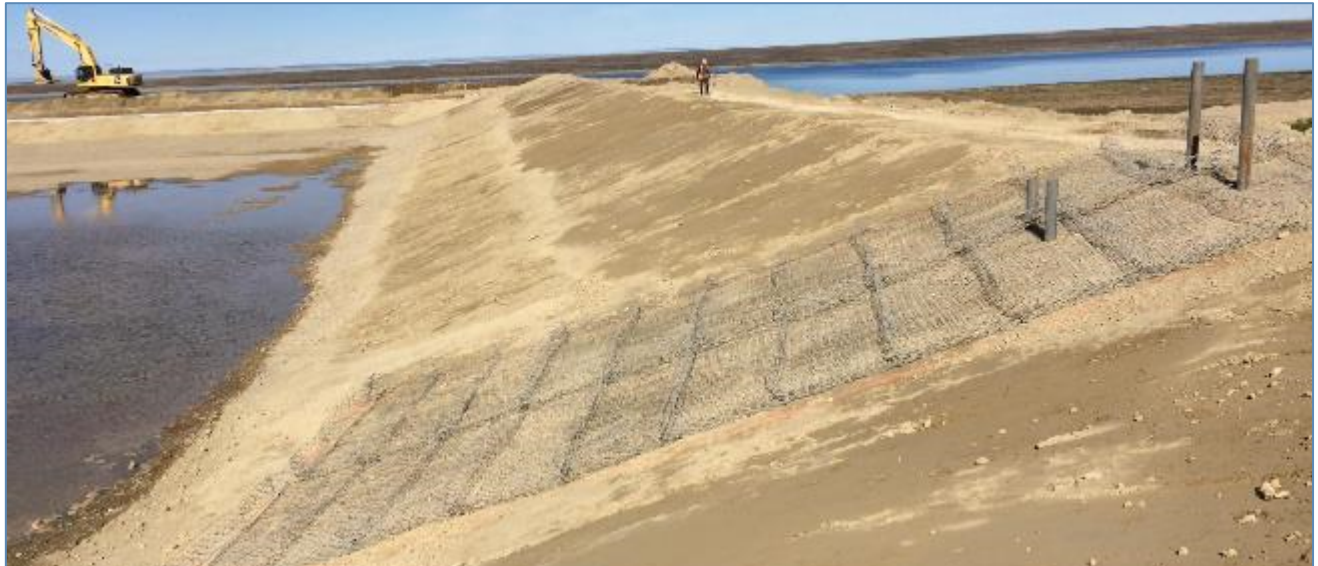
Photo 12: Gabions installed for a discharge chute
