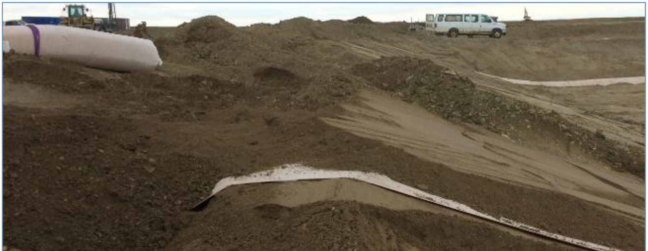
Photo 9: Cell B key to anchor GCL liner
