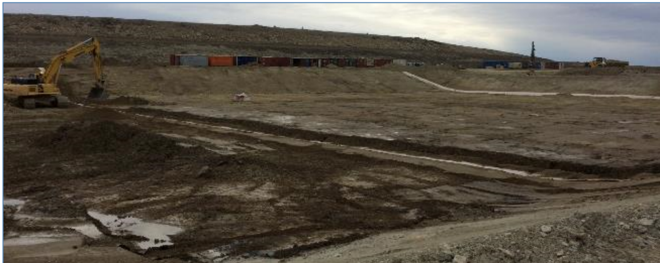
Photo 10: Cell B base construction
