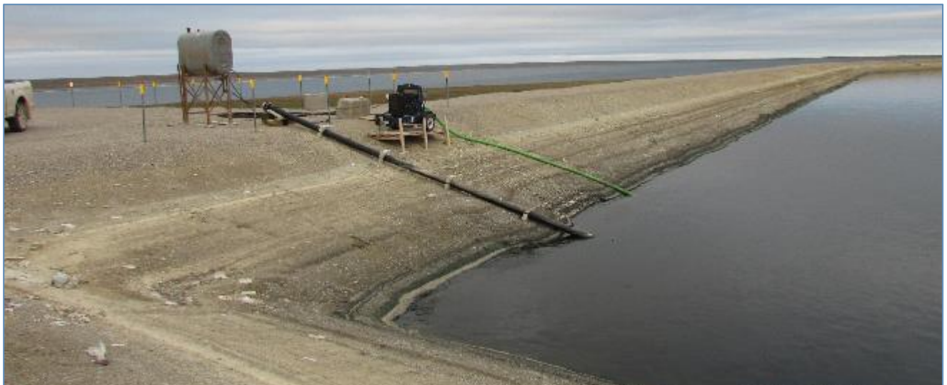
Photo 3: Decanting operations
