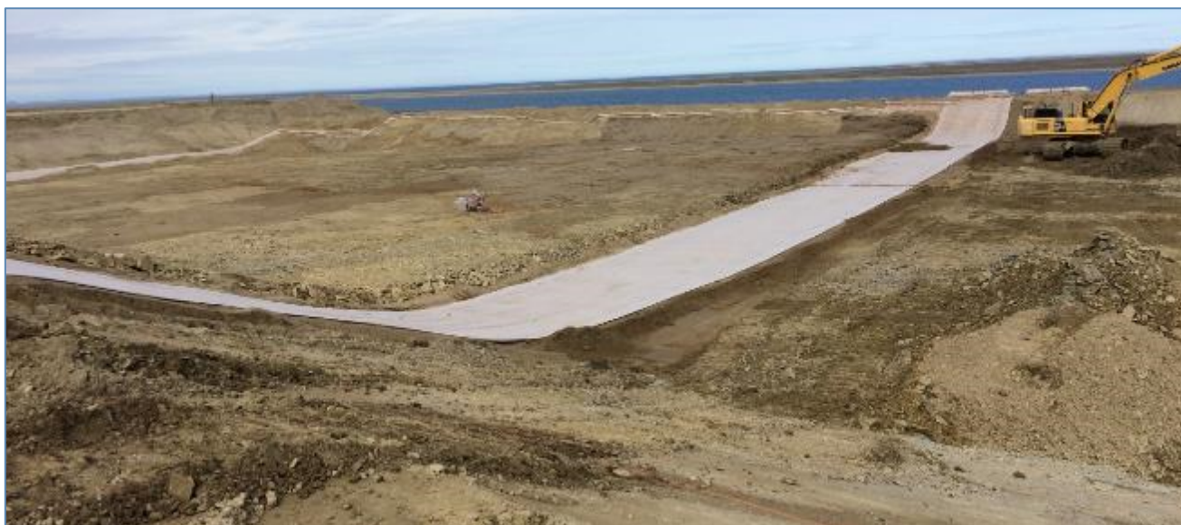
Photo 11: Cell B GCL liner installation
