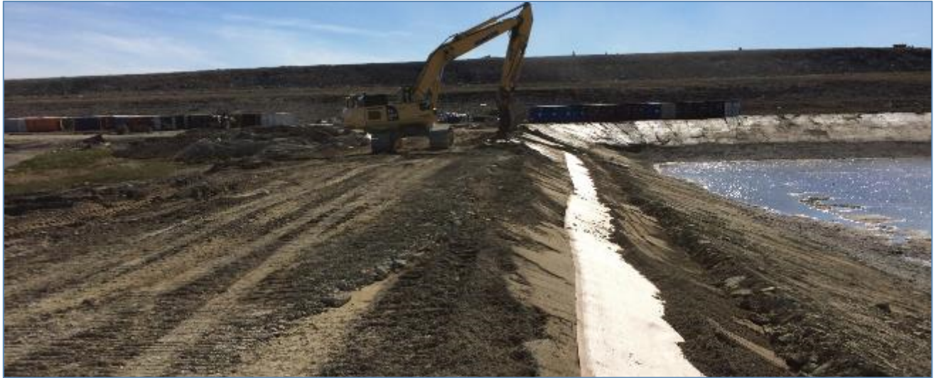
Photo 8: Cell A berm construction
