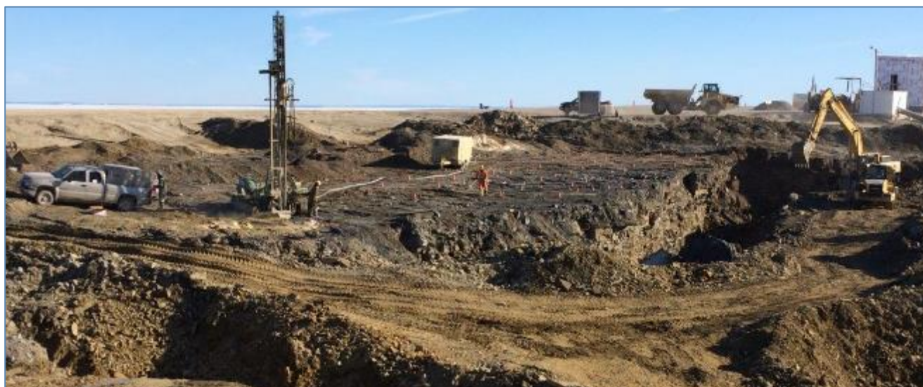
Photo 3: Drilling into the rock material to be blasted
