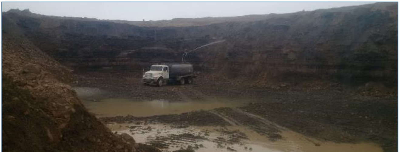
Photo 5: Pressure washing the reservoir wall
