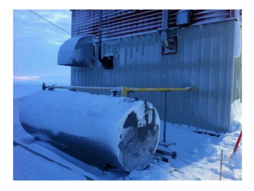
A second, smaller tank 227Liters (50 Gallon imp.) is located near the boiler and holds enough fuel to supply the furnace and the back-up generator.
