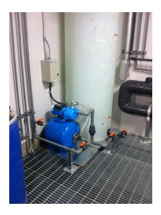
The domestic water pump is a self-contained automatic pump. When water is demanded, it maintains water pressure for service sink, cleaning hose, chlorine tank filling, etc.
