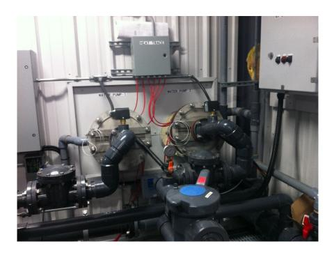
Each HTC to control: two heat trace cables and three RTD temperature sensors. There are three sensors per intake pipe: at 15 meters and at 30 meters.
