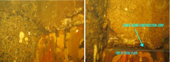
The photos below show the sealant in the expansion joints. This sealant does not go beyond the new concrete. The photos clearly show that there was no sealant in the joint previous to the placement of the sealant shown. All of the expansion joints look like this. More visual evidence can be seen in the video that was produced.
