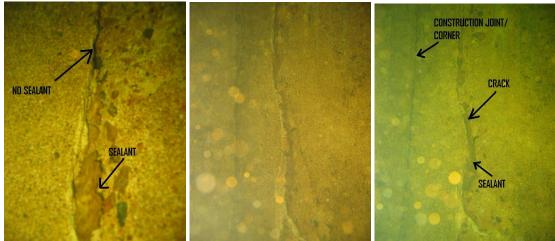
The top of the crack starts at the construction joint between the old concrete and the newer addition. It runs almost parallel with the construction joint in the corner down to
