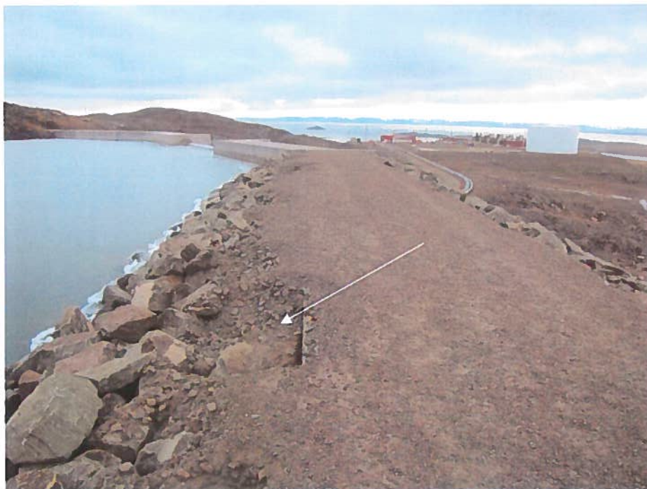
North Berm Localized Wave Scour; 2010.
