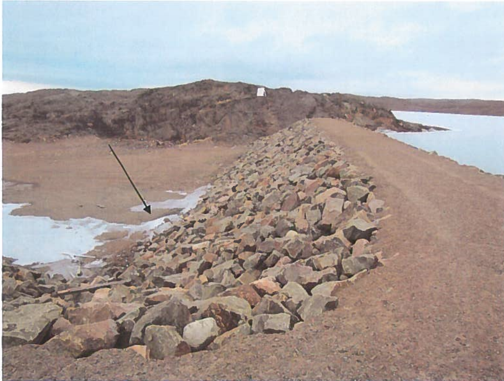
Photograph 2 Overview of North Berm, Downstream Face. Note leakage just north of ramp access.
