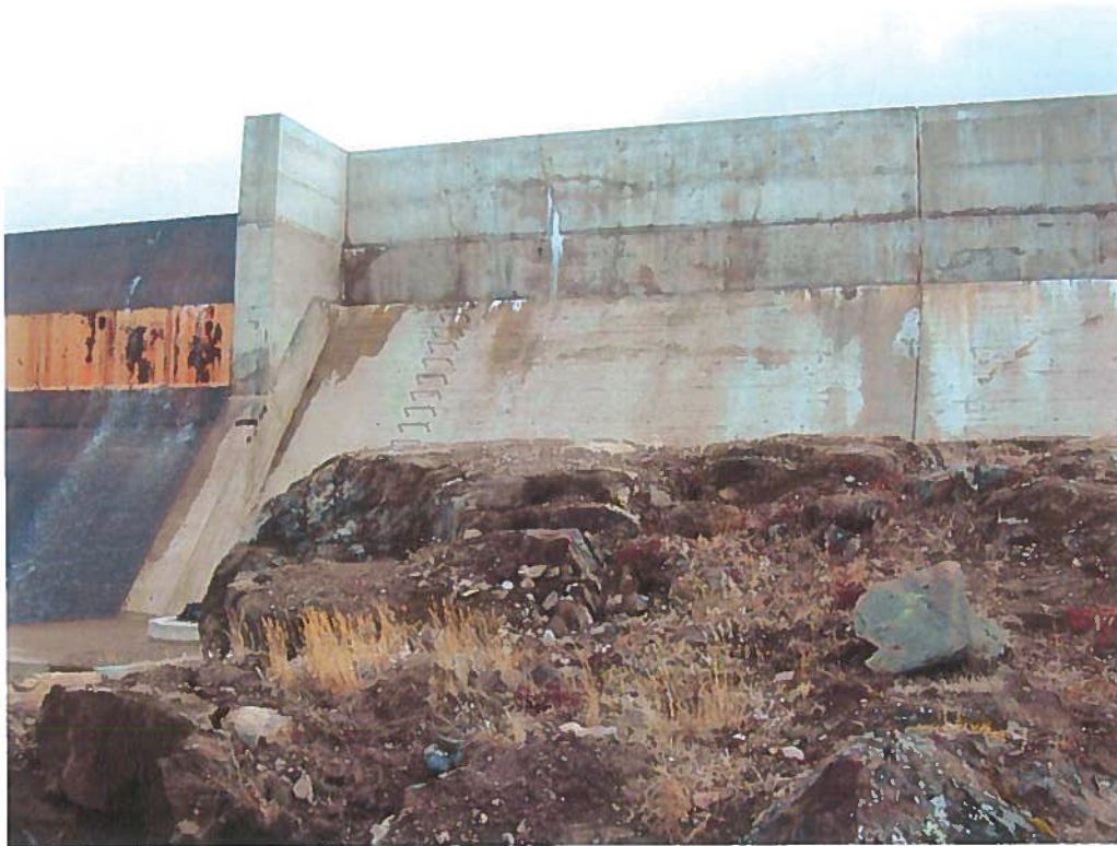
Photograph No. 8 – Overview of southern portion of Spillway section, and south Gravity elevation. Note leaching cracks in Gravity face.
