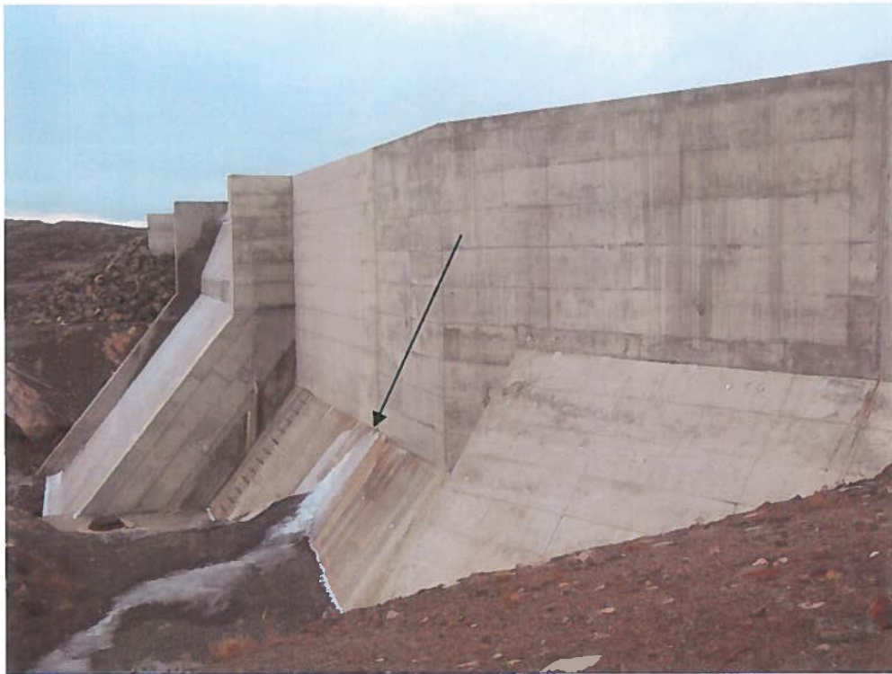
Overview of Downstream Face; 2010; Note Leakage (at arrow)
