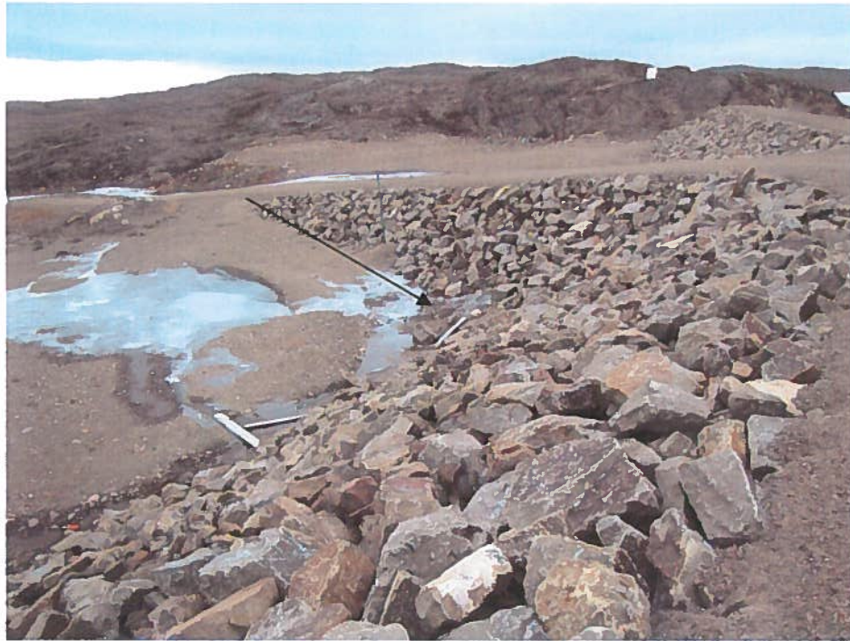
Photograph 3 North Berm at South side of ramp access; note leakage.
