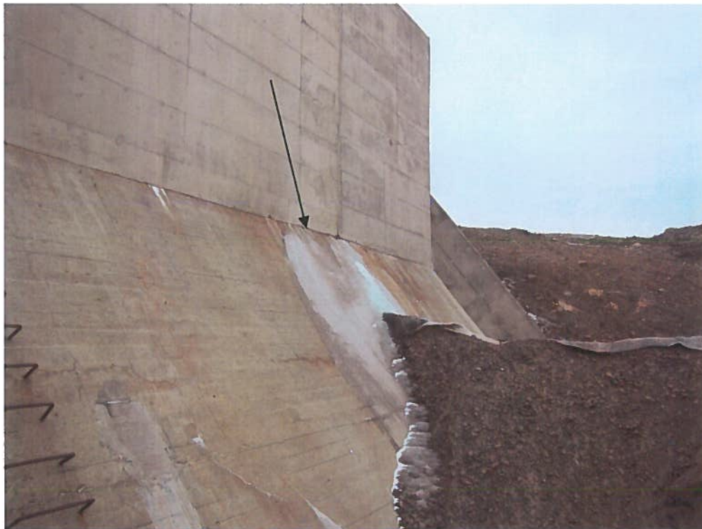
Photograph 8 Leakage at South Gravity section; Similar to 2009 DSI.
