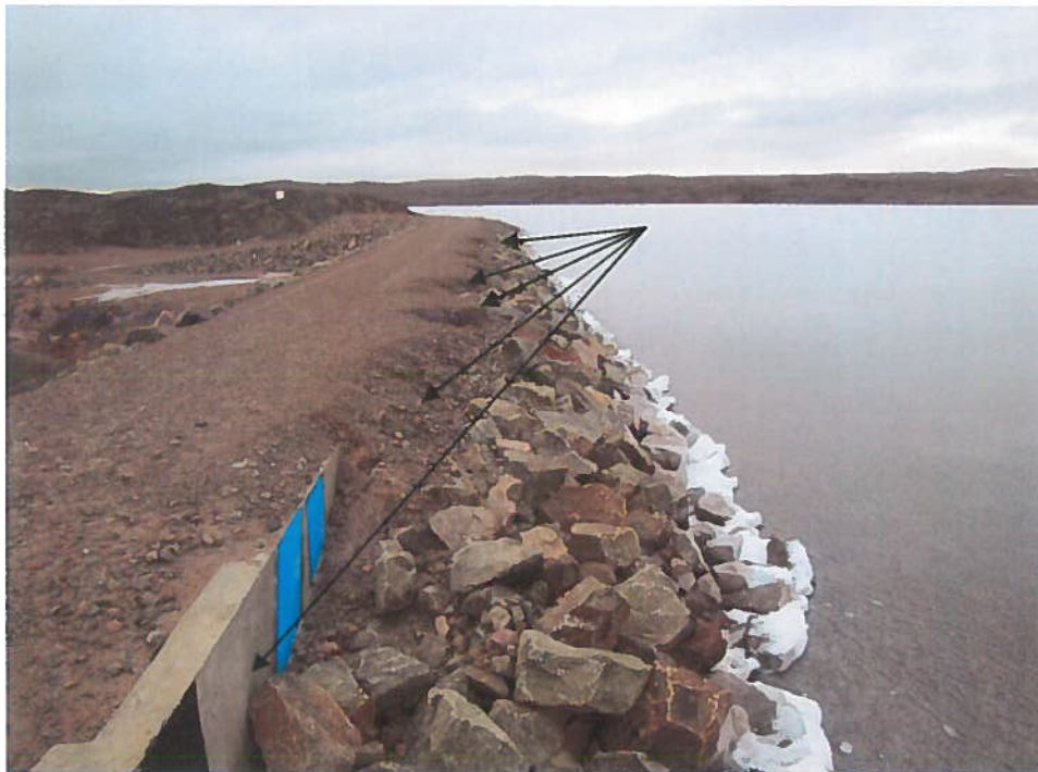
Photograph 4 Southern portion of North Berm, upstream face; note localized washouts due to wave action.
