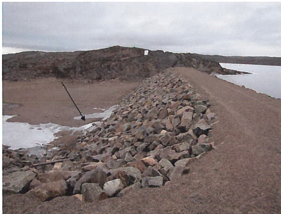
Photograph 2 Overview of North Berm, Downstream Face. Note leakage just north of ramp access.
