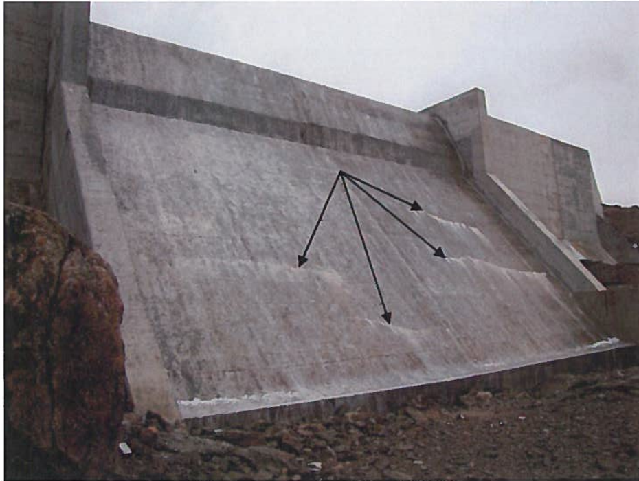
Photograph 7 Leaching cracks in Spillway face; Similar to 2009 DSI.
