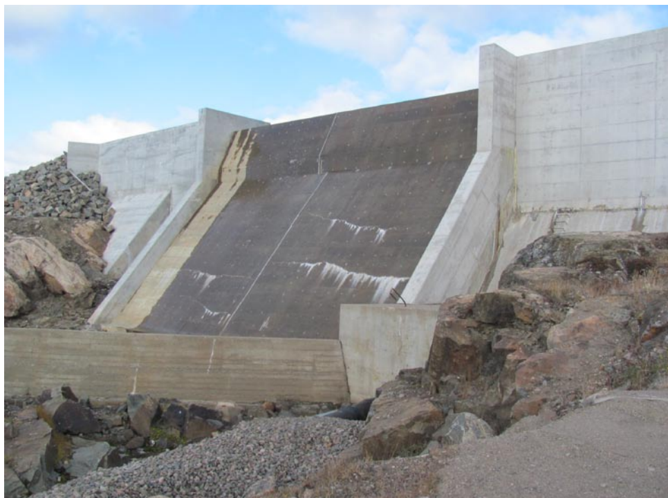
Photograph 2 Overview of spillway – note overtopping (maximum lake level)
