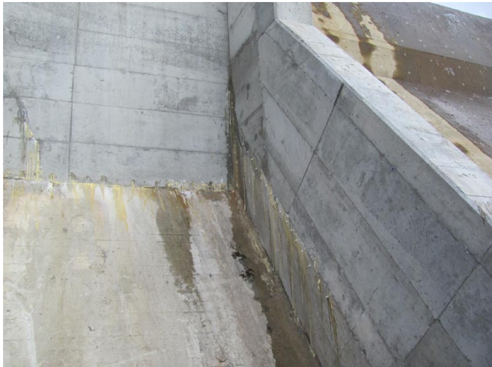
Photograph 3 2011 grouting repair area – concrete is damp only with no running water.
