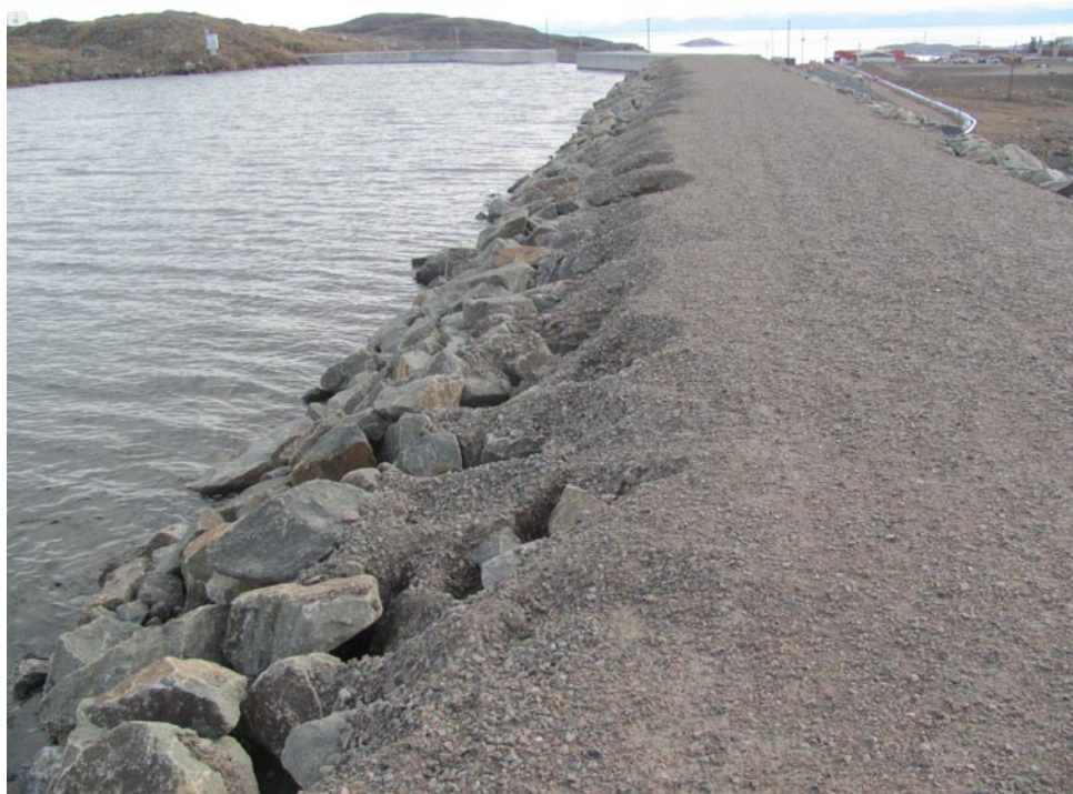
Photograph 4 Overview of North berm – note extensive loss of material from wave action.
