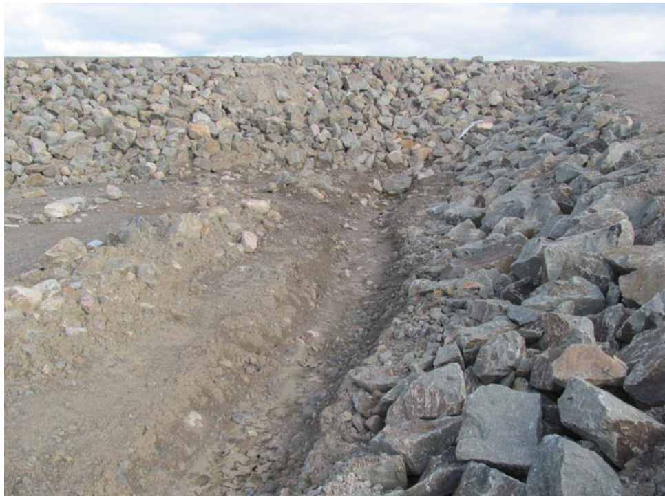
Photograph 5 North side of access ramp – note previously wet area now dry.
