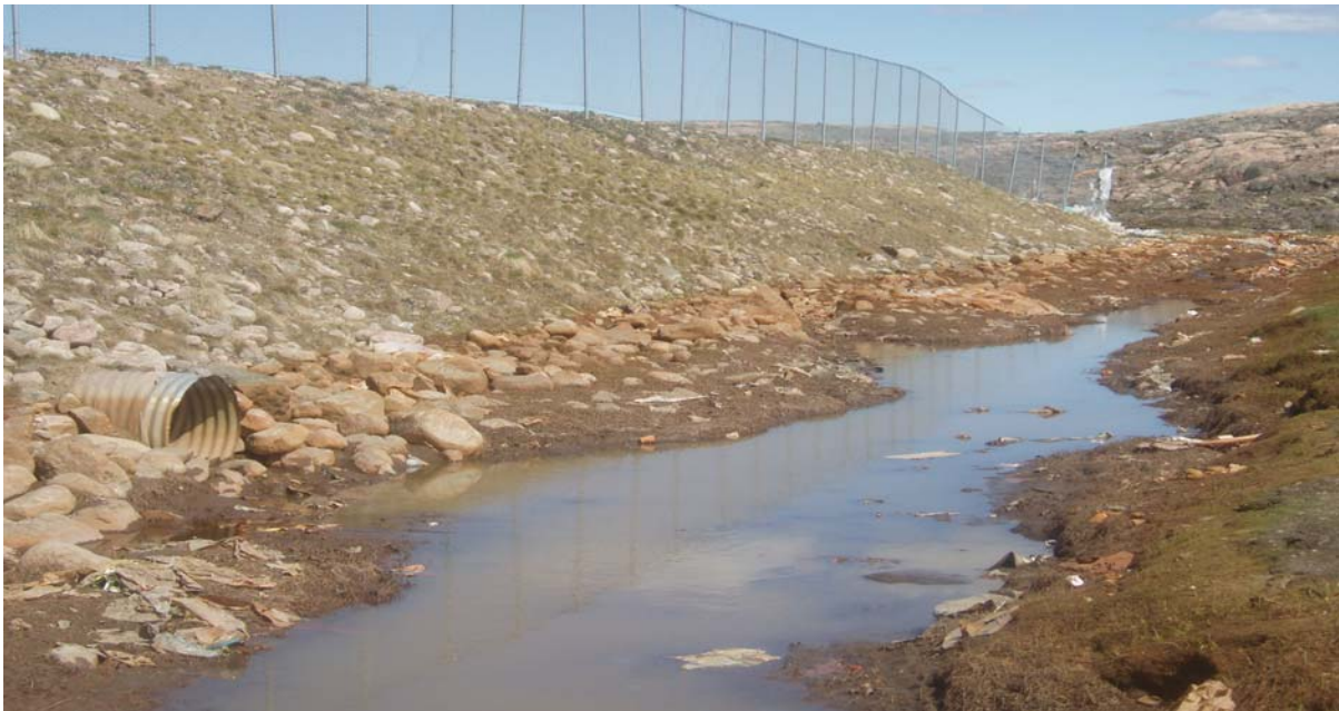
Picture 2 – Berm adjacent to South pond – Culvert to be sealed with fillcrete
