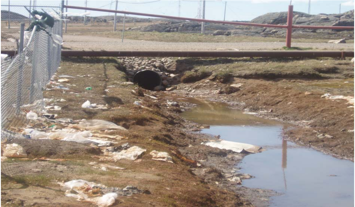
Picture 3 – Culvert crossing road south of site – New piping to be laid through this culvert to Run-off
