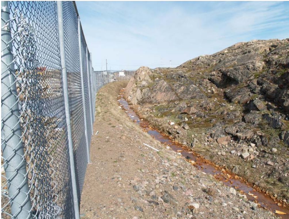
Off site runoff management control system on north side of the landfill site (view to northwest)
