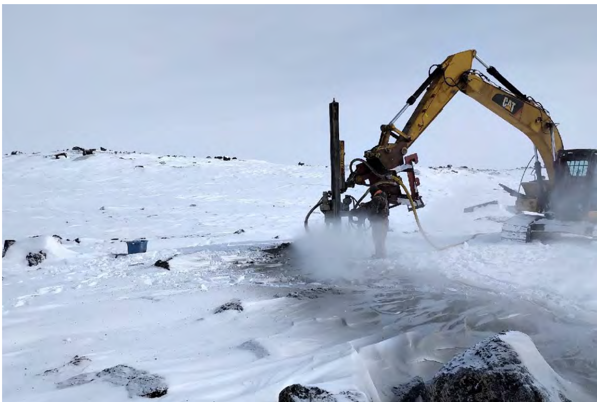
Photo 3 – Borehole Drilling Operation - Typical
