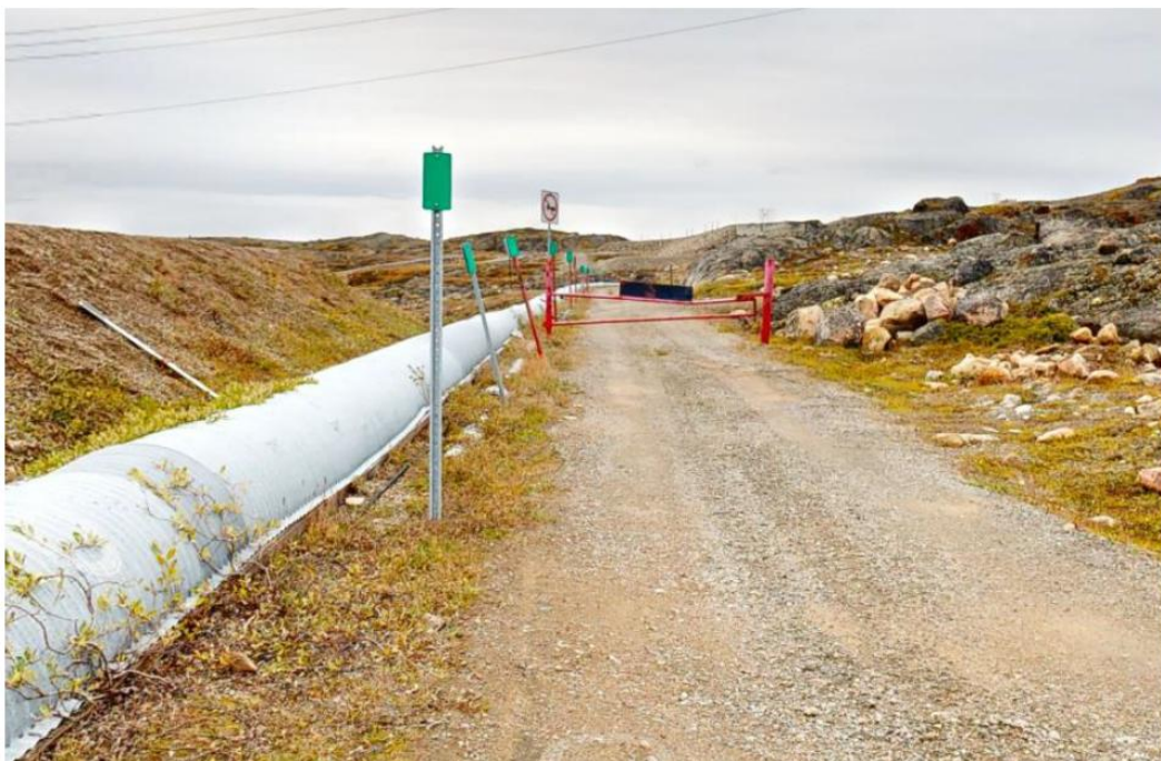
Figure 3.4 Access Road between the WTP and Lake Geraldine Access Vault
