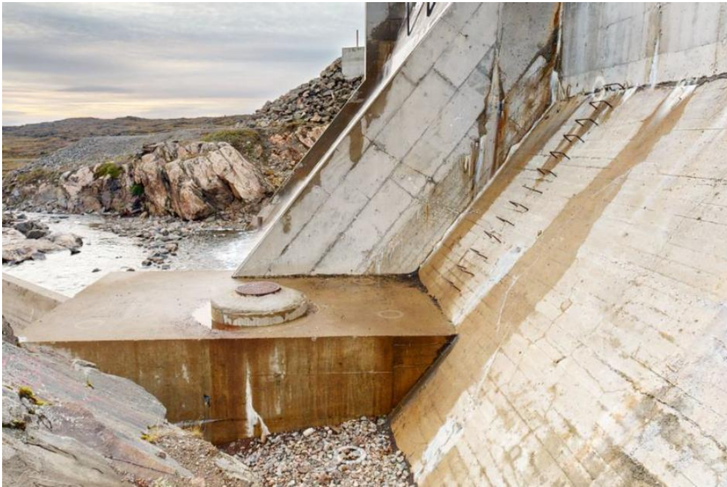
Figure 3.3 Lake Geraldine Access Vault (WSP, 2024)
