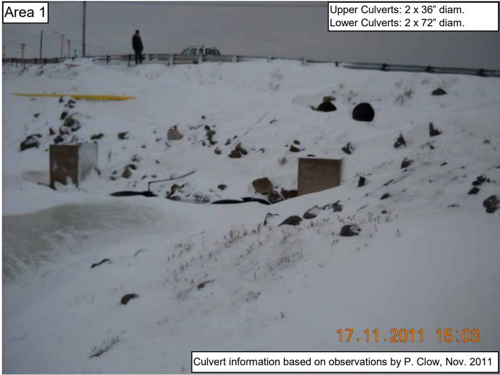
Saputi Road Crossing (looking downstream).
