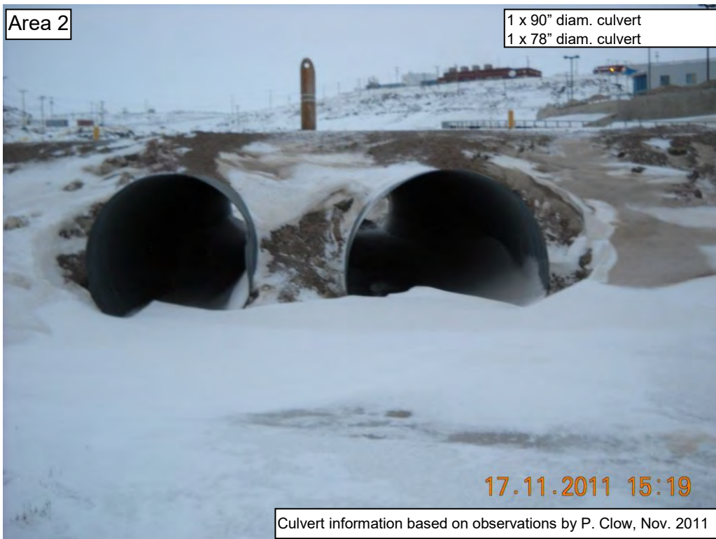
Niaqungusiariaq Road Crossing (looking upstream)
