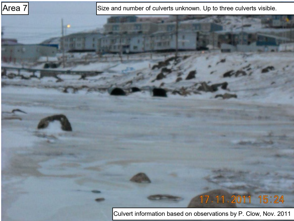
Pedestrian Crossing (upstream of Astro Hill Terrace Bridge Crossing)
