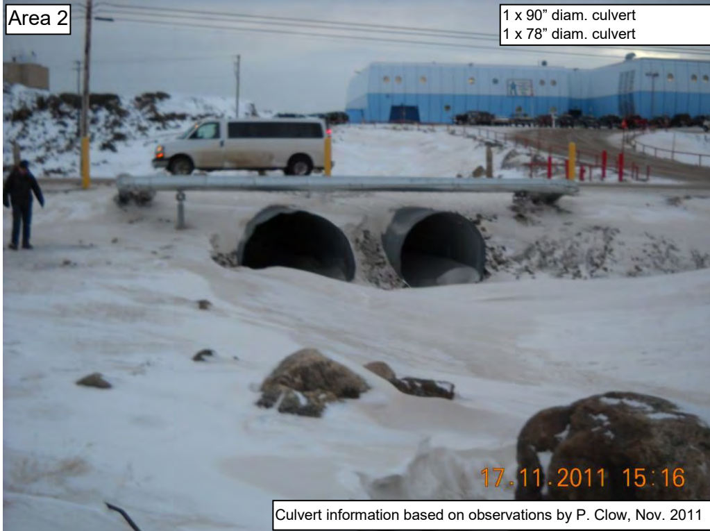
Niaqungusiariaq Road Crossing (looking downstream)
