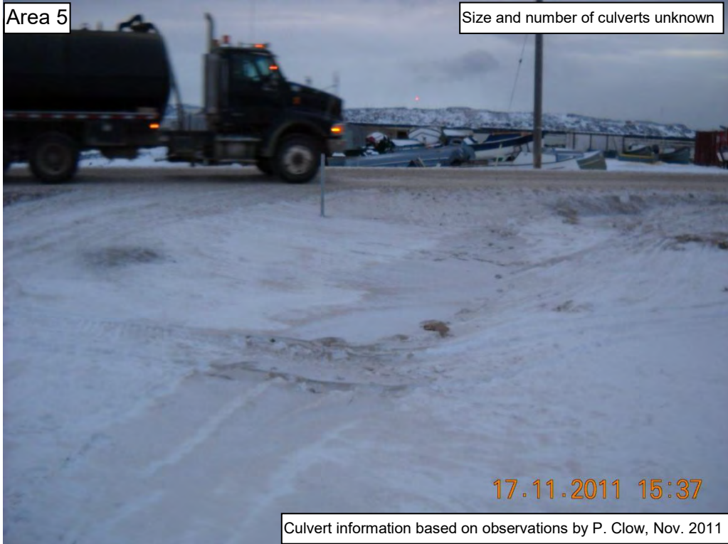
Sinaa Street Crossing (looking downstream)
