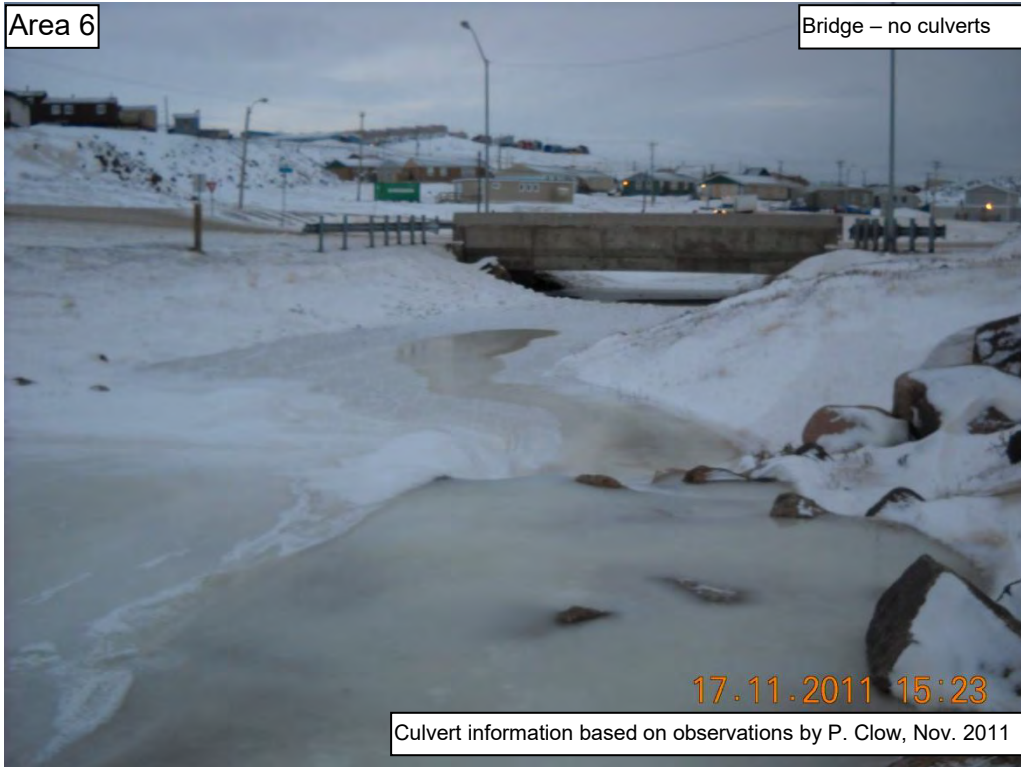
Astro Hill Terrace Bridge Crossing (looking downstream)
