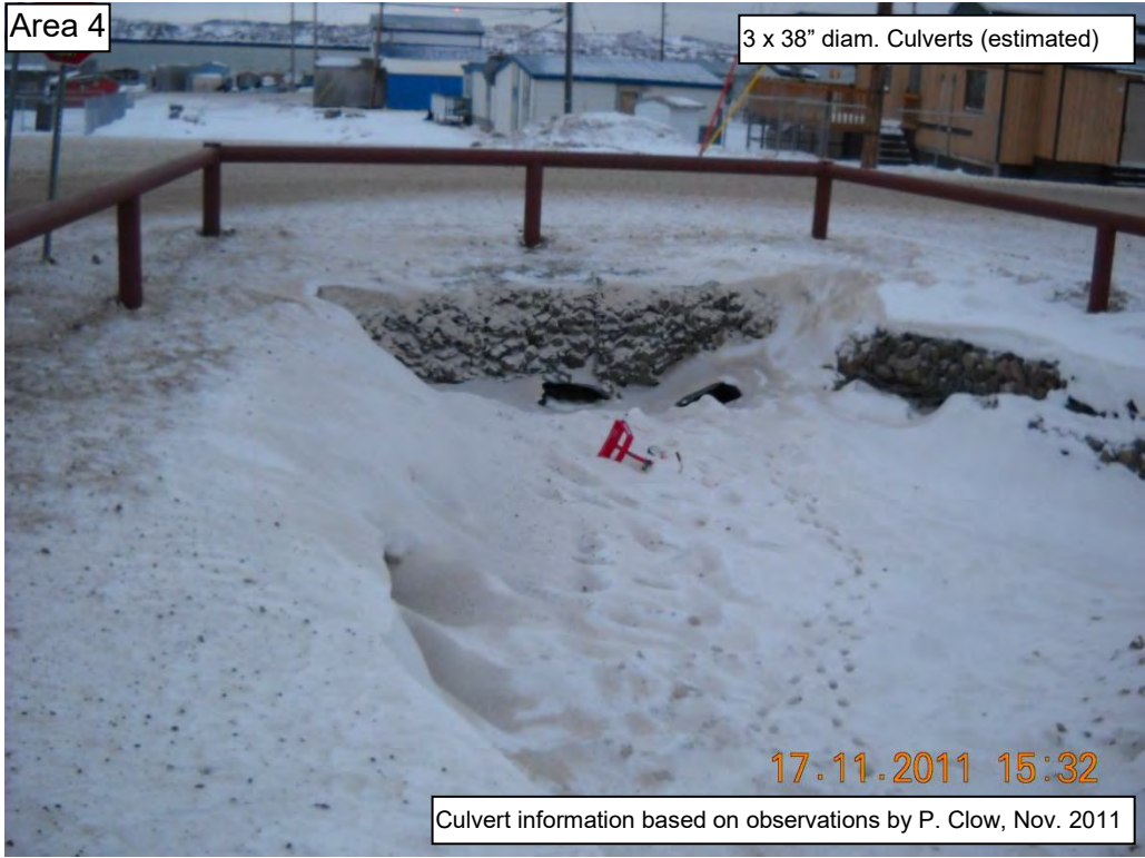
Nipisa Street Crossing (looking downstream)
