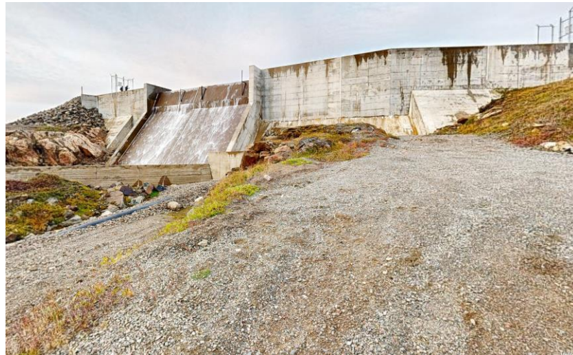
Figure 3: Lake Geraldine Dam Structure
