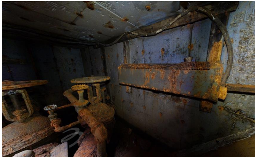
Figure 13: Existing Electrical Radiant Heater Along West Wall
