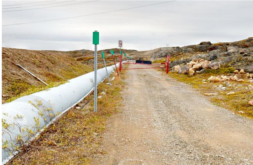
Figure 4: Access road between the WTP and Lake Geraldine Access Vault
