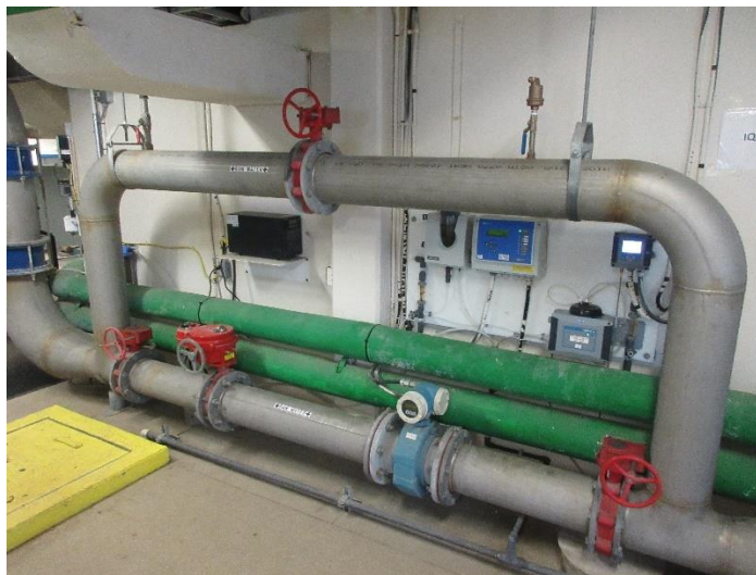
Photo 3.1: Proposed location for new RP backflow preventer
