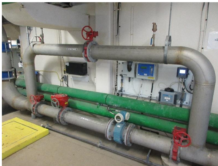
Photo 3.1: Proposed location for new RP backflow preventer
