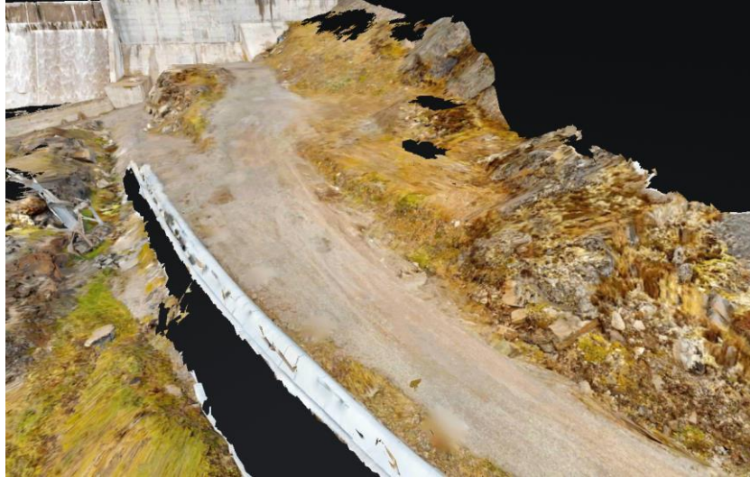
Figure 6: Matterport Aerial Rendering of Access Road approaching Lake Geraldine Dam (2023)
