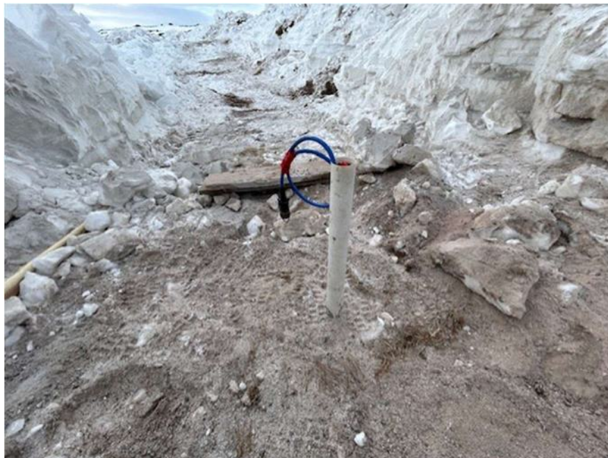
Photograph 2 – May 2, 2025 Thermistor installed in APEX2025-05.
