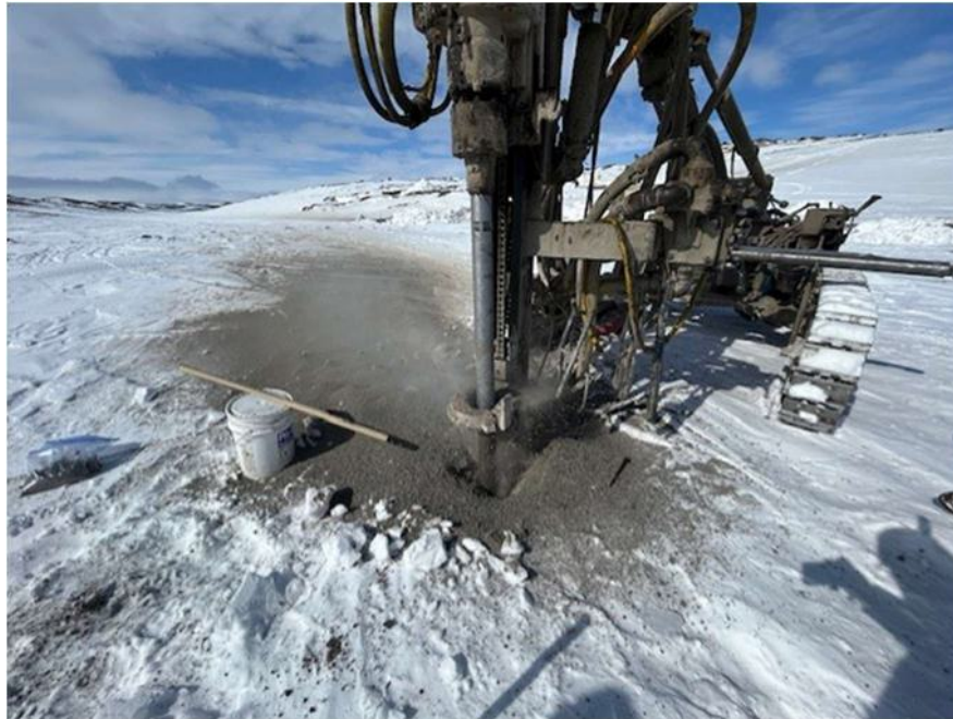
Photograph 3 – May 3, 2025 Drilling APEX2025-02.
