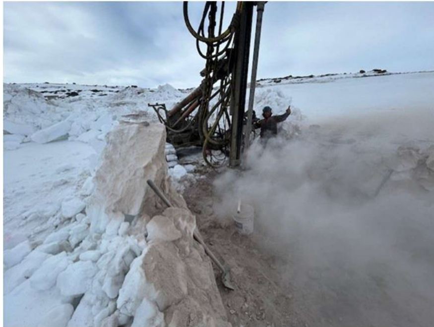
Photograph 1 – May 2, 2025 Drilling APEX2025-05.
