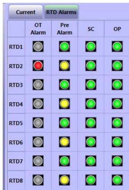
RTD Faults and Alarms
