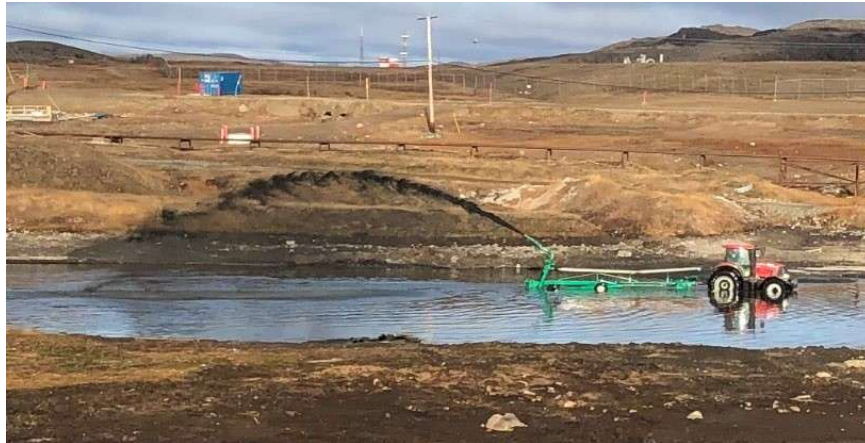
Figure 6 Mixing of Lagoon Supernatant and Settled Sludge during Desludging
