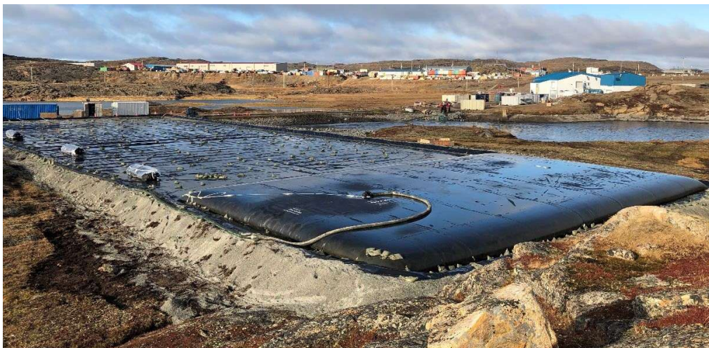
Figure 7 Desludging of Sewage Lagoon using Geotubes placed on Containment Pad
