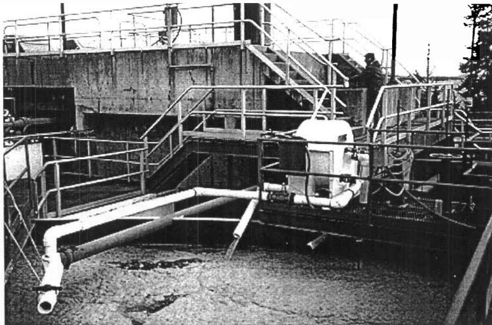
Pilot Installation of PRA Micro-Screen
