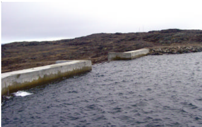
The dam on Geraldine Lake permits control of water and increases the lake's volume. The City will likely need to increase Iqaluit's raw water source in years to come.
