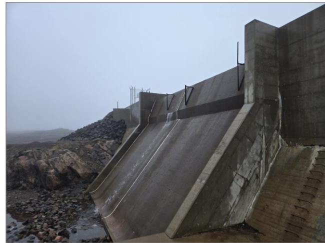
Figure 32 Spillway Conveyance and Training Wall
