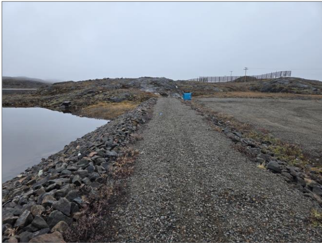
Figure 10 Crest of South Berm
