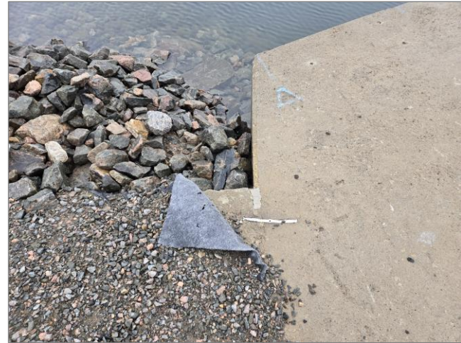
Figure 43 Waterstop at Center Berm Corewall - North Concrete Dam Interface
