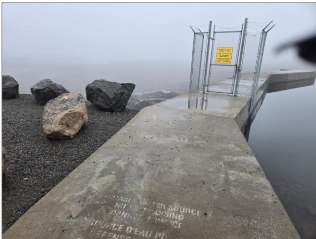
Figure 26 Left Abutment of South Concrete Dam
