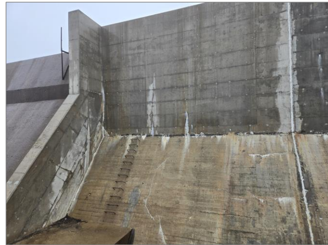
Figure 31 South Concrete Dam Intake
