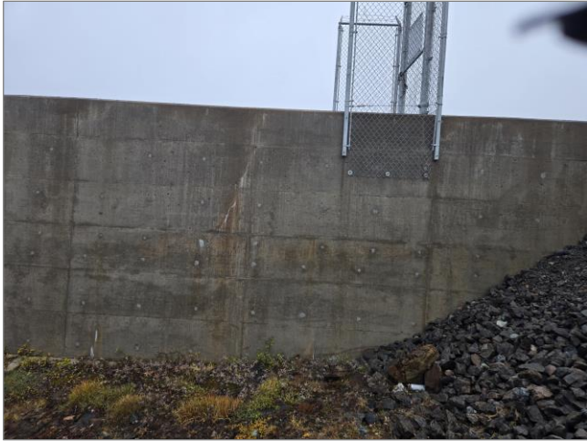
Figure 29 South Concrete Dam, Downstream Face
