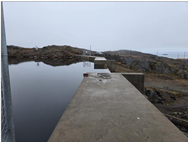
Figure 42 View across Crest. Unknown Sensor
