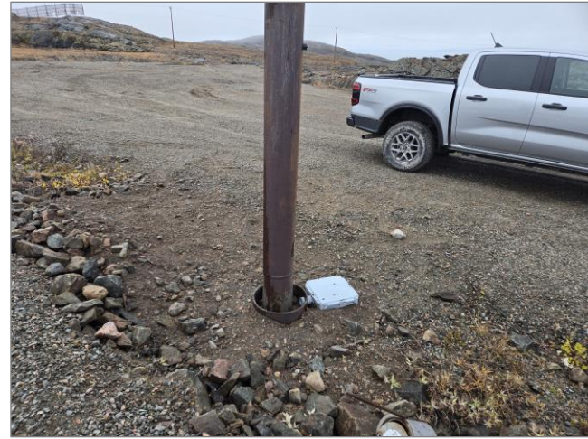
Figure 23 South Berm, BH111 Thermistor
