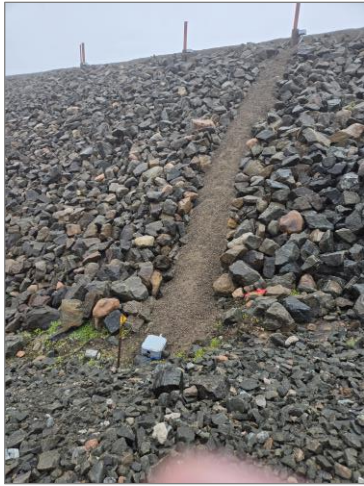
Figure 21 BH109 Thermistor, Rock Slope
