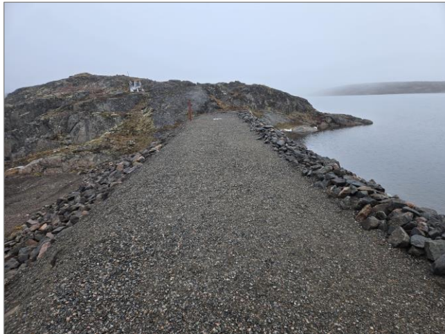
Figure 2 North Berm Abutment
