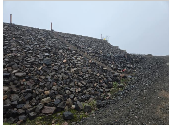
Figure 8 Downstream Rockfill Slope
