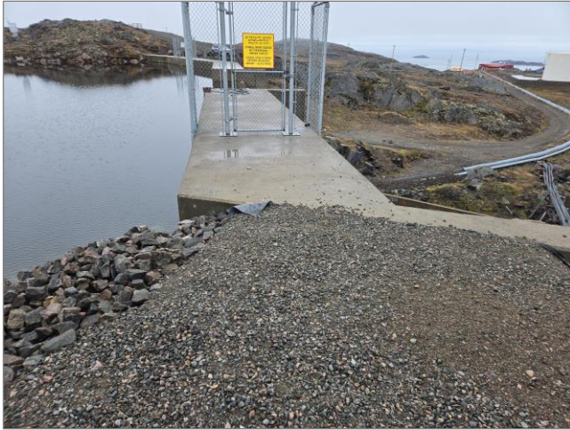
Figure 41 North Concrete Dam Abutment
