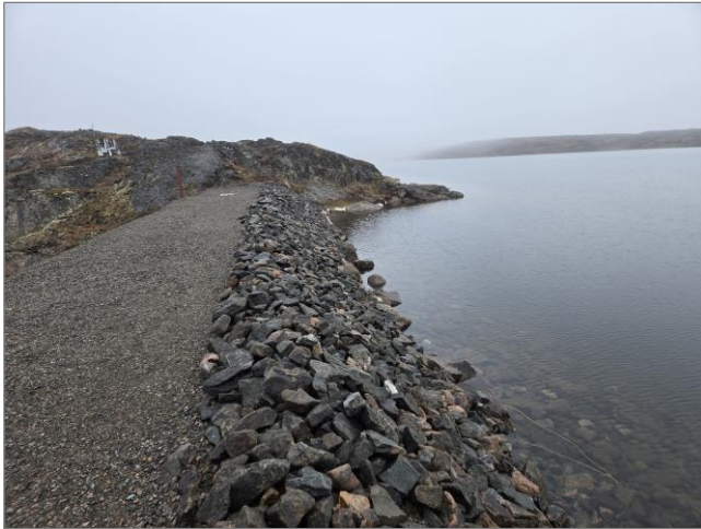
Figure 5 Upstream Riprap at North Berm Abutment
