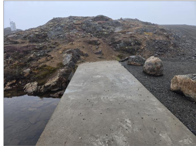
Figure 27 South Concrete Dam Tie-In to Bedrock
