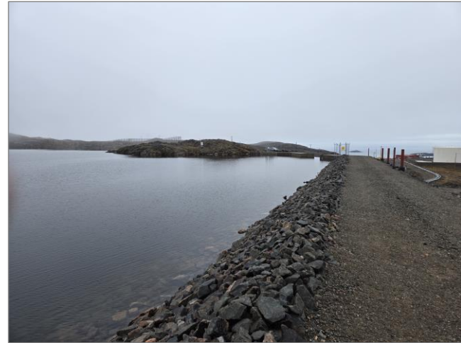
Figure 7 Upstream Limited Riprap Parapet
