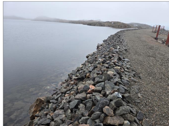
Figure 4 Upstream Riprap at North Berm
