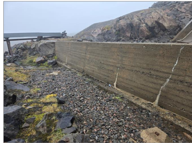
Figure 35 Discharge Channel Training Wall
