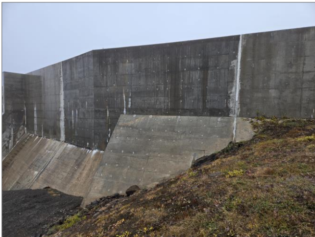
Figure 30 South Concrete Dam
