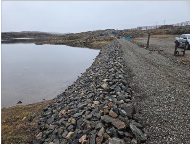
Figure 9 Upstream Rockfill – South Berm
