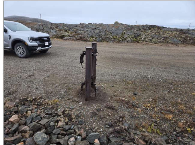
Figure 11 Utility Pole Anchor at Toe of South Berm
