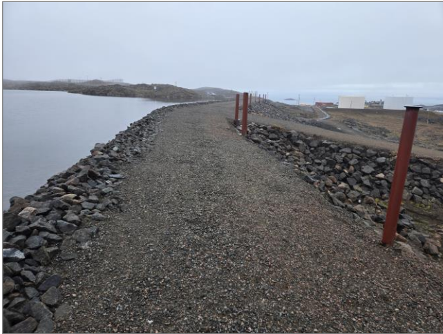
Figure 13 North Berm Crest BH101 and BH102
