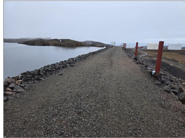
Figure 16 Central Berm Crest, BH 105, Rockfill Parapet
