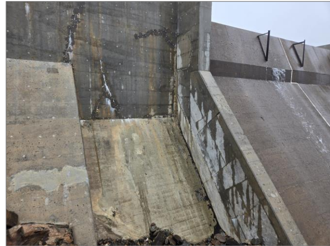
Figure 40 North Concrete Dam Training Wall
