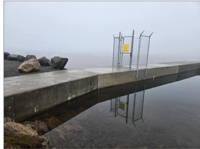
Figure 28 South Concrete Dam, Upstream Freeboard
