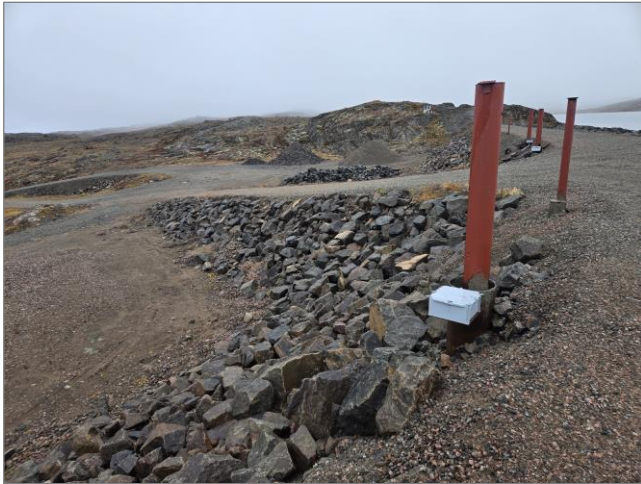
Figure 17 BH105 and Dam Access Road
