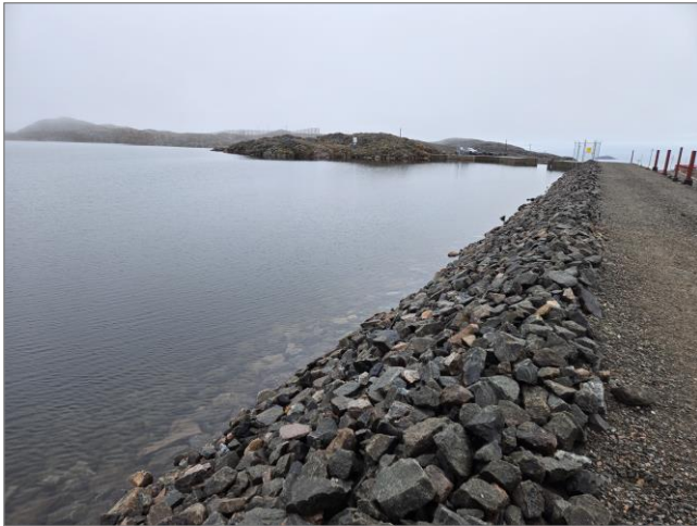
Figure 6 Upstream Riprap at Centre Berm
