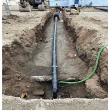
ATCO Loop Utilidor Upgrades Completed November 2023
