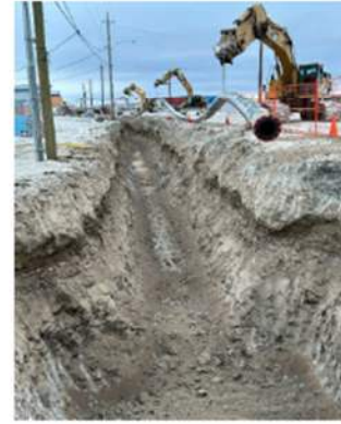
Federal Road Utilidor Upgrades November 2023
