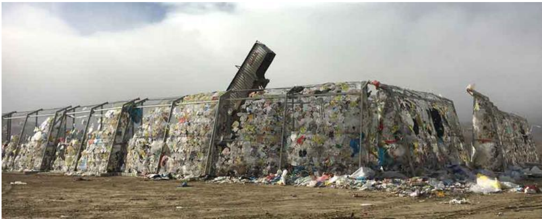
Litter screens deployed to encircle the tipping face. Portable screens would require re-positioning as wind directions changes. Photograph shows effective deployment of portable screens. Photograph courtesy Metta Technologies
