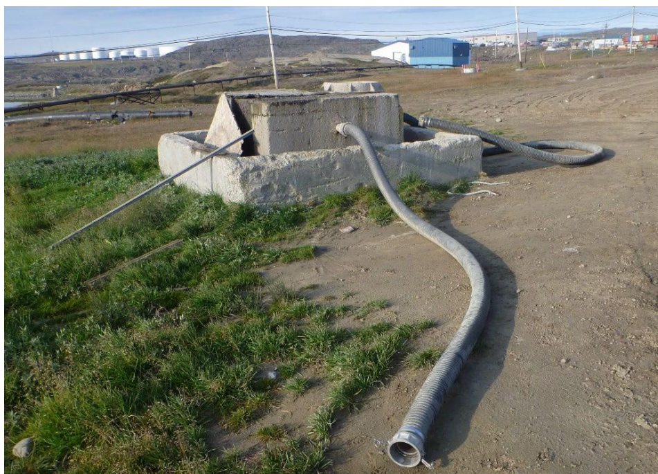
Figure 1 Truck Dump Station
