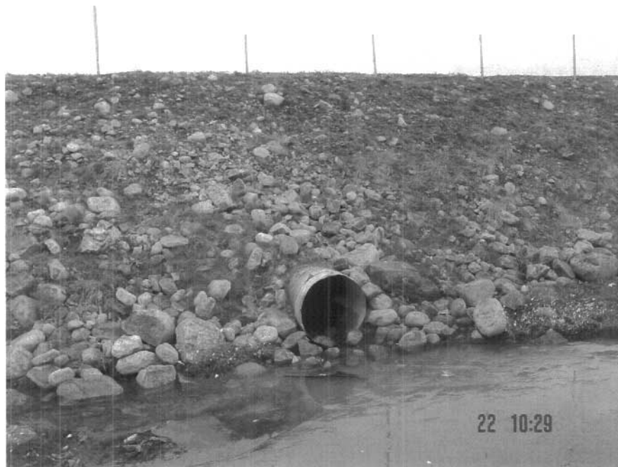
Figure 6. Plugged discharge culvert at the South end of the City of Iqaluit landfill.
