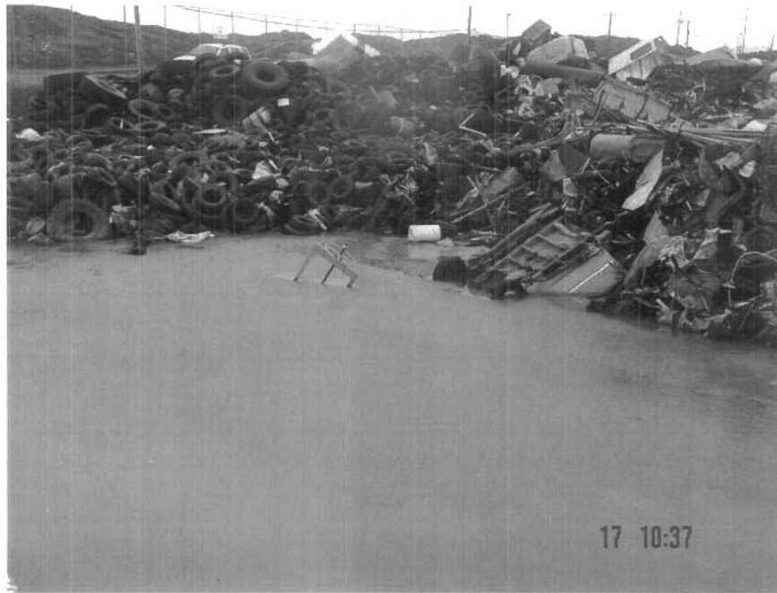
Figure 5. Collection of water at South end of Iqaluit landfill with unsegregated waste visible.
