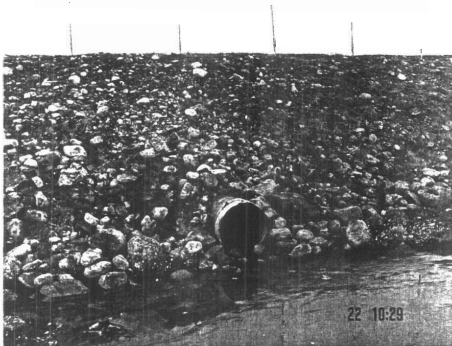
Figure 6. Plugged discharge culvert at the South end of the City of Iqaluit landfill.
