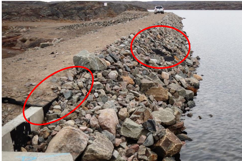
Figure 3-15: Evidence of wave action acting on Central Berm upstream armor.
