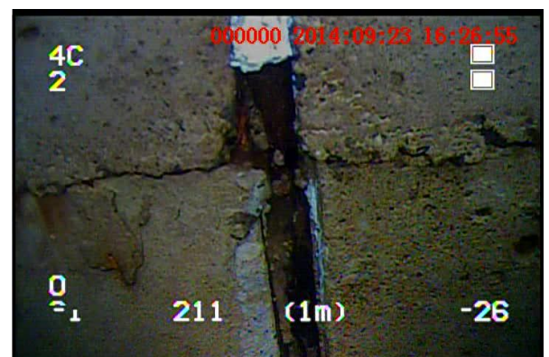
J4 showing gap in joint starting just below white caulking
