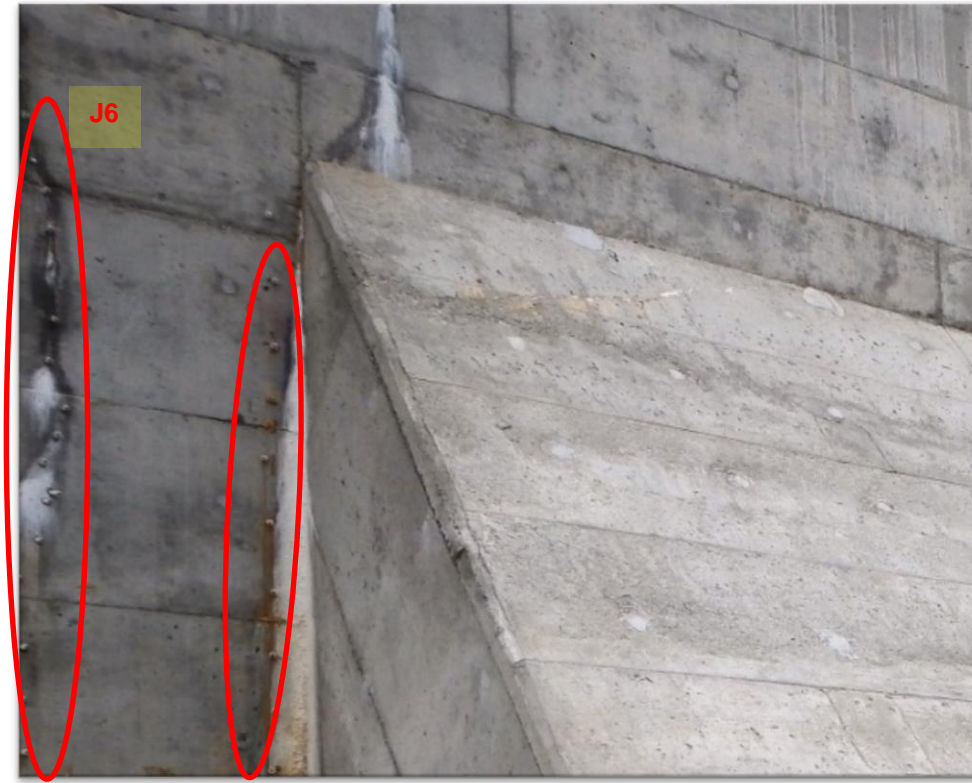
Figure 3-26: Efflorescence and staining at J6, left abutment. Injection ports from seepage repair shown.
