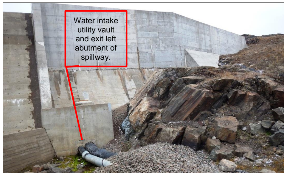
Figure 1-3: Photograph of the left abutment downstream dam face.
