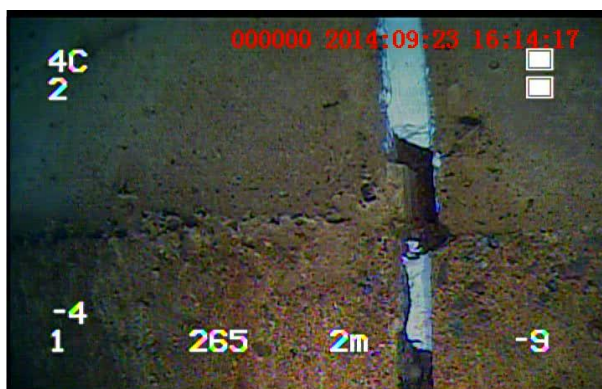
Joint J2 start of gap, and missing material
