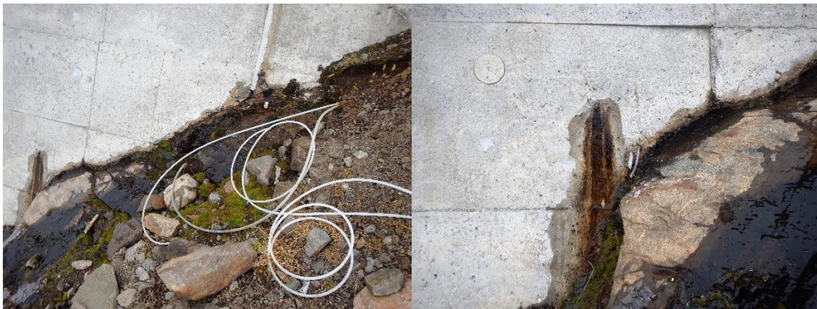
Figure 3-28: Pressure relief tubing at left abutment buttress.
