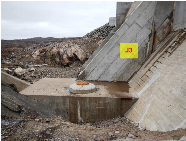
Figure 3-23: Seepage and staining at J3 and along 2006 construction lift contact.
