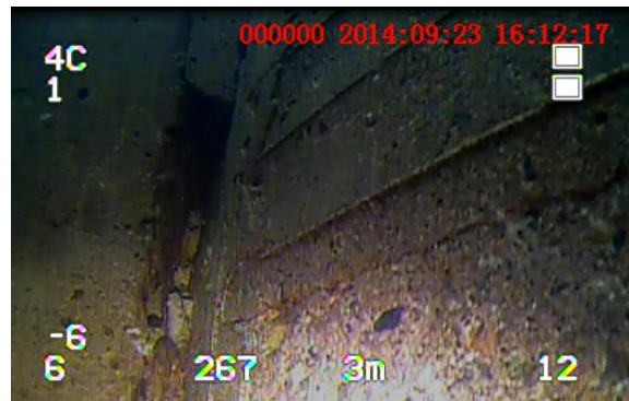
Figure 3-9: Spalling in 1995 concrete joint J1.
