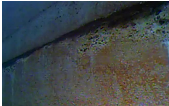
Figure 3-14: Spalling ~2 m east of J4, 2 m below crest.
