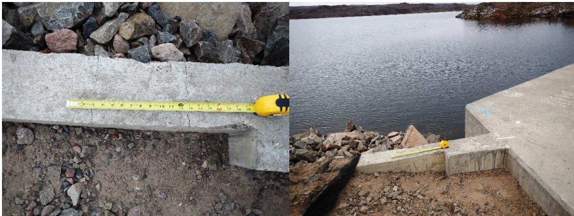
Figure 3-27: Shrinkage cracks on wingwall right abutment Station 1+35.
