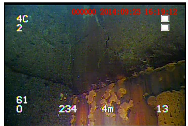
J3 continuing down showing crack until it reaches top of old structure.
