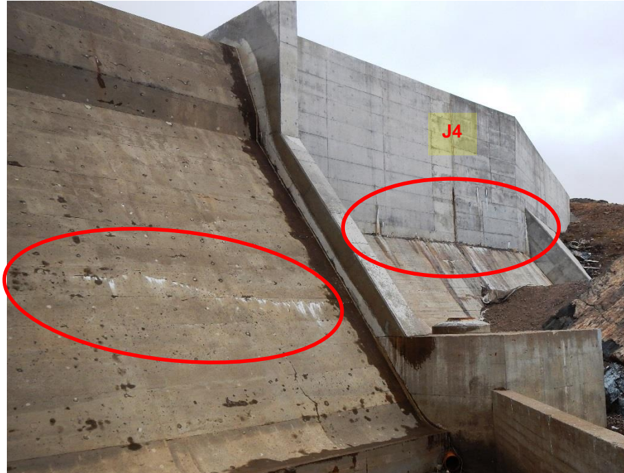
Figure 3-24: Downstream dam face showing efflorescence associated with seepage through spillway crack. Seepage and staining also noted at 2006 concrete lift contact.
