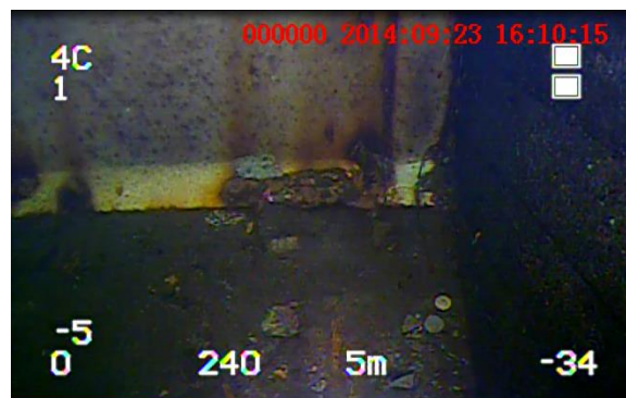
Figure 3-8: Corrosion of steel plate along spillway at El 106.7 m, corner junction at J1 (refer to Section A-A dwg S2, 2006).
