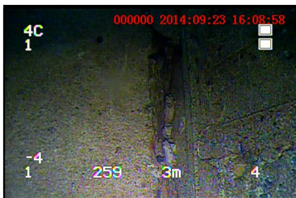
Joint J1 spalling in concrete
