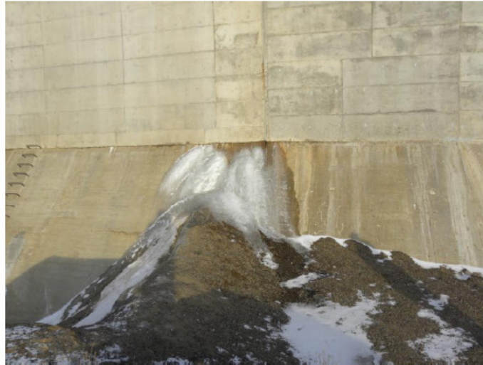
Photograph 5 New leak South of spillway section.
