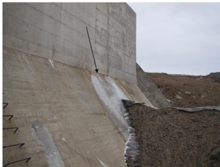
Photograph 8 Leakage at South Gravity section; Similar to 2009 DSL.
