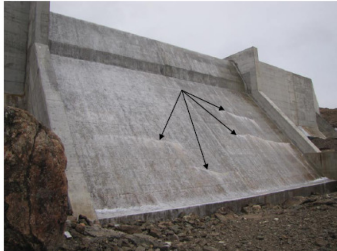
Photograph 7 Leaching cracks in Spillway face; Similar to 2009 DSL.
