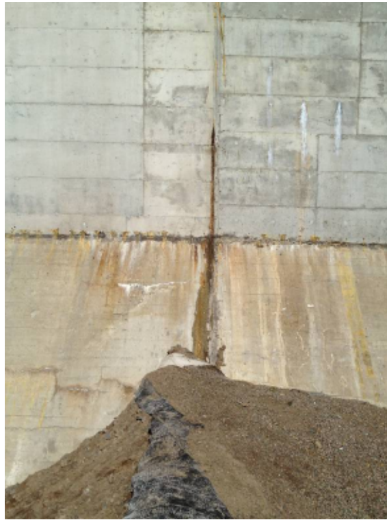
Photograph 8 South structure control joint showing minor leak at previous injection repair.
