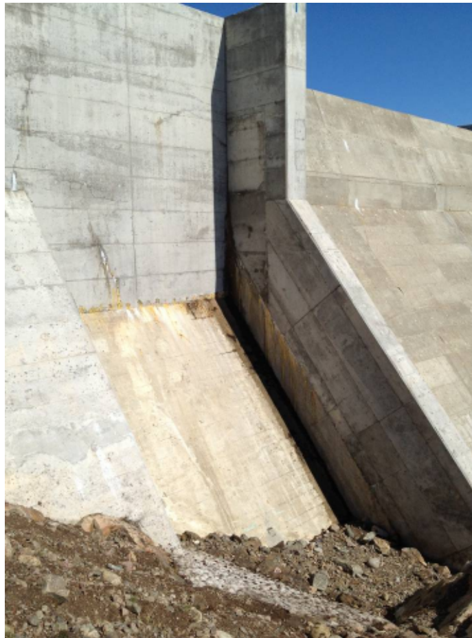
Photograph 5 Minor leakage at north transition of spillway at previous injection repair.
