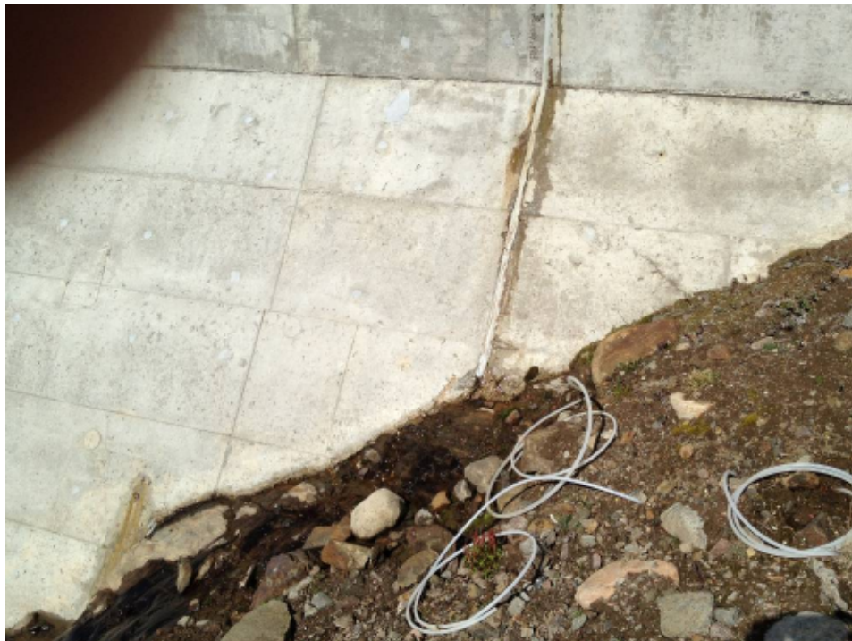
Photograph 9 Minor leak at another control joint on south structure.
