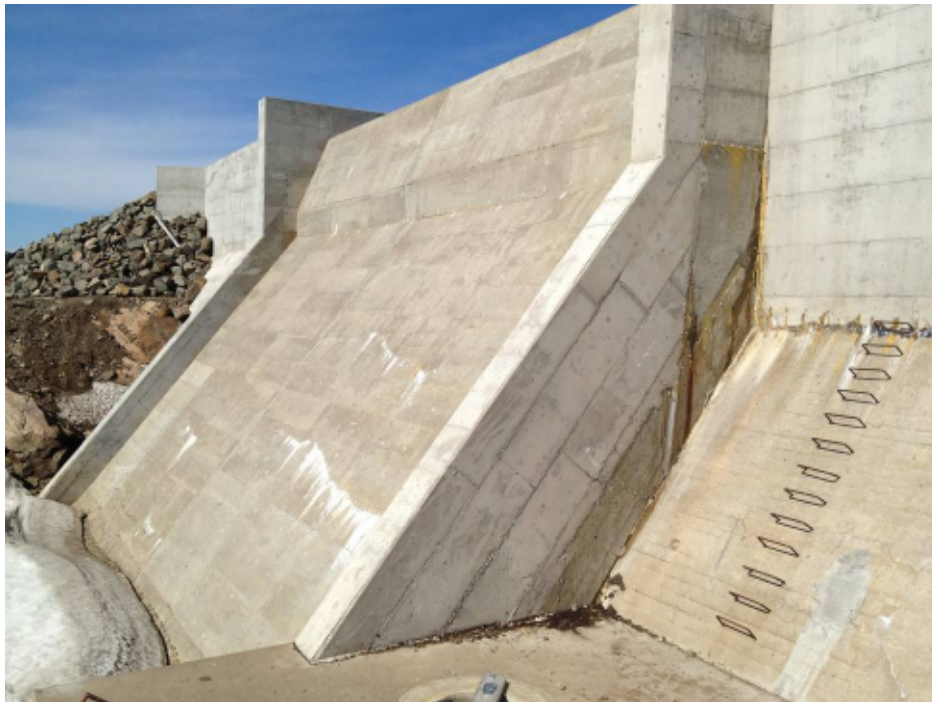
Photograph 6 Overview of spillway from the southwest. Note minor leakage at previous injection repair.
