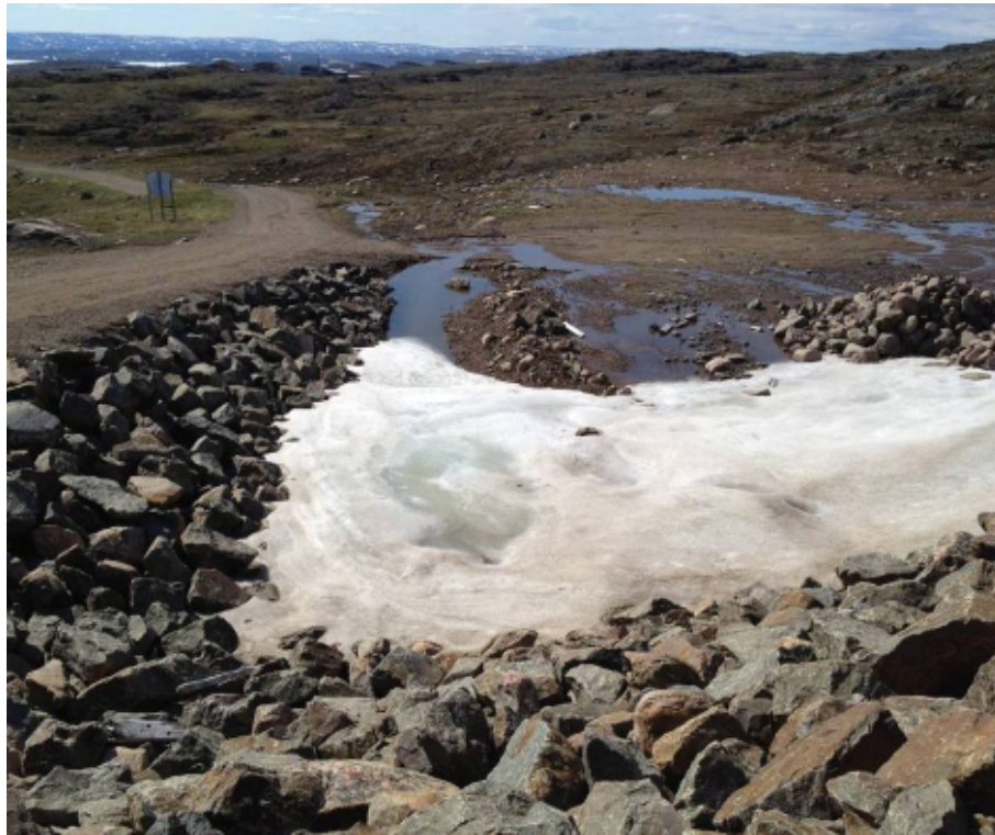
Photograph 3 Meltwater and potential minor leakage at north side of access road / north berm.
