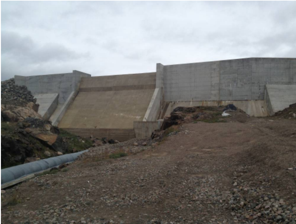
Photo 1: Overview of Dam Spillway and Wingwalls.
