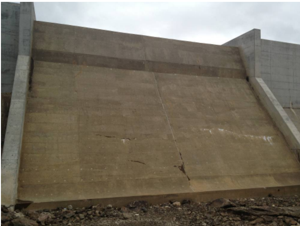
Photo 2: Spillway – Note minimal leakage.
