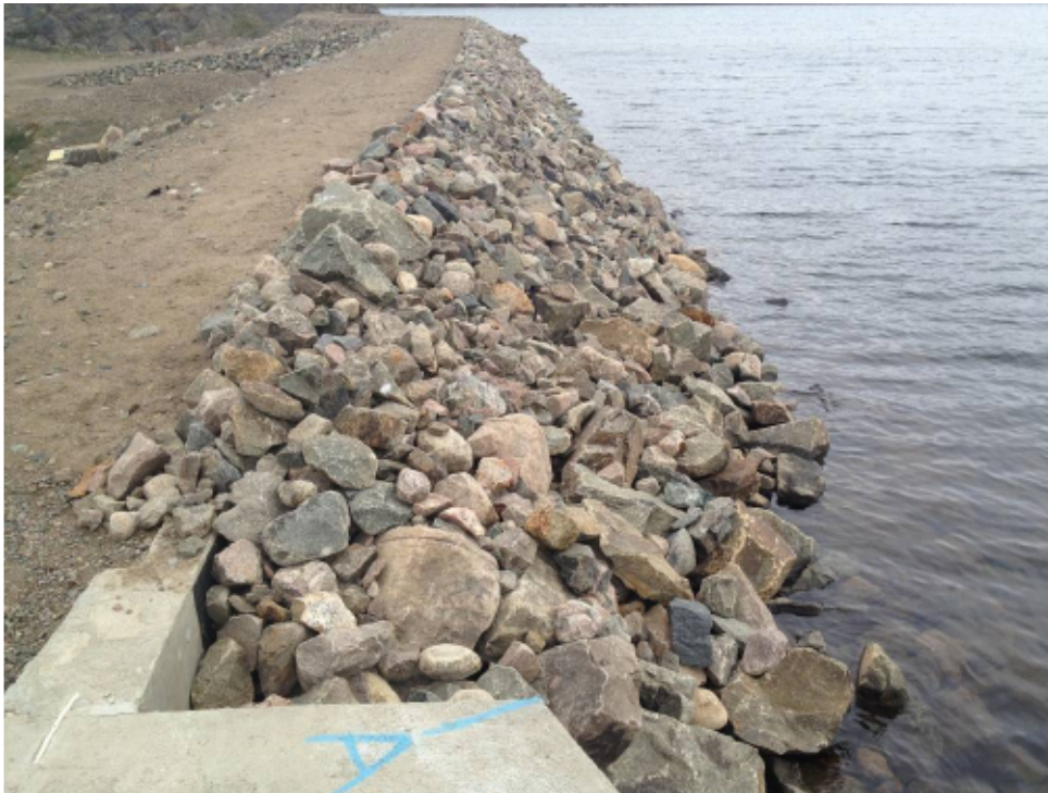
Photo 7: North Berm at Wingwall – Supplementary ballast and riprap required.
