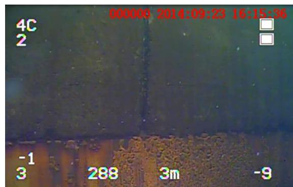
Figure 3-11: Joint filler missing from J2, photograph of contact with steel plate El 106.7 m.
