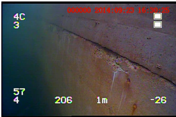
Spalling in concrete, horizontal joint between J4 & J5
