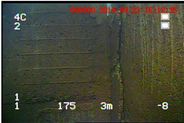
J3 just below caulking, crack in concrete extending down and out.
