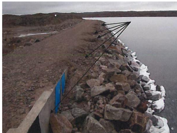
Figure 2-1: Photograph of wave erosion on upstream side of Central Berm in 2010.
