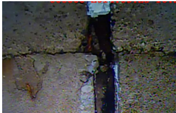
Figure 3-13: Spalling and absence of joint filler J4 on South Dam (left abutment).
