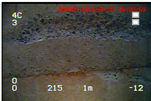
Spalling in horizontal Joint between J3 & J4
