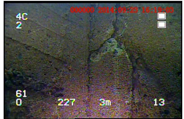
J3 just below caulking, crack in concrete extending down and out.
