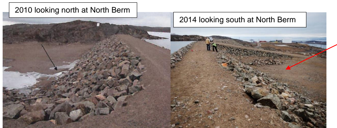
Figure 3-16: Photograph of seepage in 2010 on the downstream face of the North Berm. Seepage was not evident at this location in 2014 (right photograph).
