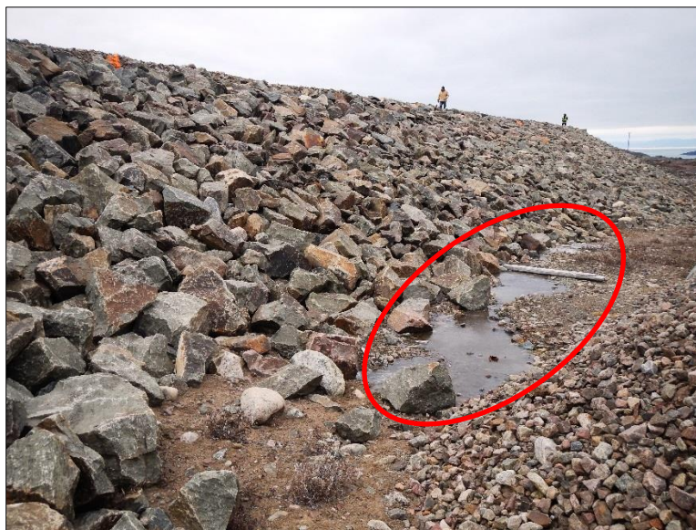
Figure 3-17: Photograph of ponding due to seepage at Station 0+70.
