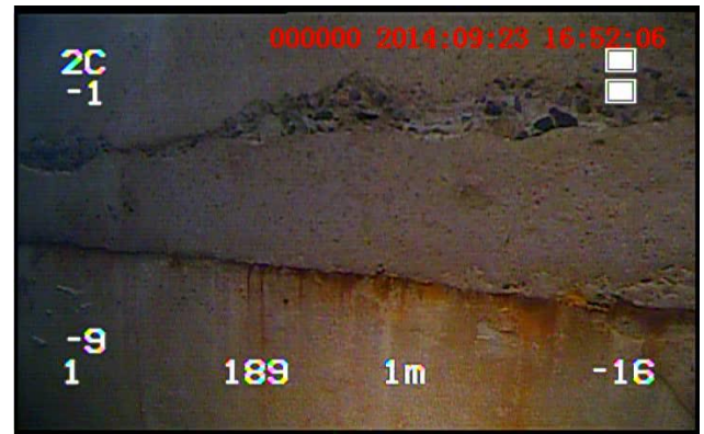
Spalling in concrete, horizontal joint between J4 & J5
