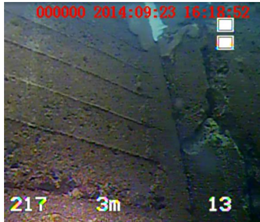
Figure 3-12: Spalling at J3 on the eastern edge of the spillway, from 2-m depth to underlying contact with steel plate.
