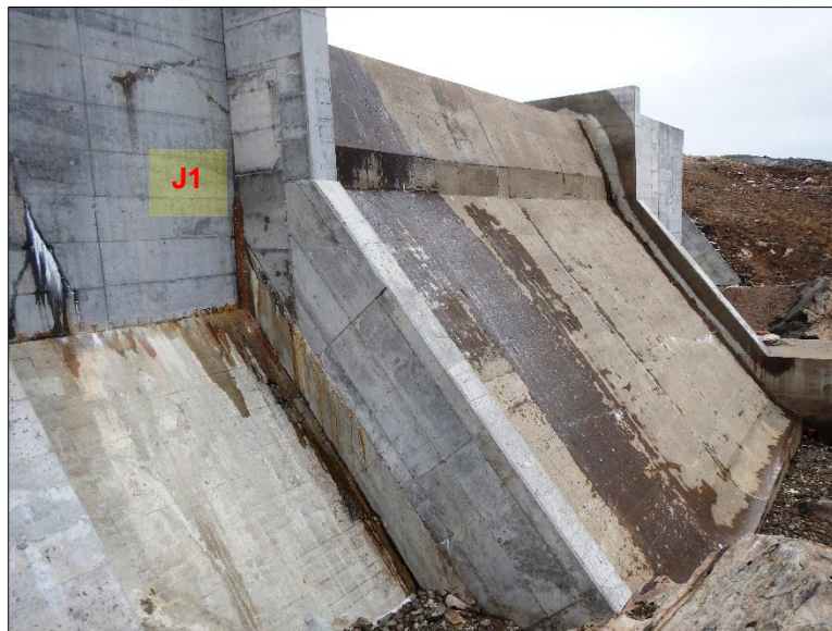
Figure 3-21: Seepage and staining at J1 and along 2006 construction lift contact.
