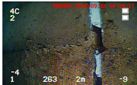
Figure 3-10: Joint filler termination at 2 m below crest on J2.
