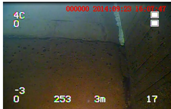
Figure 3-6: Joint filler of J1 terminates at 2 m below the crest at the 1995 and 2006 construction contact. ROV camera directed upward.
