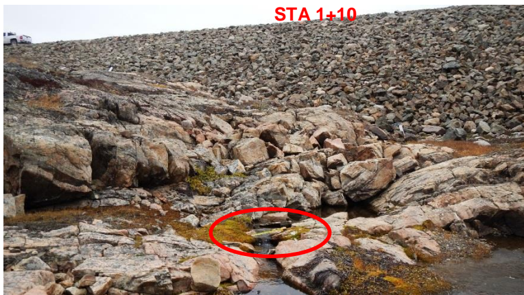
Figure 3-19: Photograph of seepage measure location circled red below Station 1+10.
