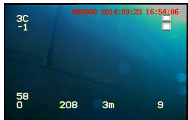
Bottom of J5, meeting Horizontal joint with old structure.
