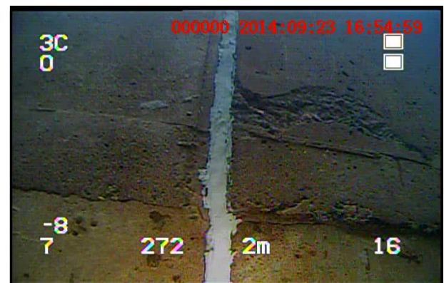
Spalling in concrete along vertical joint J5
