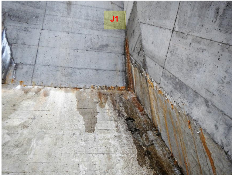
Figure 3-22: Close-up photograph of seepage and staining at J1.
