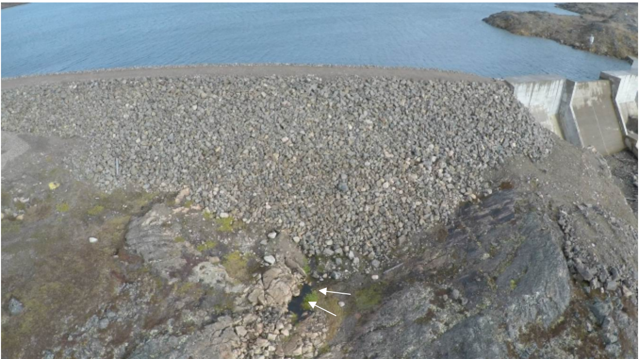
Photo 4: West elevation of the center berm, note the seepage at the base of the berm.
