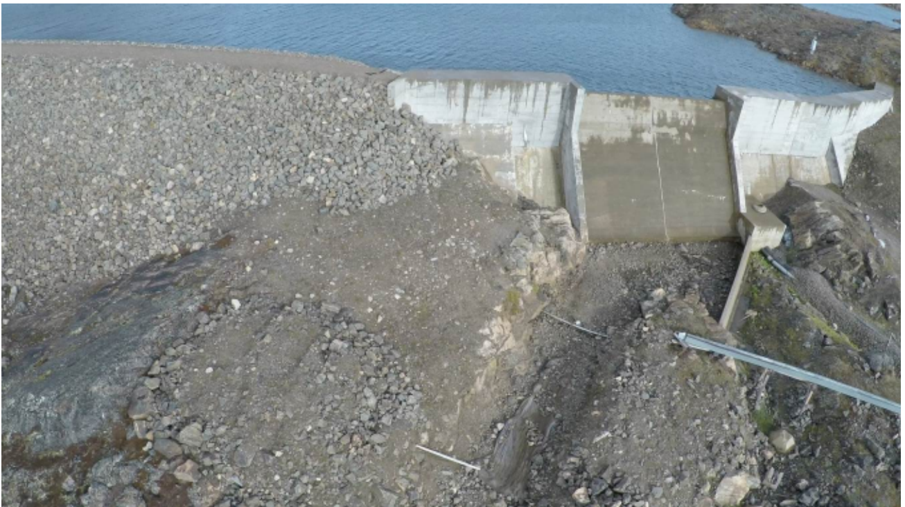
Photo 6: West elevation of the center berm and dam, note the exposed geotextile membrane within the spillway channel.
