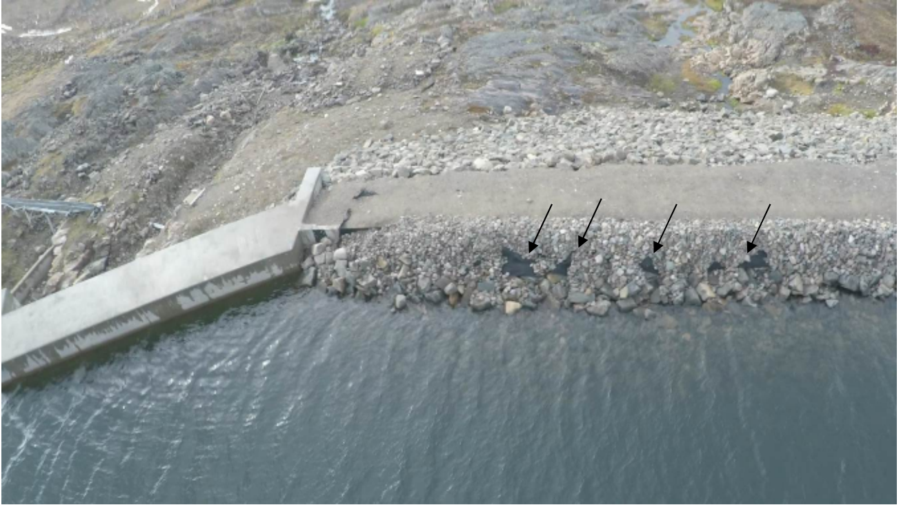
Photo 5: East elevation of the center berm, note the exposed geotextile membrane.
