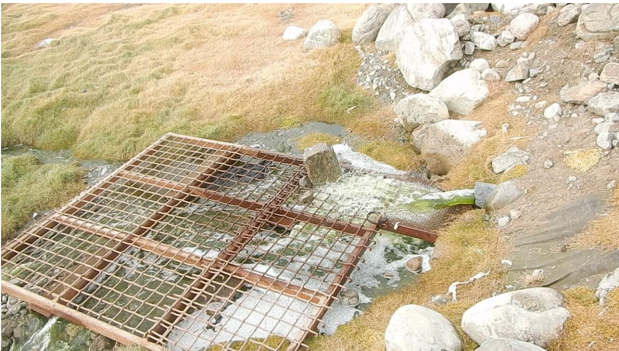
Photo 2: Active decanting of the sewage lagoon, west berm.
