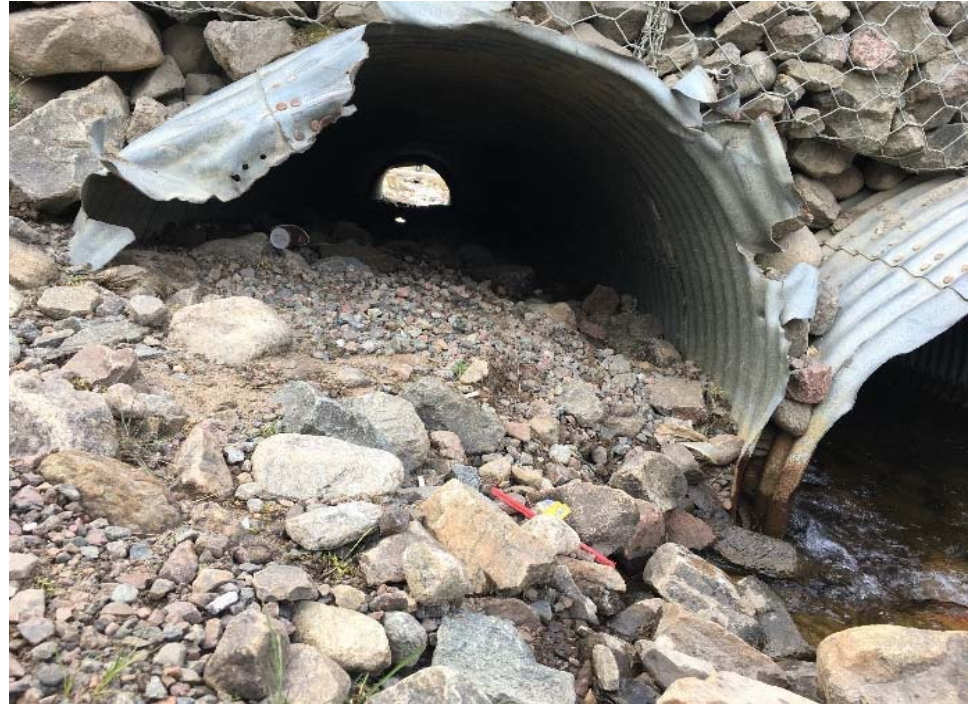
Upstream of Crossing 2 (3 x 1200 mm dia.) - Broken End
