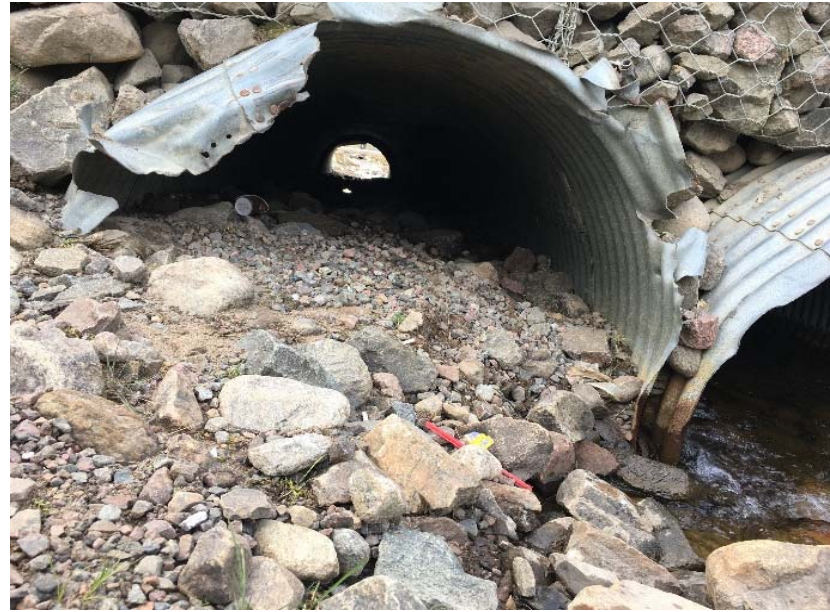
Upstream of Crossing 2 (3 x 1200 mm dia.) - Broken End
