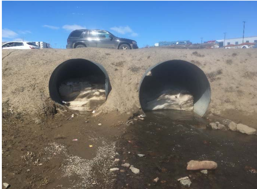
South of Crossing 8 (2 x 1950 mm dia.) looking North - Blocked due to snow
