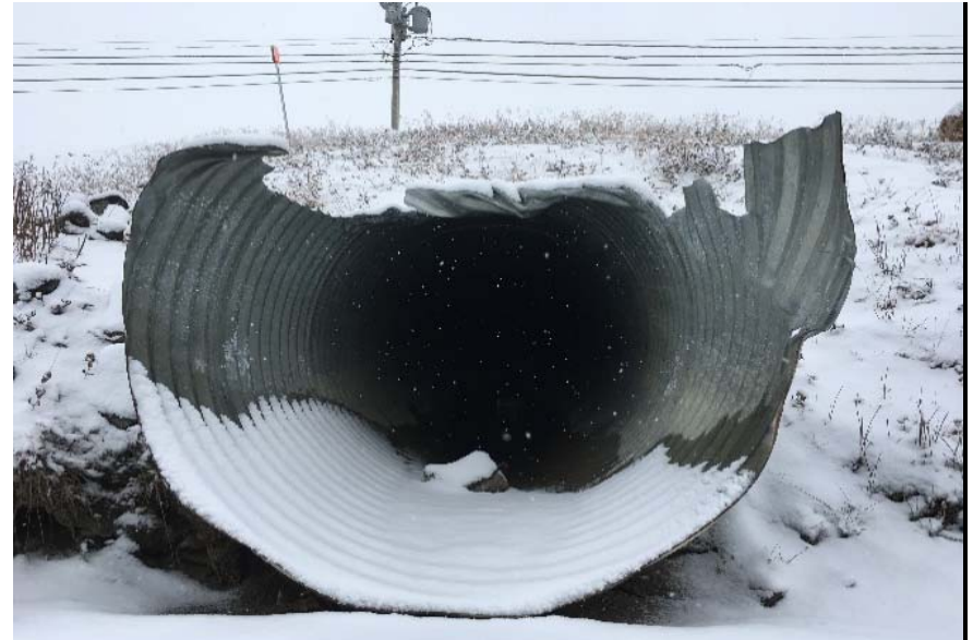
North of Crossing 3 - Broken End
