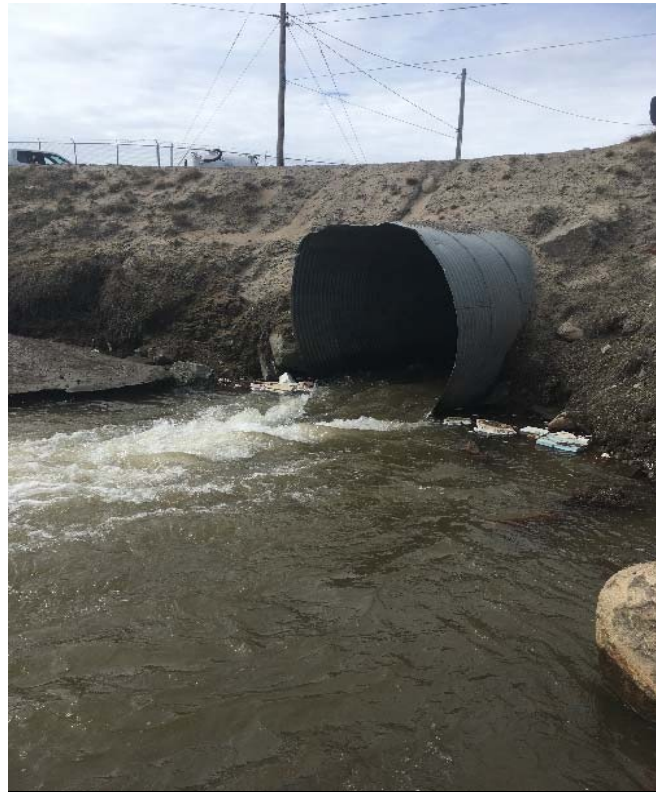
South of Crossing 2 (2100 mm dia.) - Accumulated Garbage
