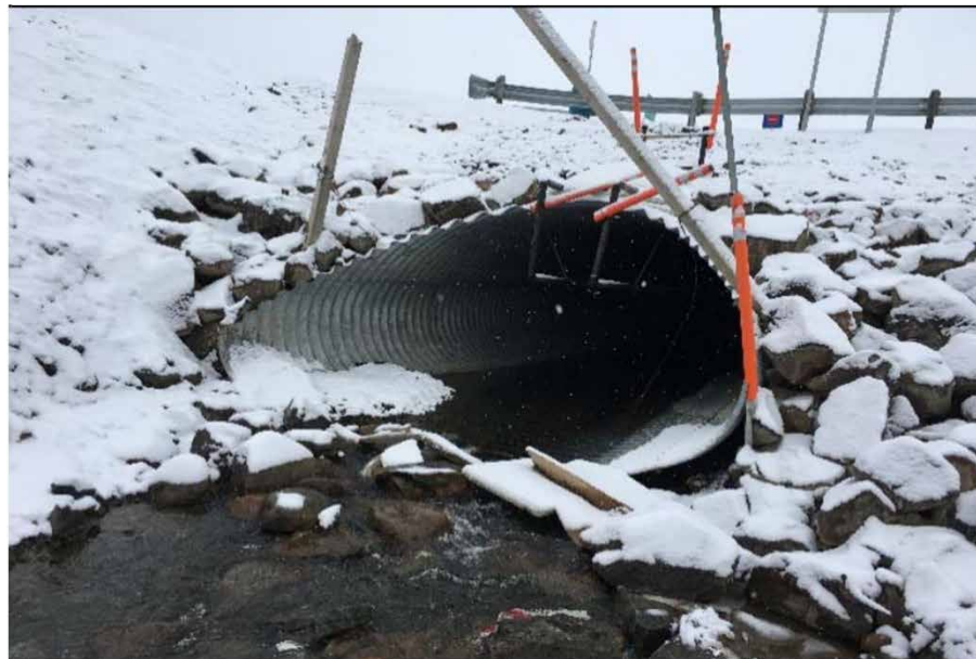
East of Crossing 10 (3100 mm dia.) -Deflected Pipe
