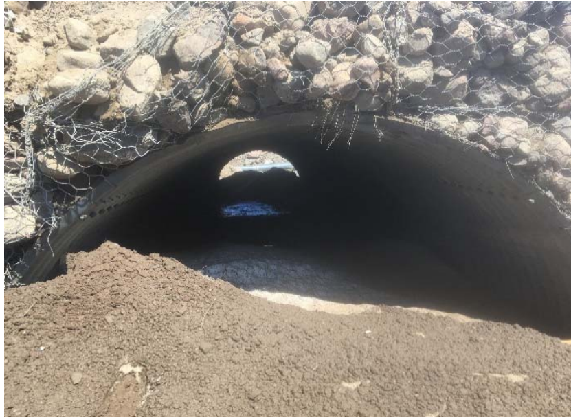
South of Crossing 7 (3200 mm dia.) looking North - Sediment Buildup
