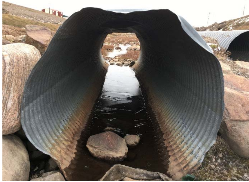
Upstream of Crossing 6 (1300 mm dia.) - Deflected Pipe
