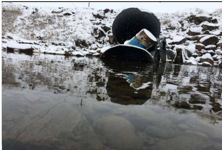
East of Crossing 13 (1600 mm dia.) looking Downstream -Barrel inside the pipe, probably received during the stream flow
