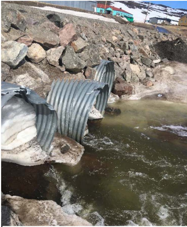
Cluster 2 of 3 Culverts (3 x 1100 mm dia.) on south side of road - Blocked due to snow
