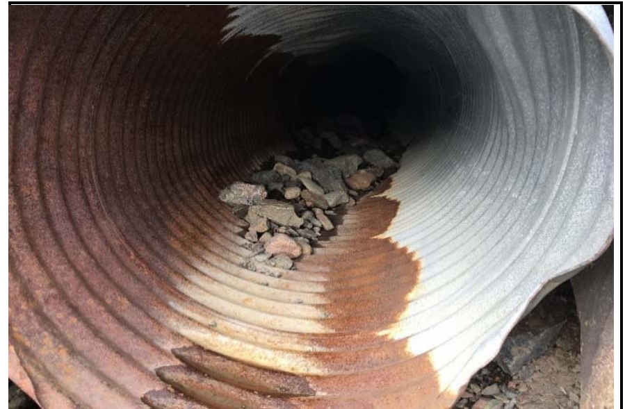
Southside of Cluster 3 - Debris due to sedimentation in the culvert
