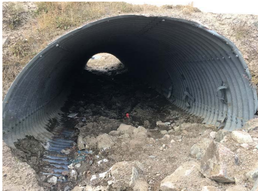
Upstream of Crossing 7 (3200 mm dia.) - Sediment Buildup inside the pipe
