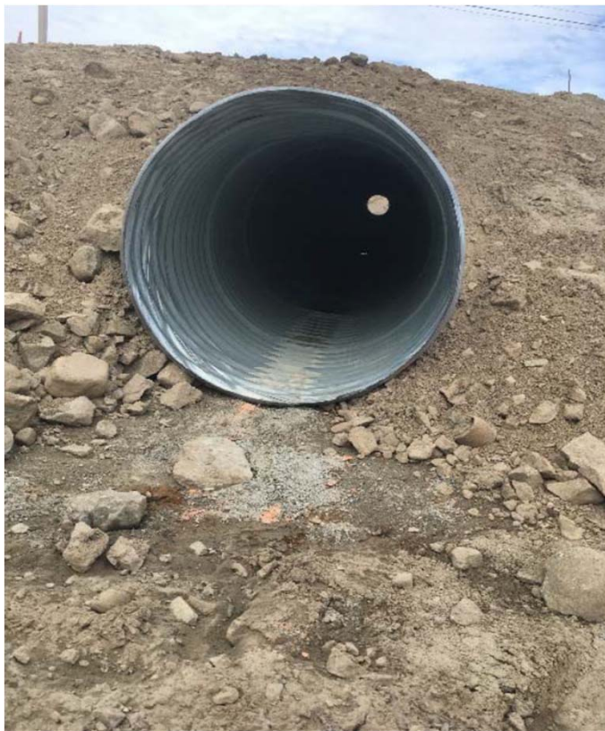
South of Crossing 4 (800 mm dia.) -not receiving any flow
