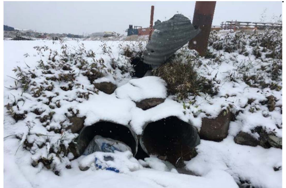
North of Crossing 5 (3 x 300 mm dia.) looking Upstream -Garbage in the pipe
