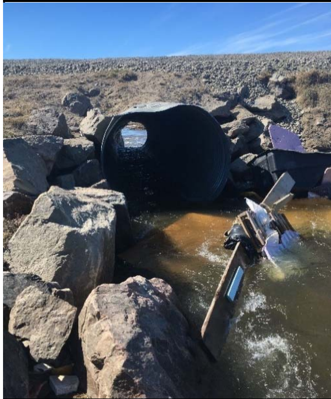
North of Crossing 12 (3 x 1000 mm dia. and 1 x 2100 mm dia.) - Garbage in the stream
