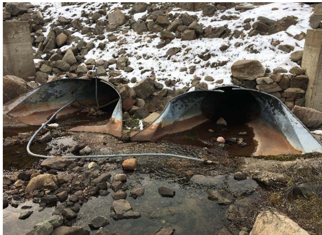
Upstream of Crossing 10 -2 x 1350 mm dia., 80m long, steep installation
