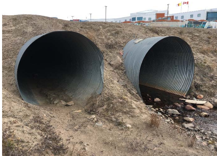
Downstream of Crossing 8 (2 x 1950 mm dia.)
