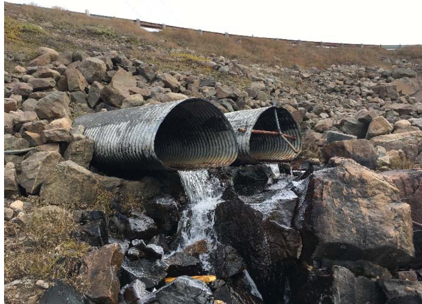
Downstream of Crossing 10 (2 x 1350 mm dia.)
