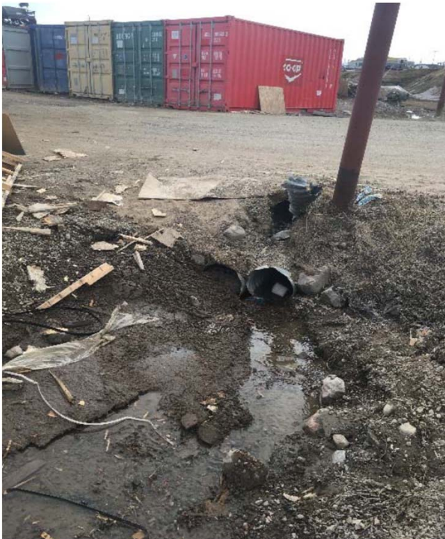
North of Crossing 5 (3 x 300 mm dia.) - Garbage accumulated
