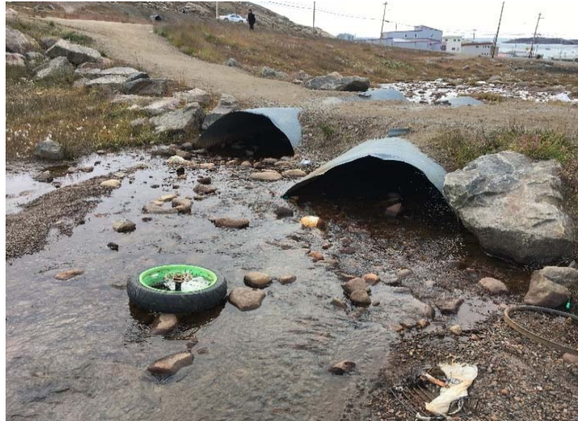
Upstream of Crossing 4 (2 x 1350 mm dia.) - Tire seen in the stream, pipes half buried in the substrate
