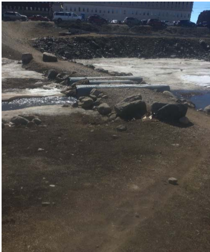
Crossing 6 looking South West - 2 x 1300 mm dia., 7 m long with one 800 mm dia. dia overflow pipe
