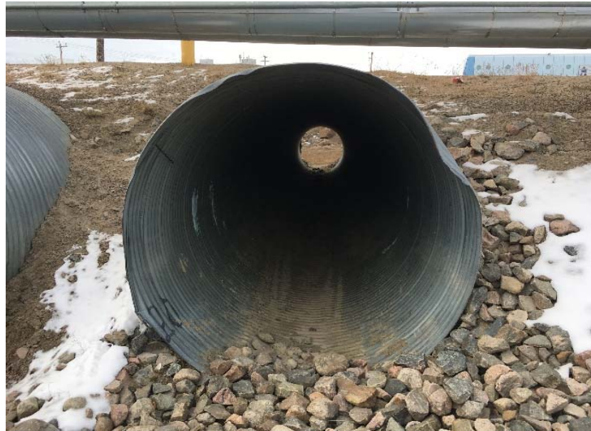
Upstream of Crossing 8 (1950 mm dia.) - Sediment buildup in front of pipe
