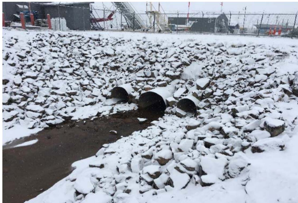
East of Crossing 8 (2 x 1000 mm dia. and 1 x 1600 mm dia.)
