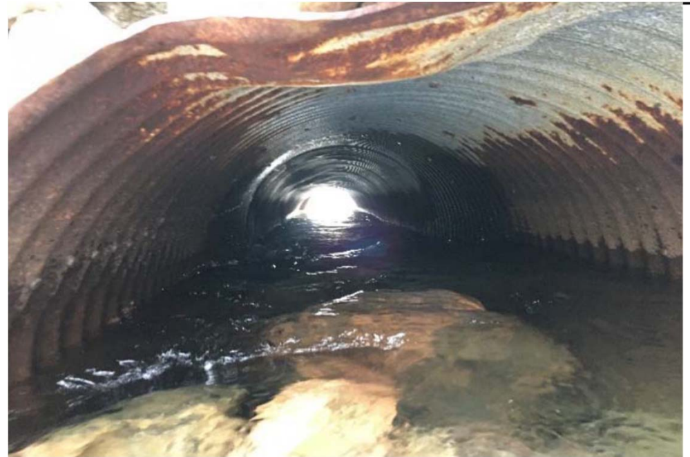
Cluster 2 of 3 Culverts (3 x 1100 mm dia.) on south side of road - Blocked due to snow
