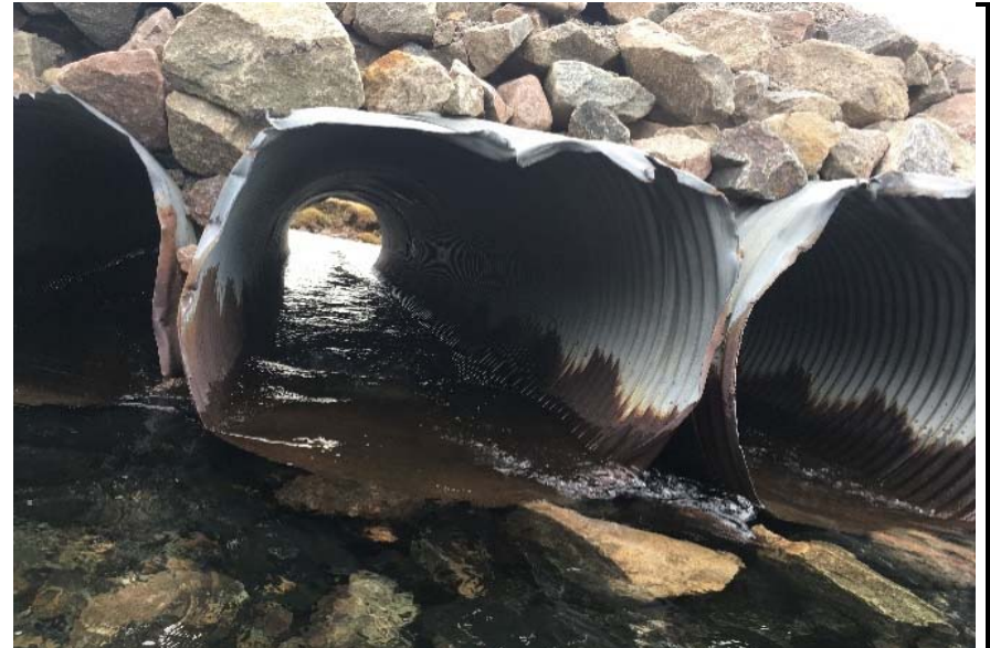
Cluster 2 (3 x 1100 mm dia.) taken from South side of road - Damaged Ends
