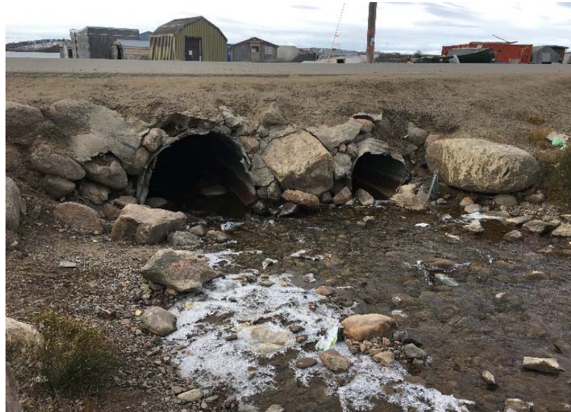
Upstream of Crossing 1 ( 2 x 700 mm dia.) - Damaged Ends
