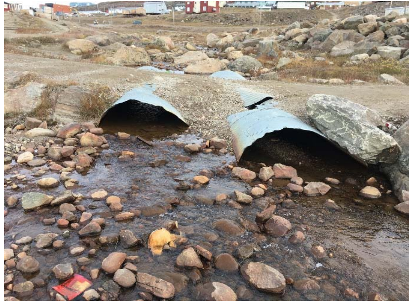
Downstream of Crossing 4 (2 x 1350 mm dia.) - Garbage in the stream
