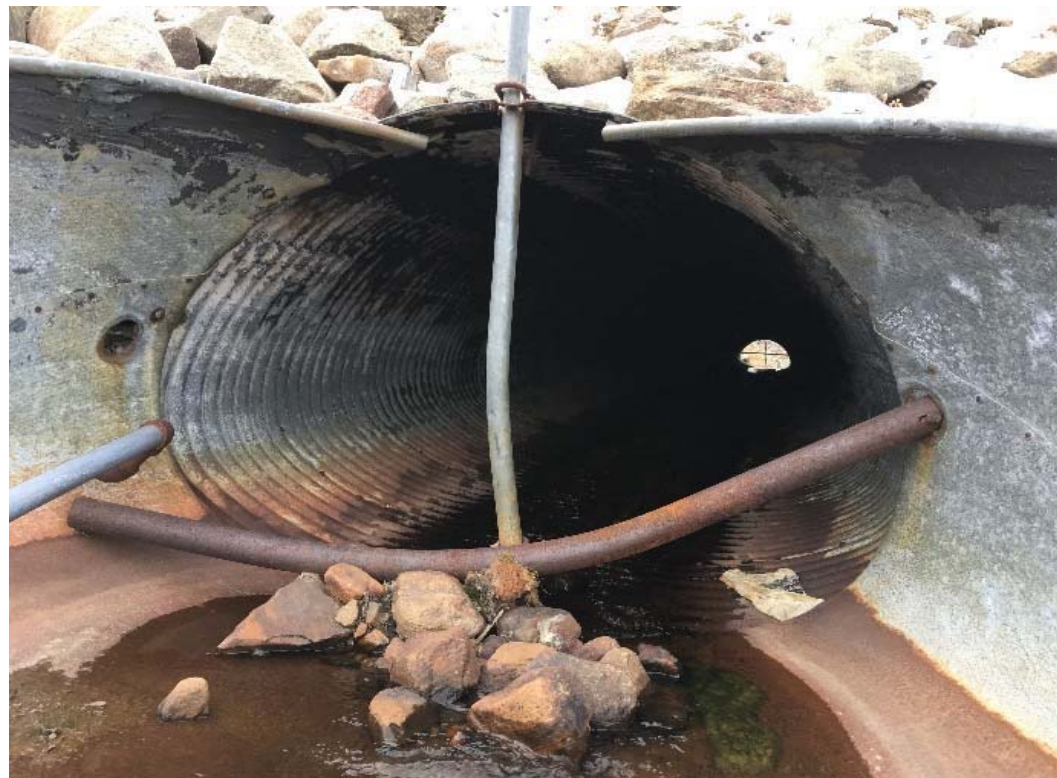
Upstream of Crossing 10 (1350 mm dia.) -Bars in the pipe
