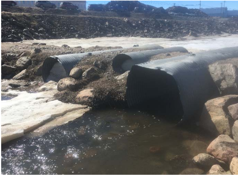
Crossing 6 ( 2 x 1300 mm dia. and 1 x 800 mm dia. overflow) looking South West - Blocked due to snow
