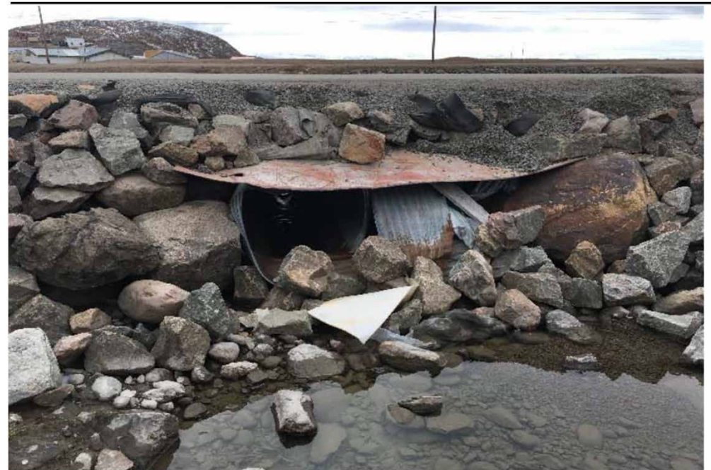
Cluster 1 of 4 Culverts (4 x 9400 mm dia.) on north side of road - Garbage and broken pieces in front of pipe
