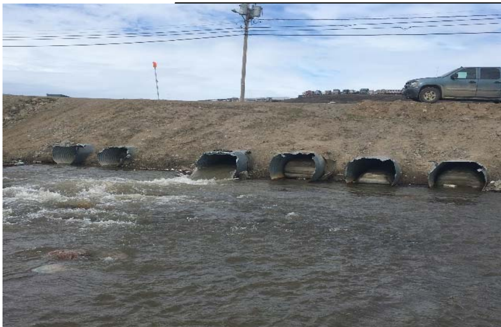
South of Crossing 3 (4 x 1200 mm dia. and 2 x 1000 mm dia.) - Damaged Ends
