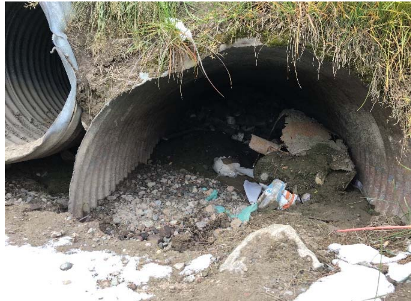
Upstream of Crossing 3 (1500 mm dia.) - Garbage and sediment buildup inside the pipe
