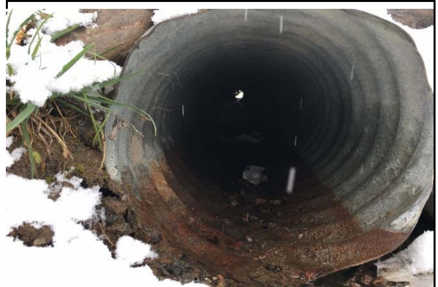
North of Crossing 5 (300 mm dia. ) looking Upstream - Corroded pipe exposed after the removal of garbage
