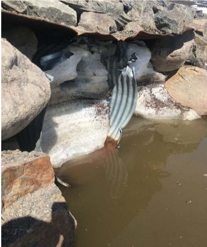
Eastern most culvert on south side of road - Blocked Pipe
