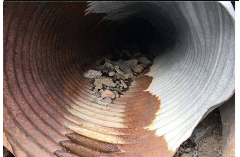
Southside of Cluster 3 - Debris due to sedimentation in the culvert
