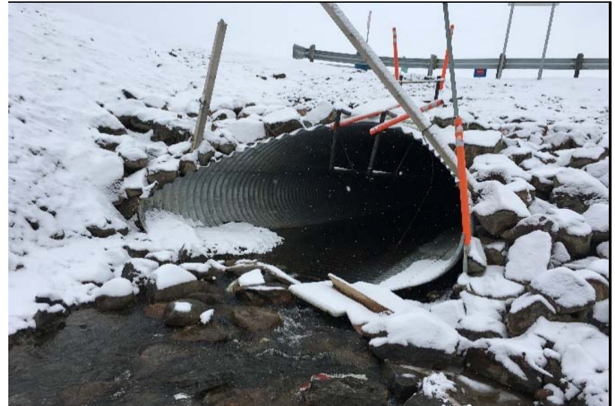
East of Crossing 10 (3100 mm dia.) - Deflected Pipe
