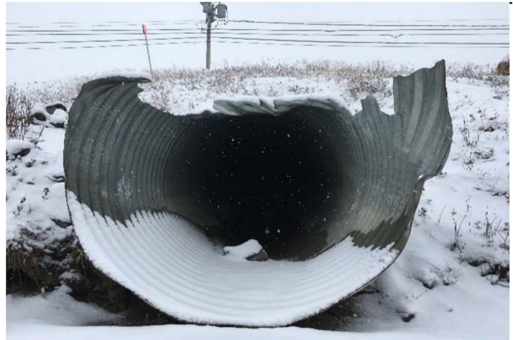
North of Crossing 3 - Broken End
