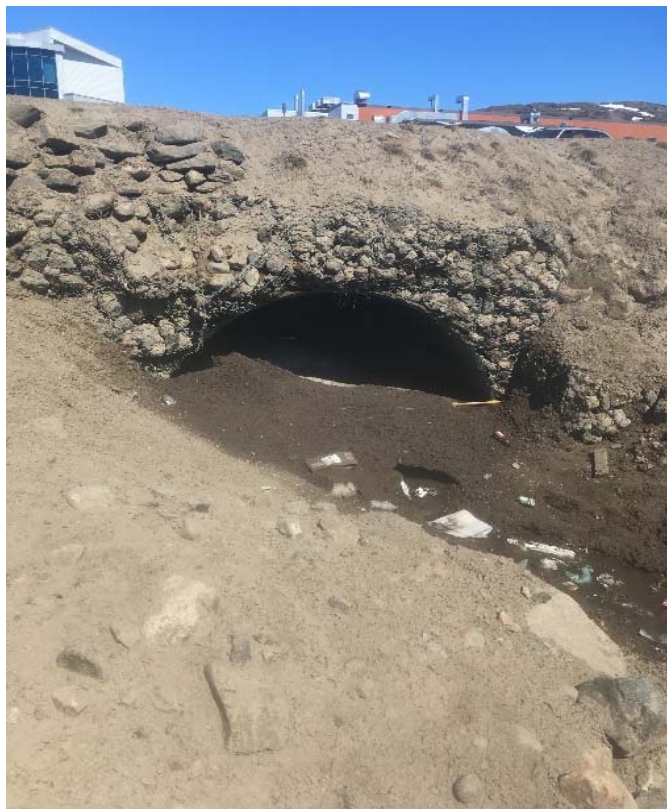
South of Crossing 7 (3200 mm dia.) looking North -Pipe not accessible due to sediment buildup
