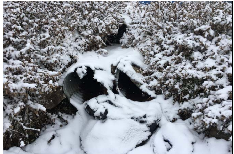
South of Crossing 5 (3 x 300 mm dia. ) looking Downstream - Garbage accumulated
