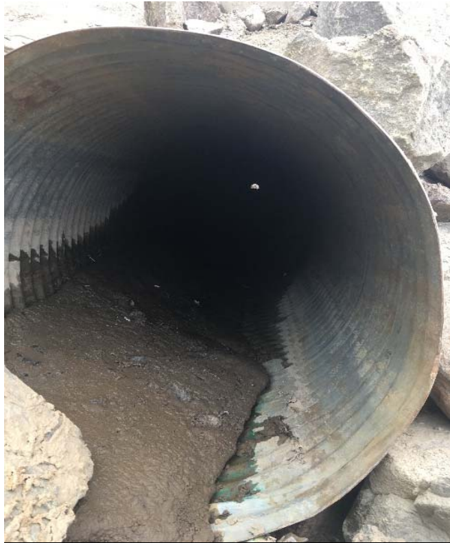
East of Crossing 8 (1600 mm dia.) closeup - Sediment buildup inside the pipe
