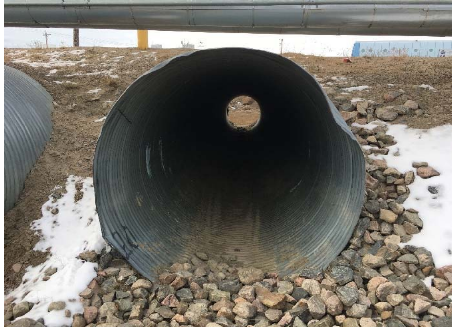
Upstream of Crossing 8 (1950 mm dia.) -Sediment buildup in front of pipe
