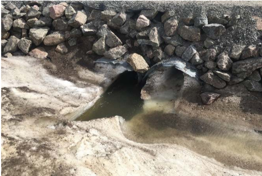
Cluster 1 (4 x 9400 mm dia.) taken from north side of road - Blocked due to snow
