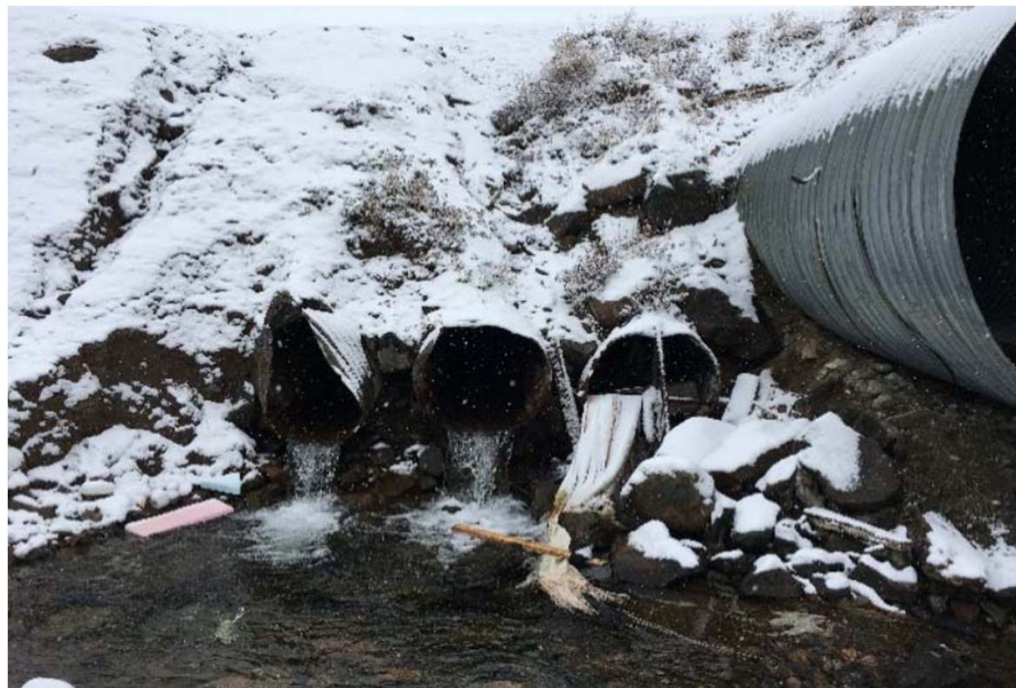
South of Crossing 12 (3 x 1000 mm dia. and 1 x 2100 mm dia.)
