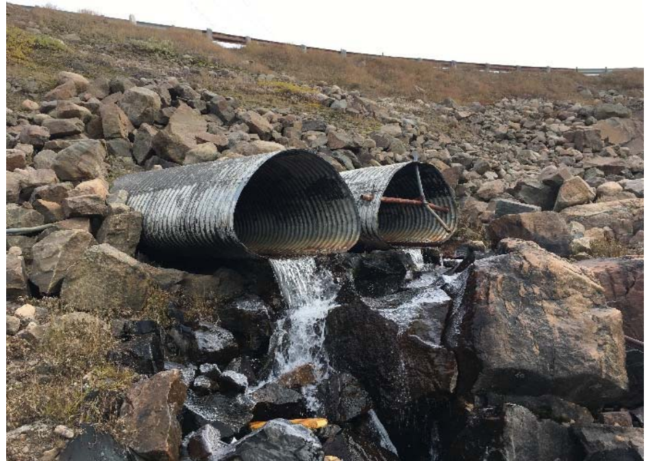
Downstream of Crossing 10 (2 x 1350 mm dia.)
