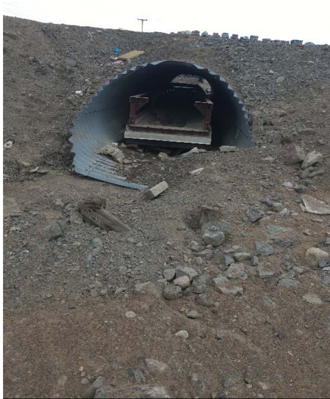
West of Crossing 9 (2100 mm dia.) - Furniture inside the pipe
