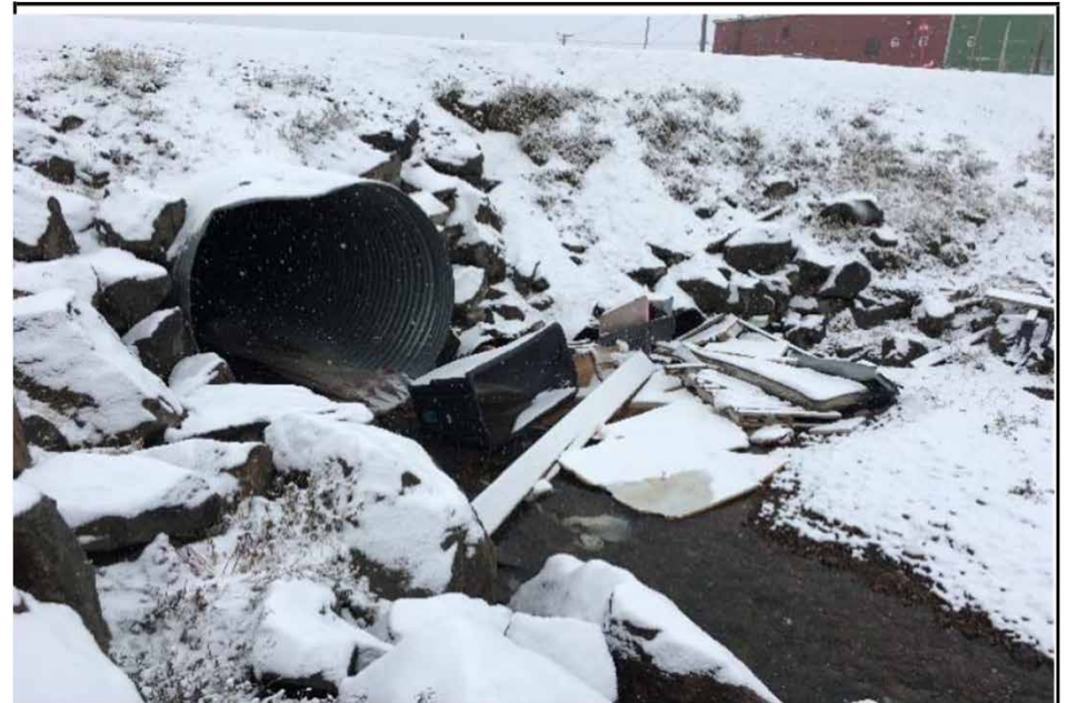
North of Crossing 12 (3 x 1000 mm dia. and 1 x 2100 mm dia.) looking Upstream -Garbage buildup infront of pipe
