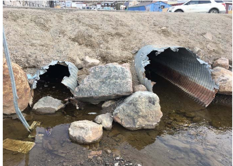
Downstream of Crossing 1 ( 2 x 700 mm dia.) - Damaged and broken pieces
