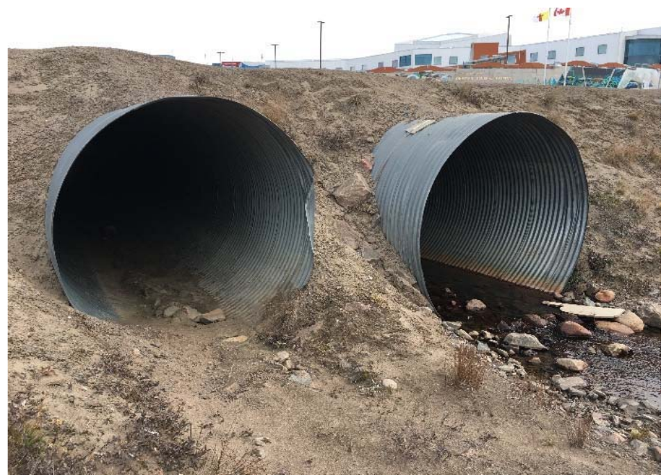
Downstream of Crossing 8 (2 x 1950 mm dia.)
