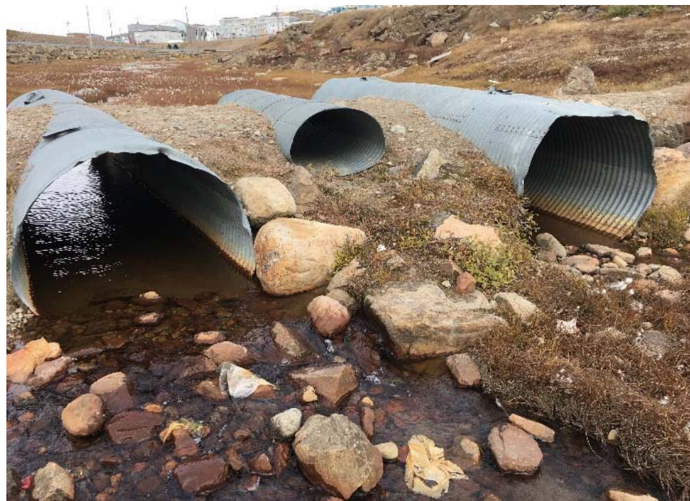
Downstream of Crossing 6 -2 x 1300 mm dia., 7 m long with one 800 mm dia. dia overflow pipe
