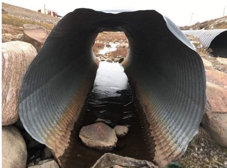
Upstream of Crossing 6 (1300 mm dia.) -Deflected Pipe
