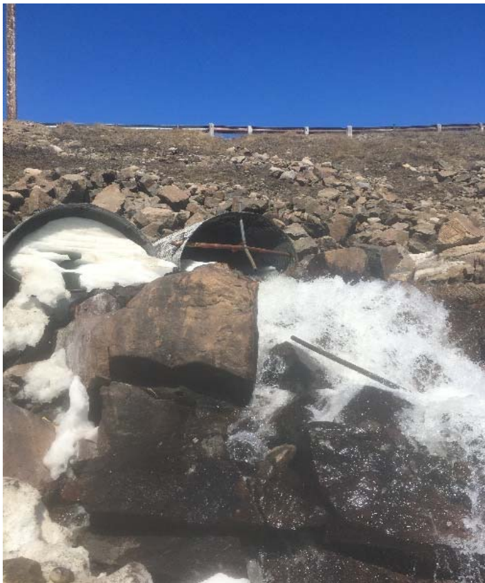
South of Crossing 10 (2x 1350 mm dia.) looking Downstream -80 m long, steep installation
