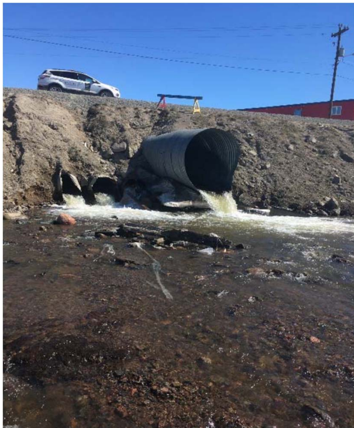
South of Crossing 12 (3 x 1000 mm dia. and 1 x 2100 mm dia.)
