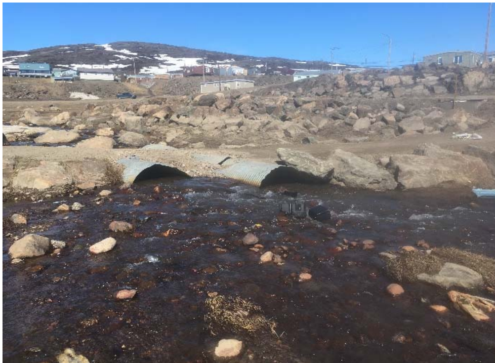
Crossing 4 (2 x 1350 mm dia.) looking North -Pipes half buried in the substrate
