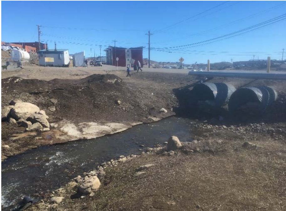
North of Crossing 8 (2 x 1950 mm dia. -22m long) looking Southeast
