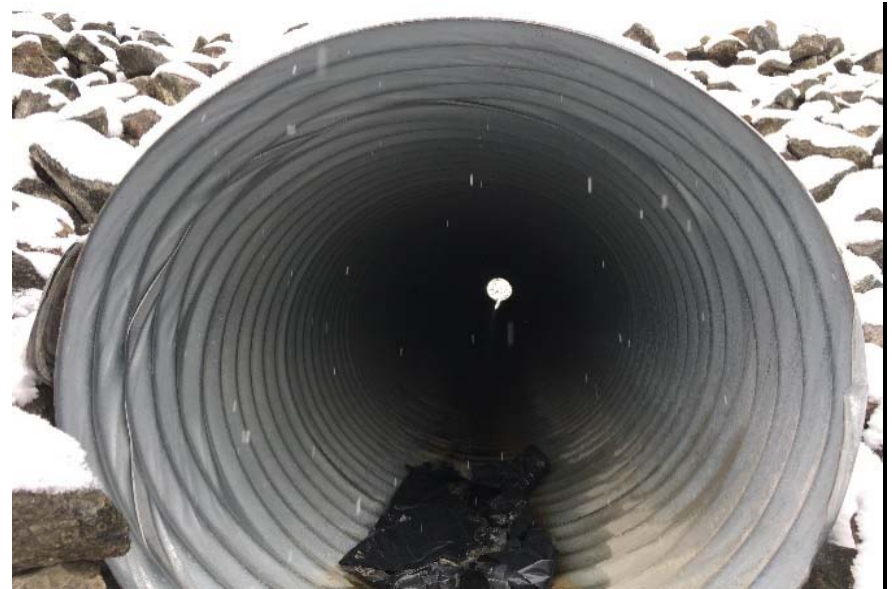
North of Crossing 4 (800 mm dia.) looking Upstream - Garbage in the pipe
