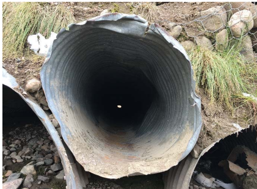
Upstream of Crossing 3 (2 x 1500 mm dia. and 1 x 620 mm dia.) -Deflected Pipe with damaged ends
