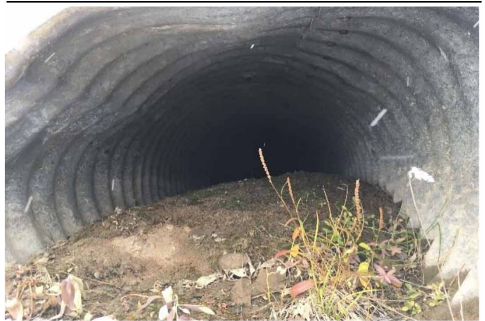
South of Crossing 7 (600 mm dia.) -Sediment buildup in the pipe
