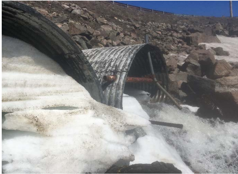
South of Crossing 10 (2 x 1350 mm dia.) looking Downstream - Blocked due to snow
