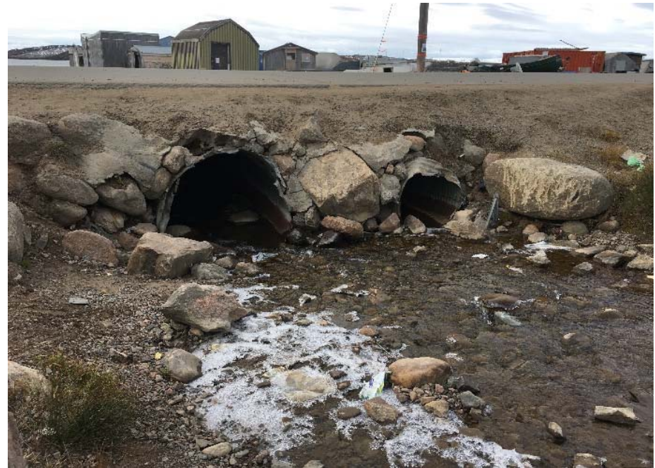
Upstream of Crossing 1 (2 x 700 mm dia.) - Damaged Ends
