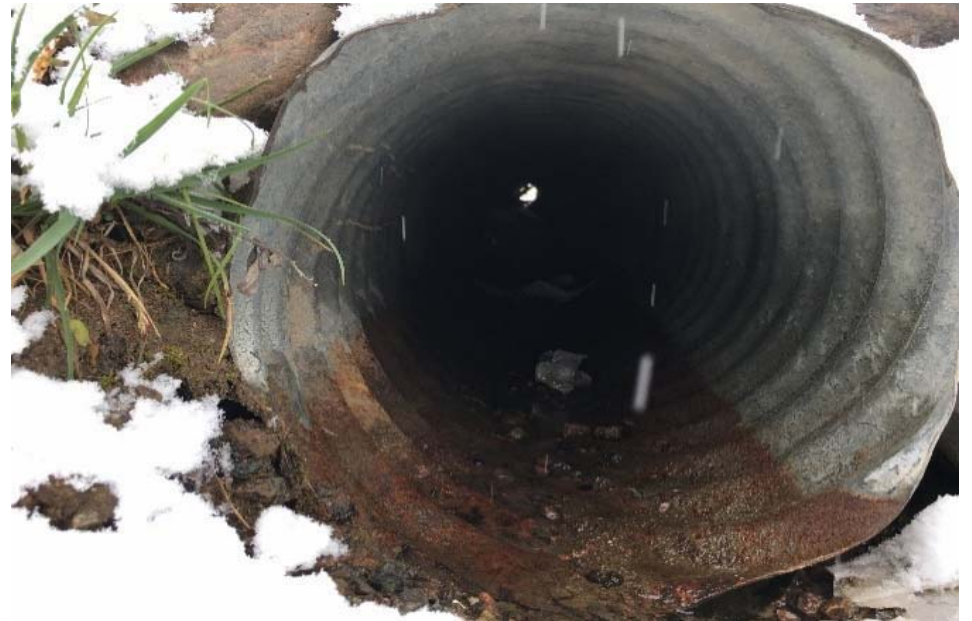
North of Crossing 5 (300 mm dia. ) looking Upstream -Corroded pipe exposed after the removal of garbage
