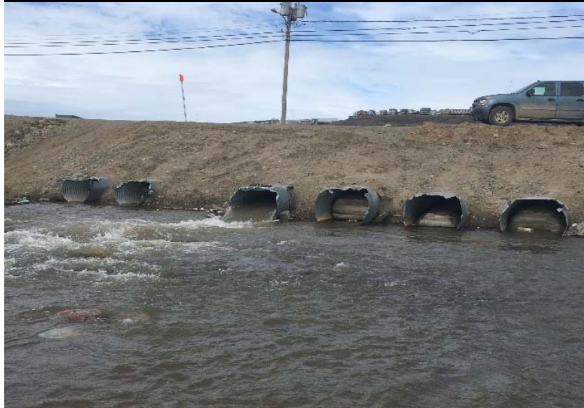
South of Crossing 3 (4 x 1200 mm dia. and 2 x 1000 mm dia.) - Damaged Ends
