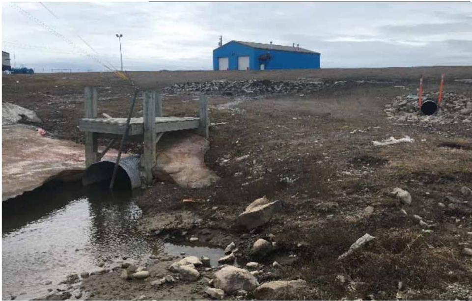
East of Crossing 6 (1200 mm dia. ) & 6B (600 mm dia. )
