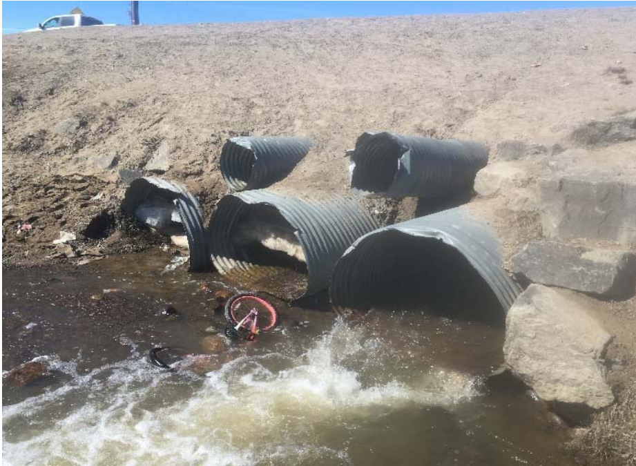
South of Crossing 3 (3 x 1500 mm dia. and 2 x 620 mm dia.) -Bike in the stream
