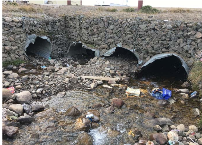
Upstream of Crossing 2 (3 x 1200 mm dia.) - Garbage in front of the pipe
