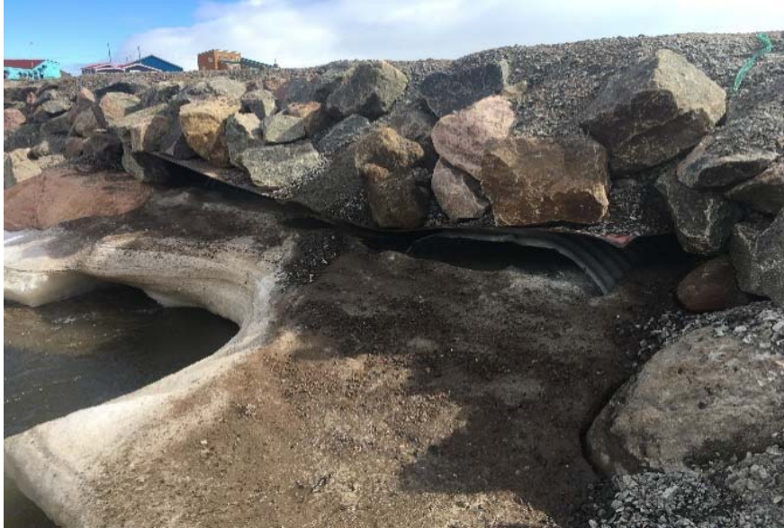
Cluster 2 (3 x 1100 mm dia.) taken from North side of road - Blocked due to snow
