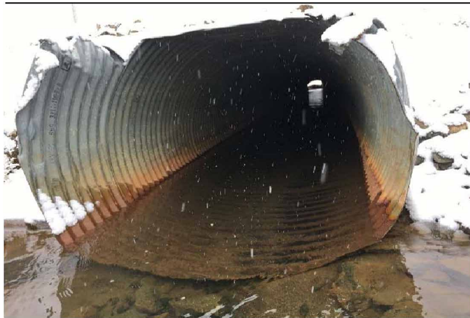
North of Crossing 3 - damaged ends
