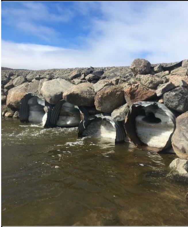
Cluster 1 of 4 Culverts (4 x 9400 mm dia.) on south side of road - Blocked due to snow
