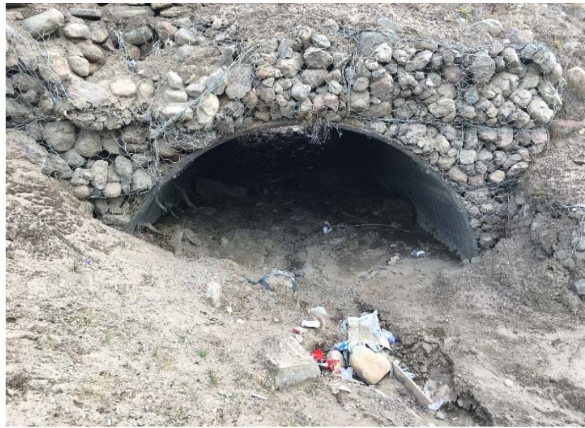
Downstream of Crossing 7 (3200 mm dia.) - Garbage infront of pipe
