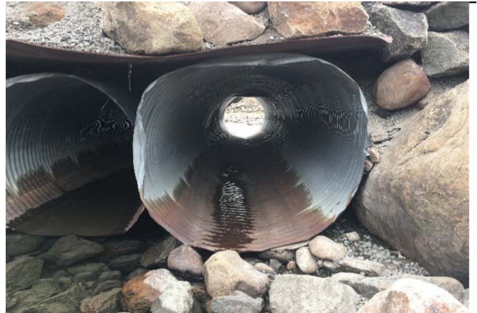
Northside of Cluster 3 - Deflected Pipe due to heavy loads
