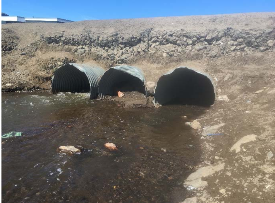
South of Crossing 2 (3 x 1200 mm dia.) - Garbage in the stream, pipe not in good shape
