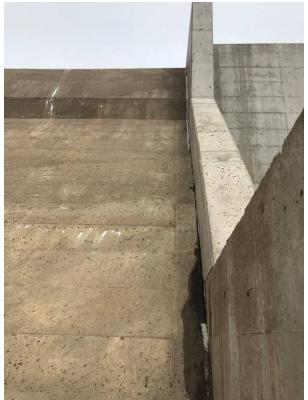
**Photograph 8:** Concrete spillway. Minor leakage through concrete right side of spillway.
