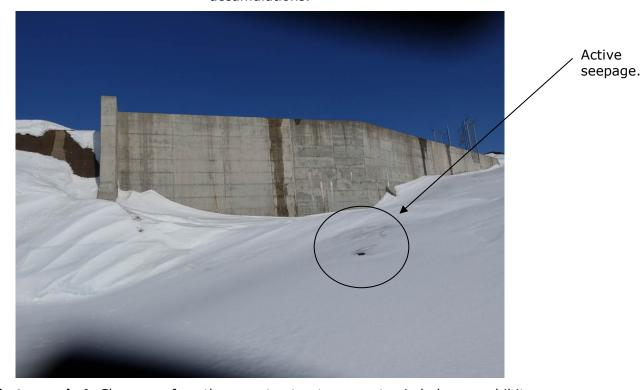
**Photograph 4:** Close-up of south concrete structure – note circled area exhibits active seepage; see also Photograph 5.
