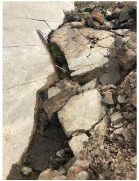
**Photograph 10:** Moving water observed at base on concrete dam below expansion joint.
