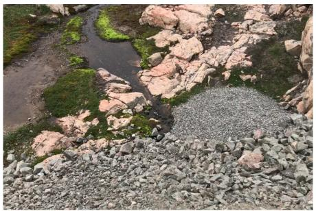
**Photograph 6:** Base of centre berm at lowest point looking south. The moving water appears to be moving through the gravel road way and towards the remaining ice in Photograph 1.
