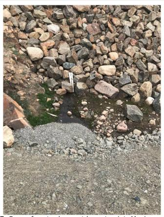
**Photograph 5:** Base of centre berm at lowest point. Moving water observed.
