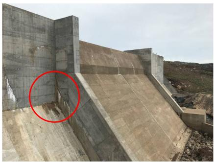
**Photograph 7:** Concrete spillway. Minor leakage through concrete left of the spillway.
