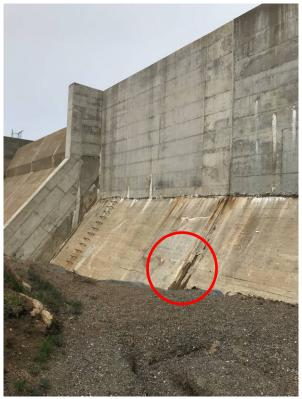
**Photograph 9:** Minor leakage to the right of the spillway at expansion joint.
