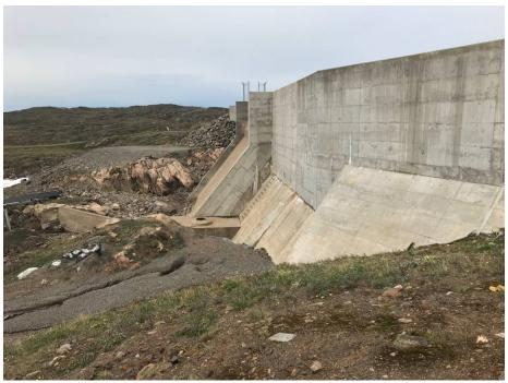
**Photograph 12:** Overview of concrete dam looking north. Soil/ granular washout bottom left of photograph.
