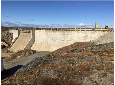
**Photograph 13:** August 27 2019 Overview of concrete dam after the completion of upstream concrete repair and crack injection. Leaking as shown in Photograph 9 is no longer present. Soil/ granular washout filled in by the contractor in August 2019.
