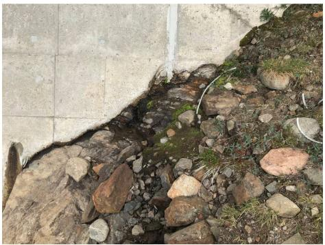
**Photograph 11:** Moving water observed at base on concrete dam below expansion joint.
