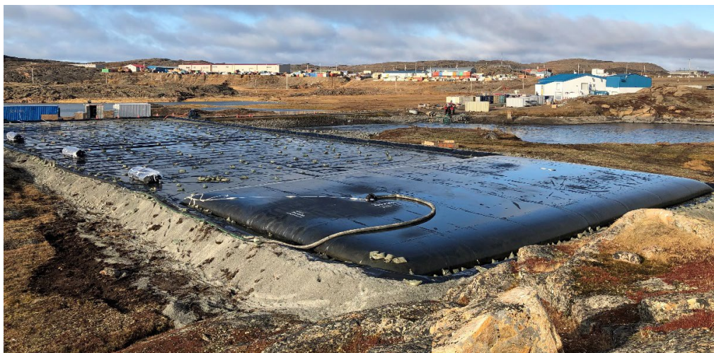
Figure 3.4 Desludging of sewage lagoon using geotubes placed on containment pad
