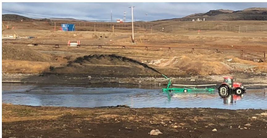
Figure 3.3 Mixing of lagoon supernatant and settled sludge during desludging
