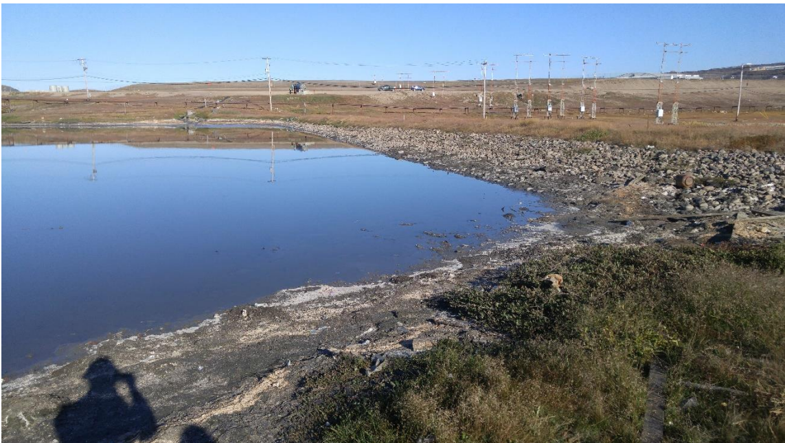
Figure 11 Exposed riprap and shoreline along the east dyke of the lagoon
