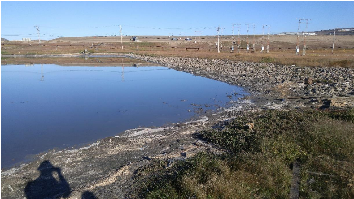
Figure 11 Exposed riprap and shoreline along the east dyke of the lagoon
