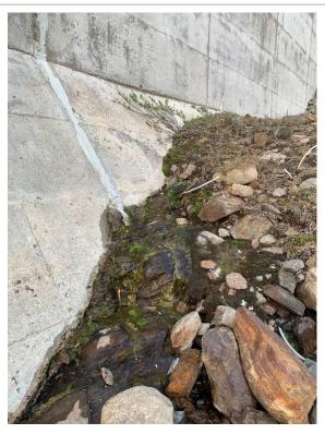
**Photograph 3** – Water seepage at base of J5 joint, south of spillway.
