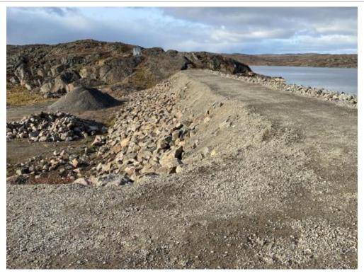
**Photograph 13 –** North beam looking northwest, edge of roadway susceptible to erosion.
