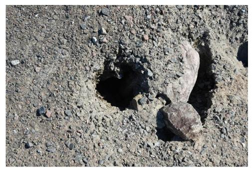
**Photograph 6** – Small sink hole located in the center berm.
