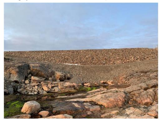
**Photograph 10 –** Seepage at valley of center berm.
