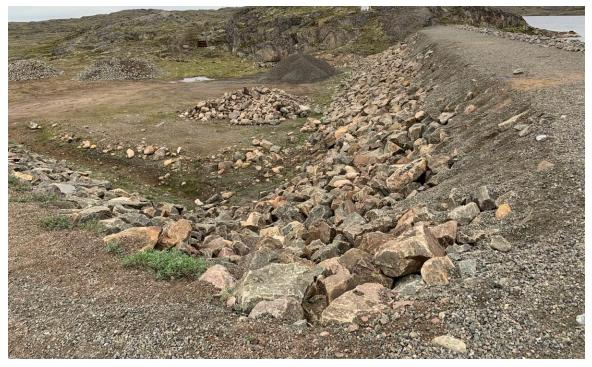
**Photograph 8 –** Downstream face of the north berm, no active seepage was noted during our site visit.
