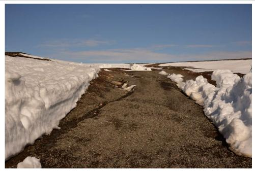
**Photograph 5** – Typical erosion of the north access road.
