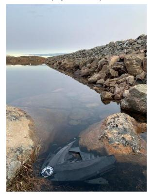
**Photograph 8** –Steep slope of rip rap on upstream side of berm. Snowmobile debris within reservoir.
