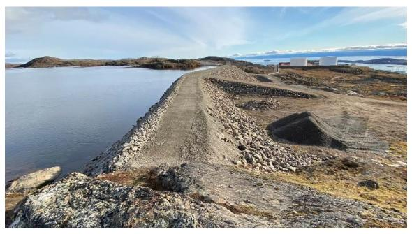
**Photograph 12** – North and center berms and north access road ramp, looking southeast.
