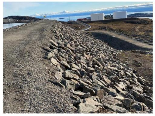
**Photograph 14 –** Overview of center berm, note steel slope and edge of roadway susceptible to erosion.
