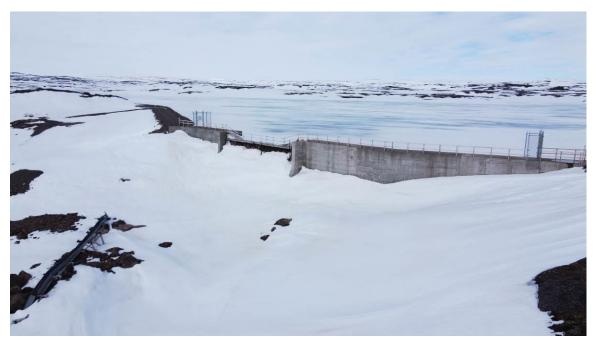
**Photograph 1** – Overview of concrete structure, center berm and north berm.
