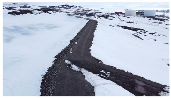
**Photograph 3 –** Typical berm condition, center berm and access ramp.
