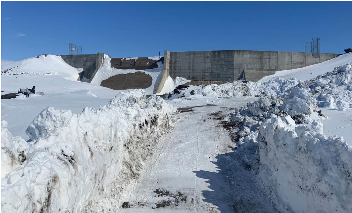
Photograph 1 – Overview of concrete structure, center berm and north berm.
