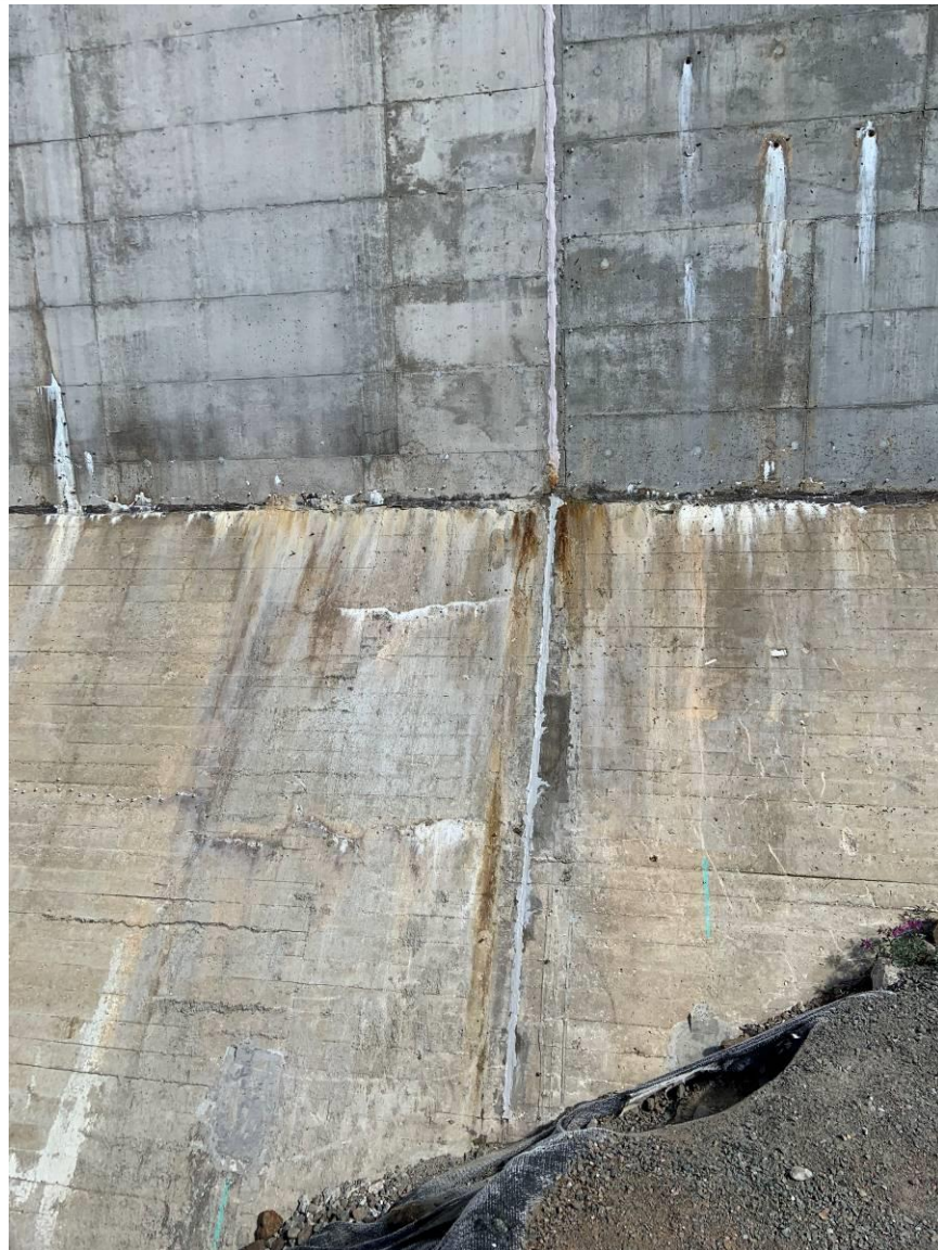
Photograph 5 – Typical expansion joint (concrete dam).
