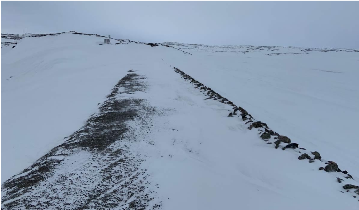
Photograph 3 – Typical north berm condition at the time of our review.
