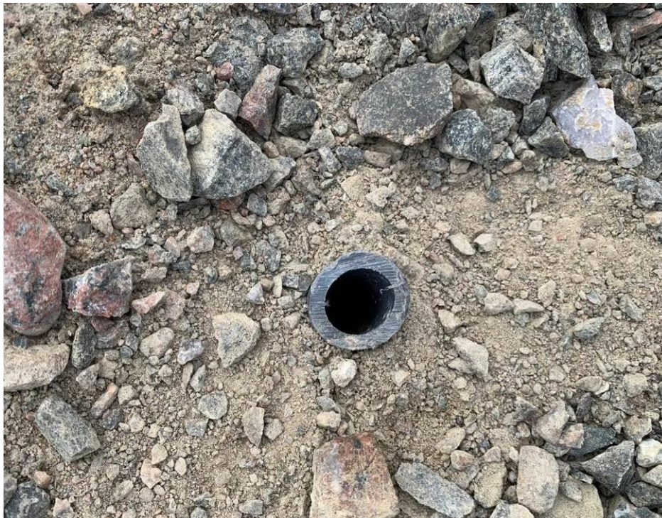
Photograph 6 – Borehole tube for piezometer (open).
