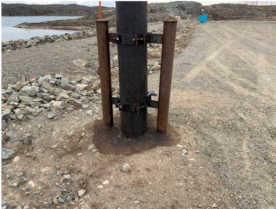
Photograph 4 – Oil residue on the ground around the base of the hydro pole, south berm.
