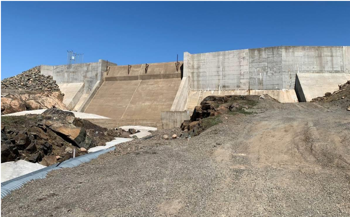
Photograph 1 – Overview of concrete structure.
