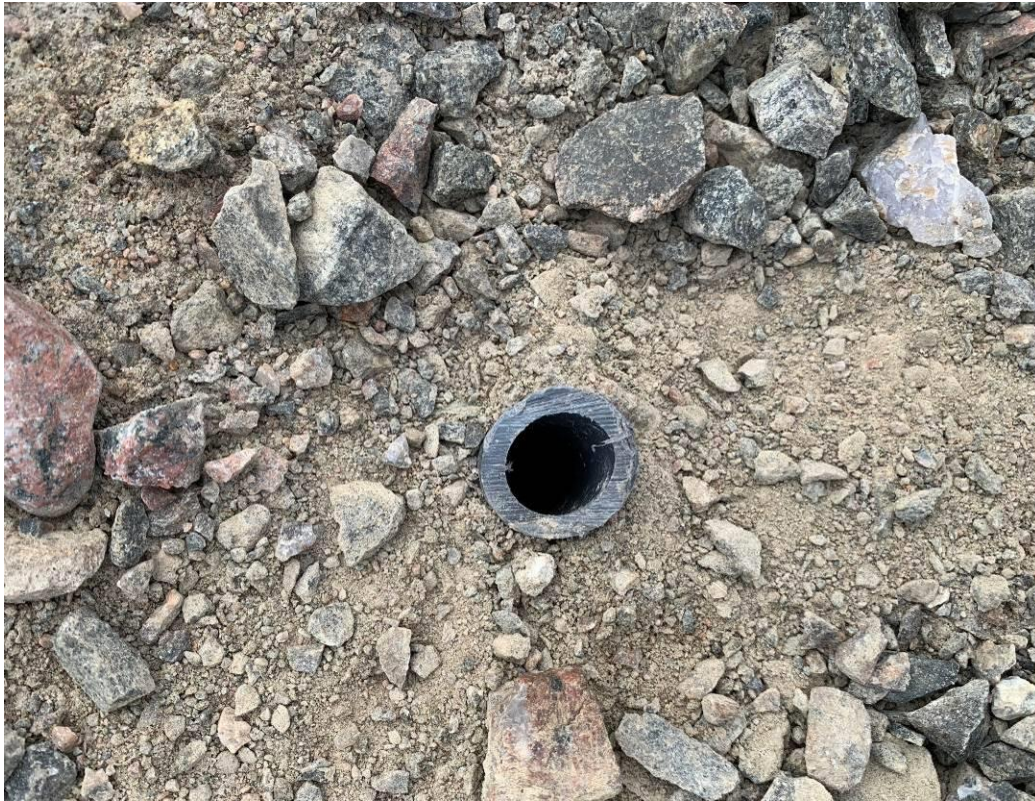
Photograph 6 – Borehole tube for piezometer (open).
