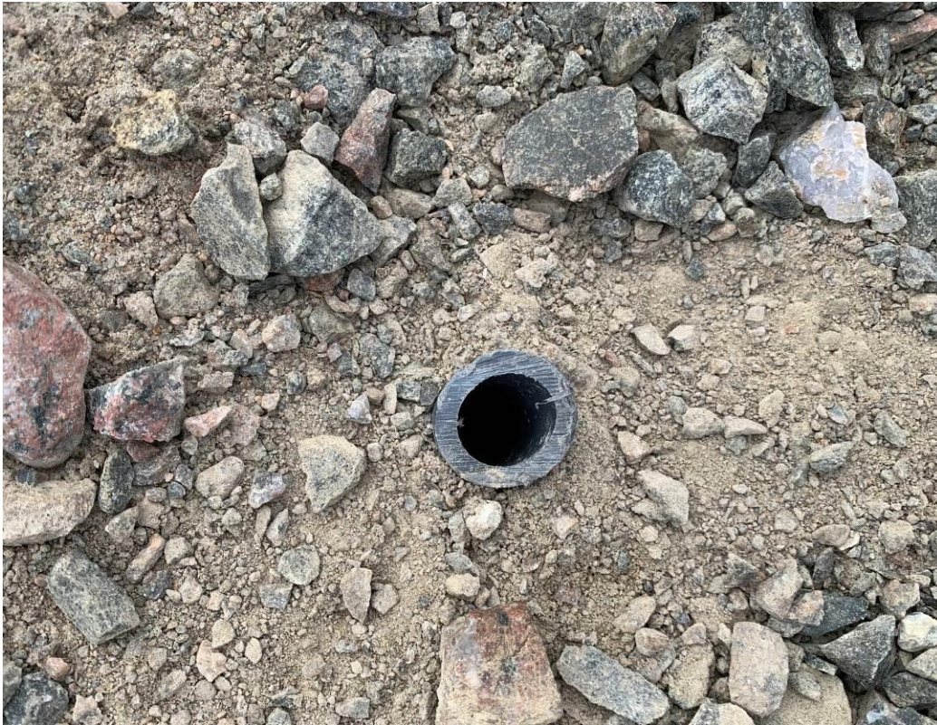
Photograph 9 – Borehole tube for piezometer (open).
