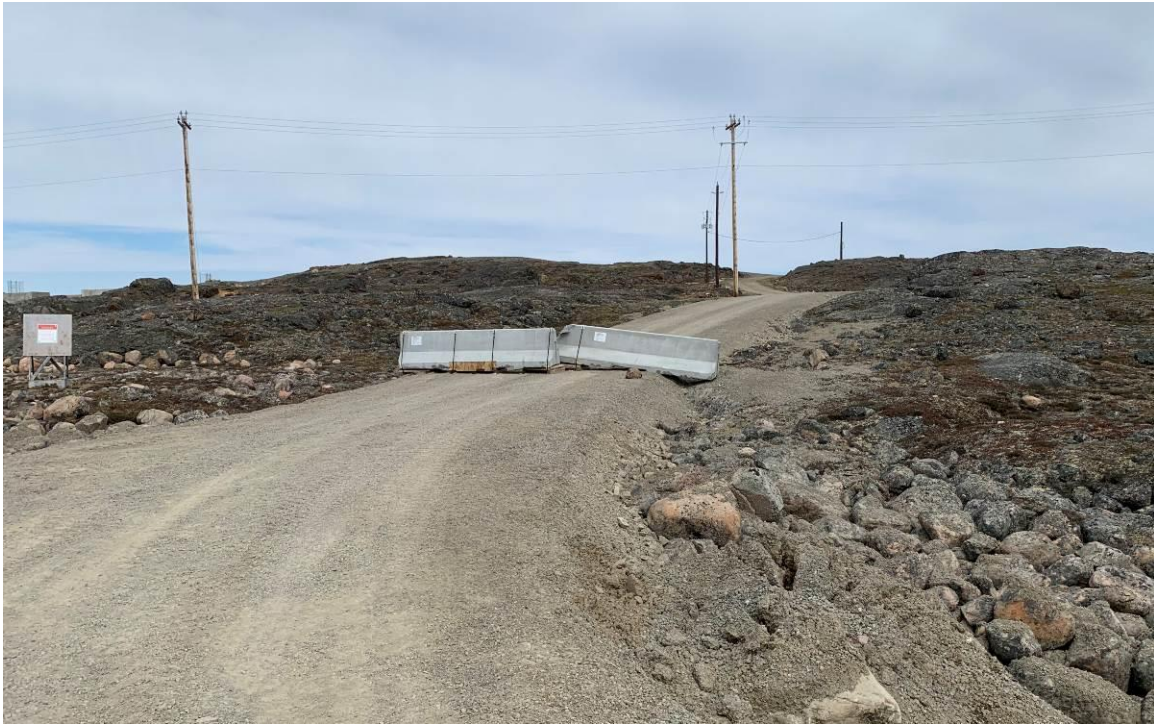
Photograph 4 – The temporary road to south berm has been blocked with a concrete barrier to limit public access to the dam and reservoir.
