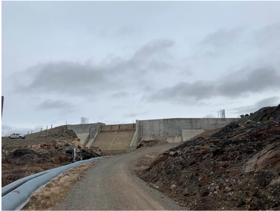
Photograph 1 – Overview of concrete structure.
