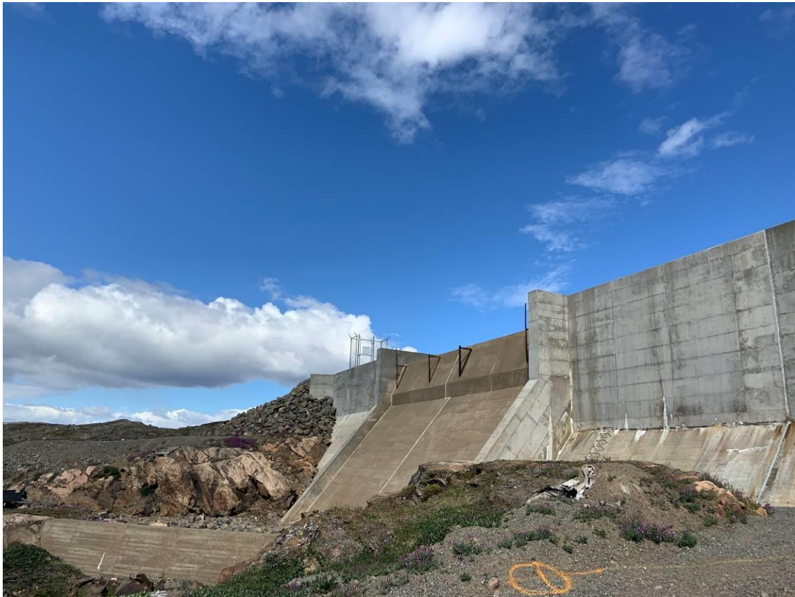
Photograph 1 – Overview of concrete structure.
