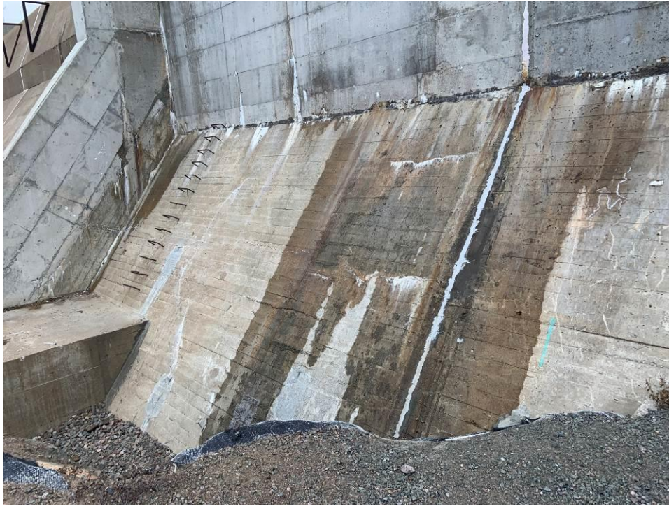
Photograph 5 – Typical expansion joint (concrete dam).
