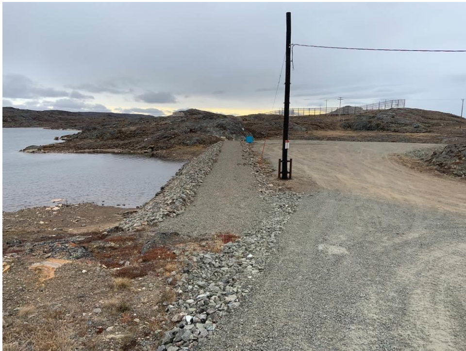
Photograph 2 – Typical south berm condition at the time of our review.
