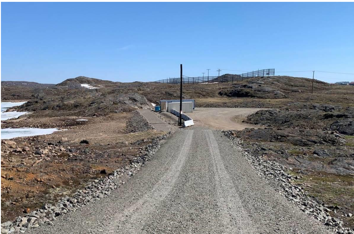
Photograph 2 – Typical south berm condition at the time of our review.
