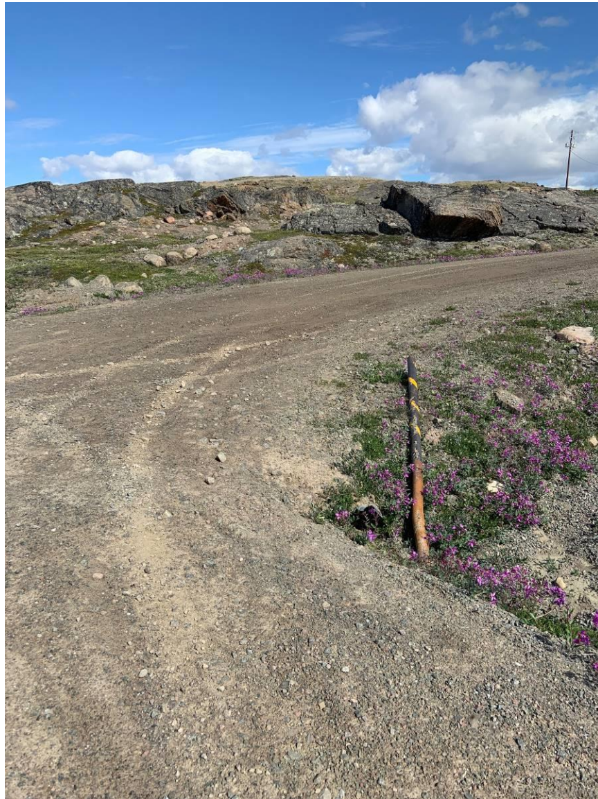
Photograph 8 – Corner marker at the junction of the south access road and the road to the south berm has been knocked over.
