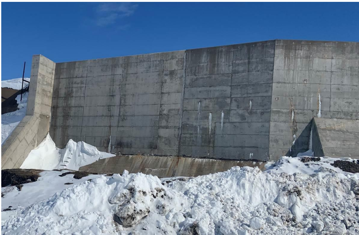
Photograph 8 – Typical concrete condition, south of the spillway.
