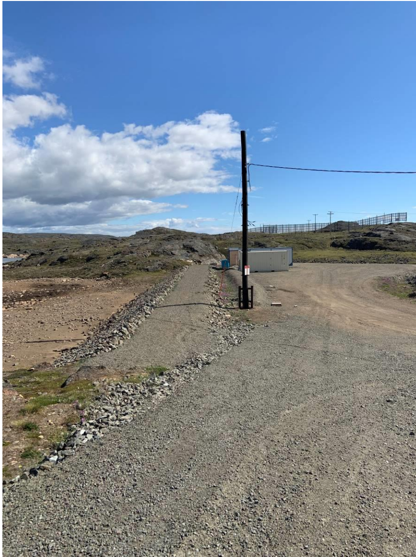
Photograph 2 – Typical south berm condition at the time of our review.
