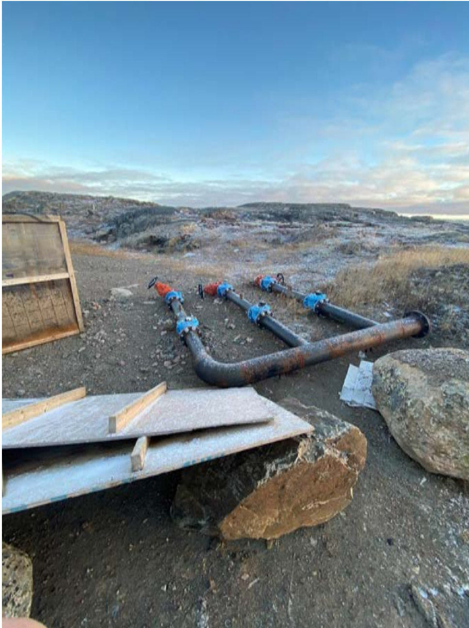
Figure 7: Apex River pumps manifold outside the Coke Plant (Oct.19).
