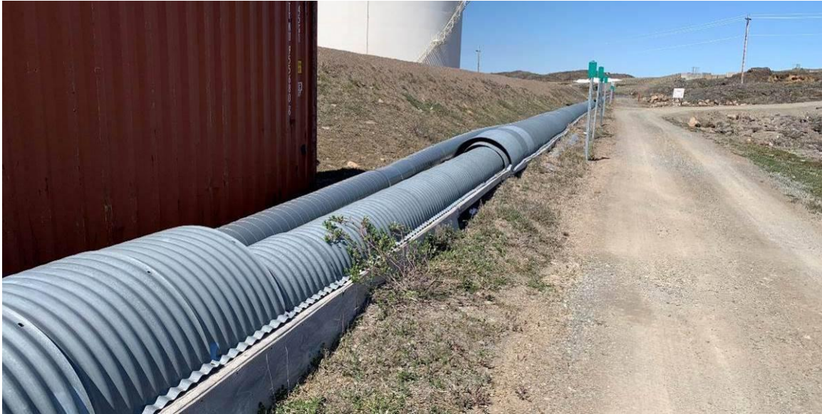
Photograph 12 – Section of the supply pipe from the dam with the corrugates metal enclosure removed.
