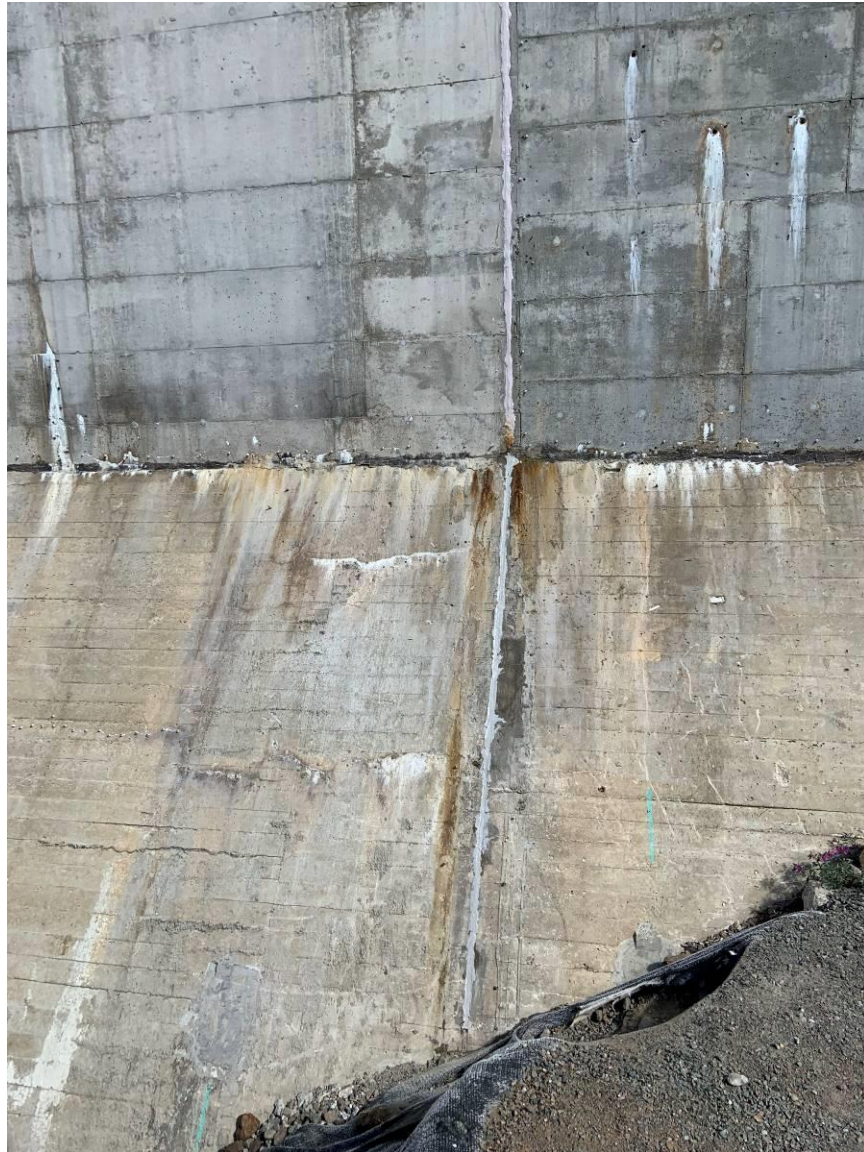
Photograph 5 – Typical expansion joint (concrete dam).
