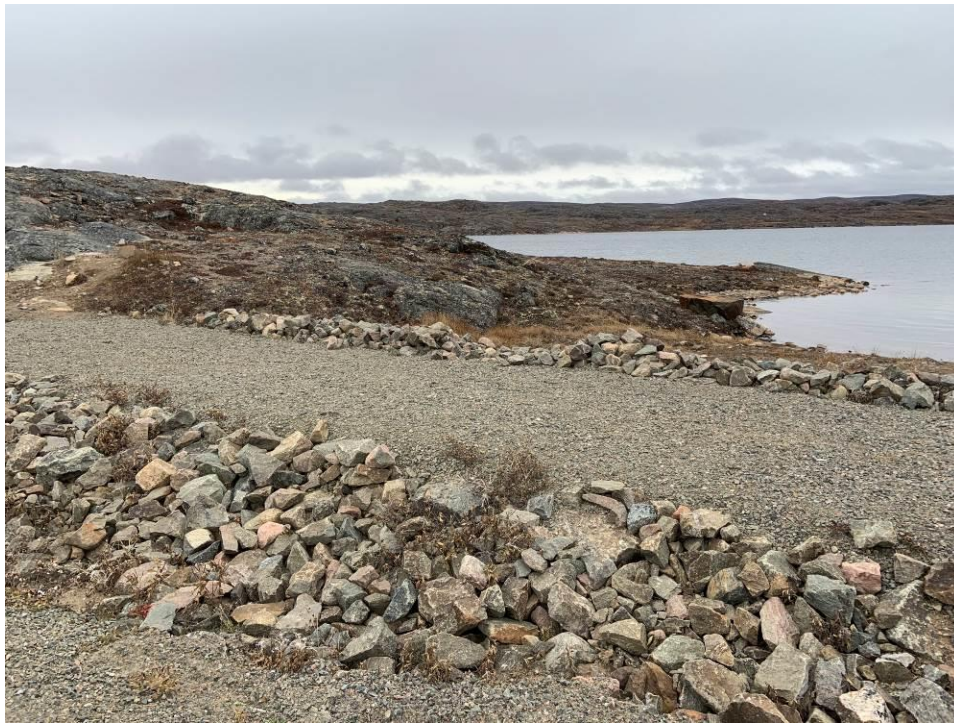
Photograph 12 – Displaced rip rap in South Berm.
