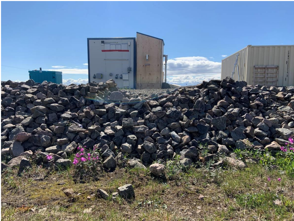
Photograph 12 – Displaced rip rap in South Berm
