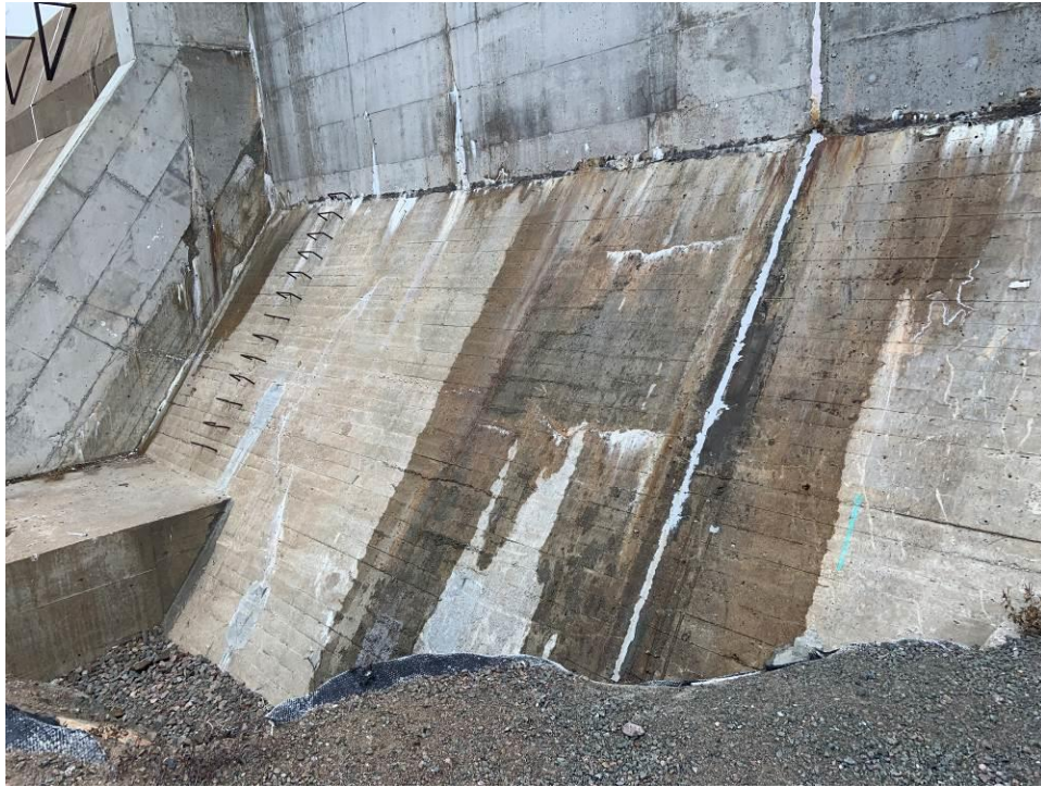
Photograph 5 – Typical expansion joint (concrete dam).
