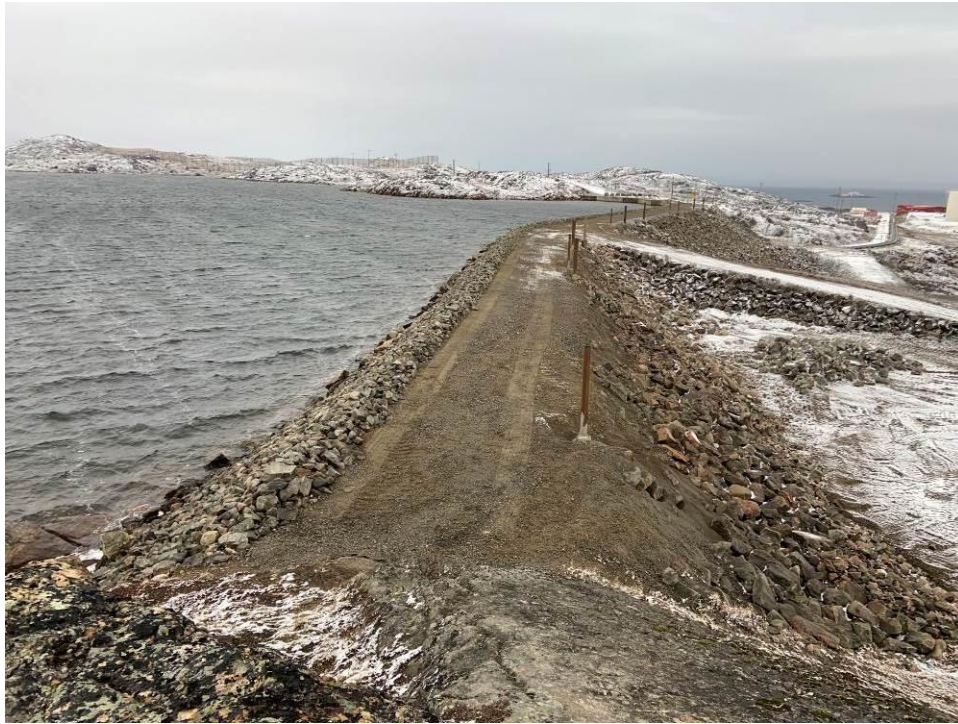
Photograph 3 – Typical north and center berm condition at the time of our review. New monitoring stations installed.
