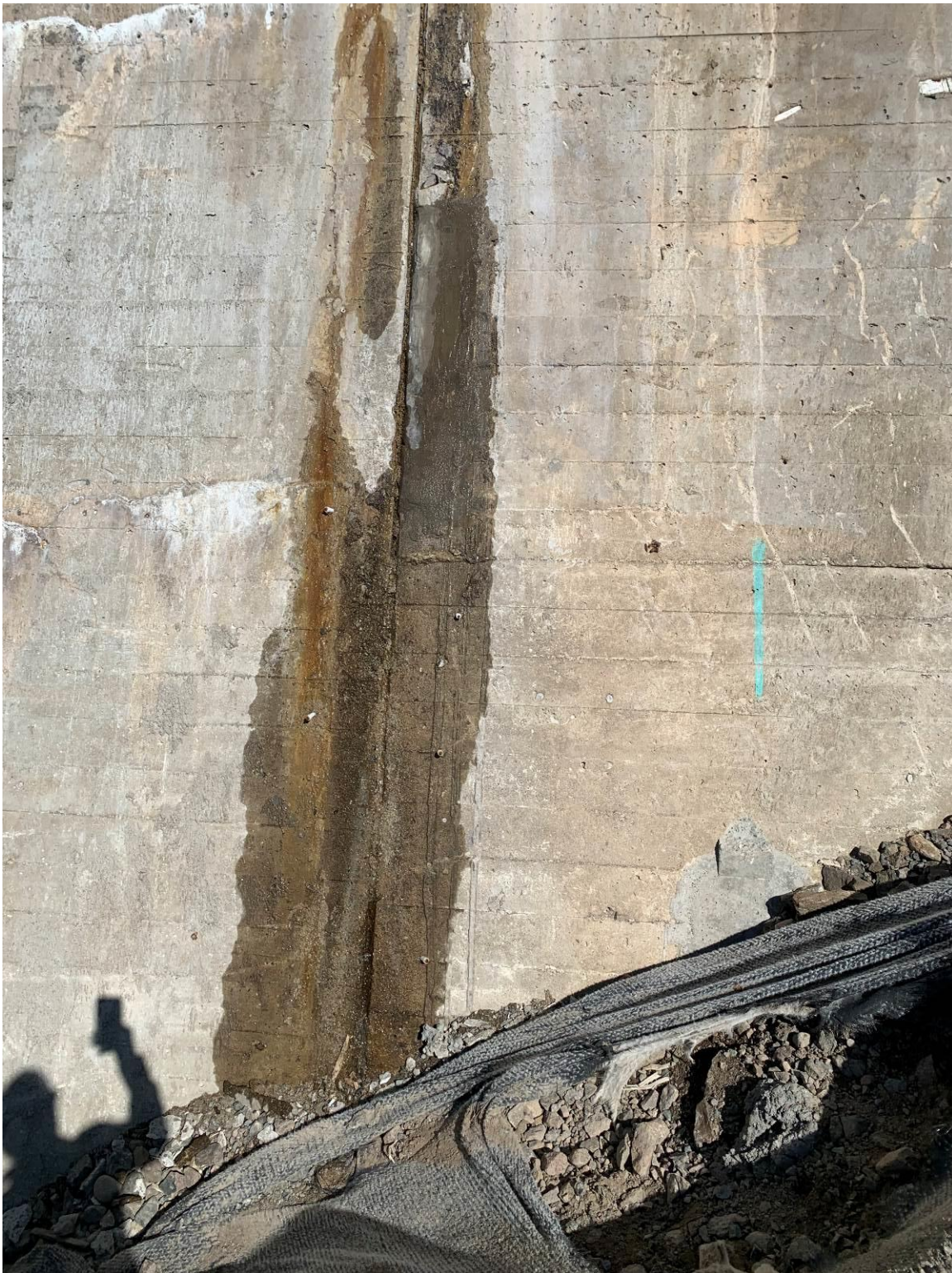
Photograph 8 – Typical expansion joint seepage (concrete dam).
