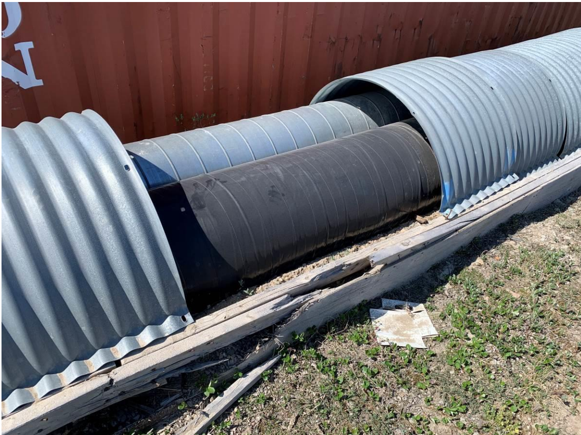
Photograph 13 – Section of the supply pipe from the dam with the corrugates metal enclosure removed.
