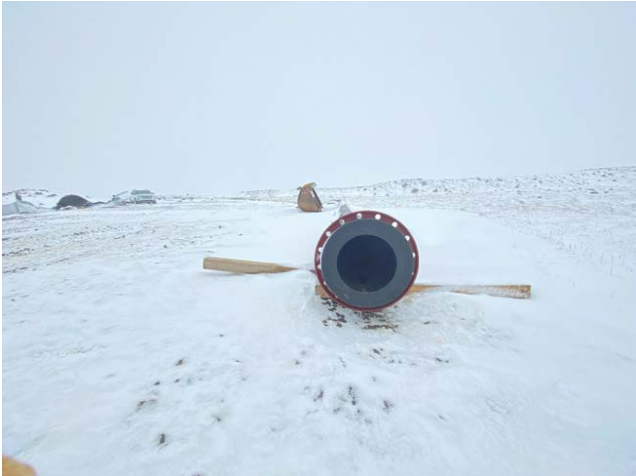
Figure 9: HDPE line at Unnamed Lake to be capped (Oct.3).
