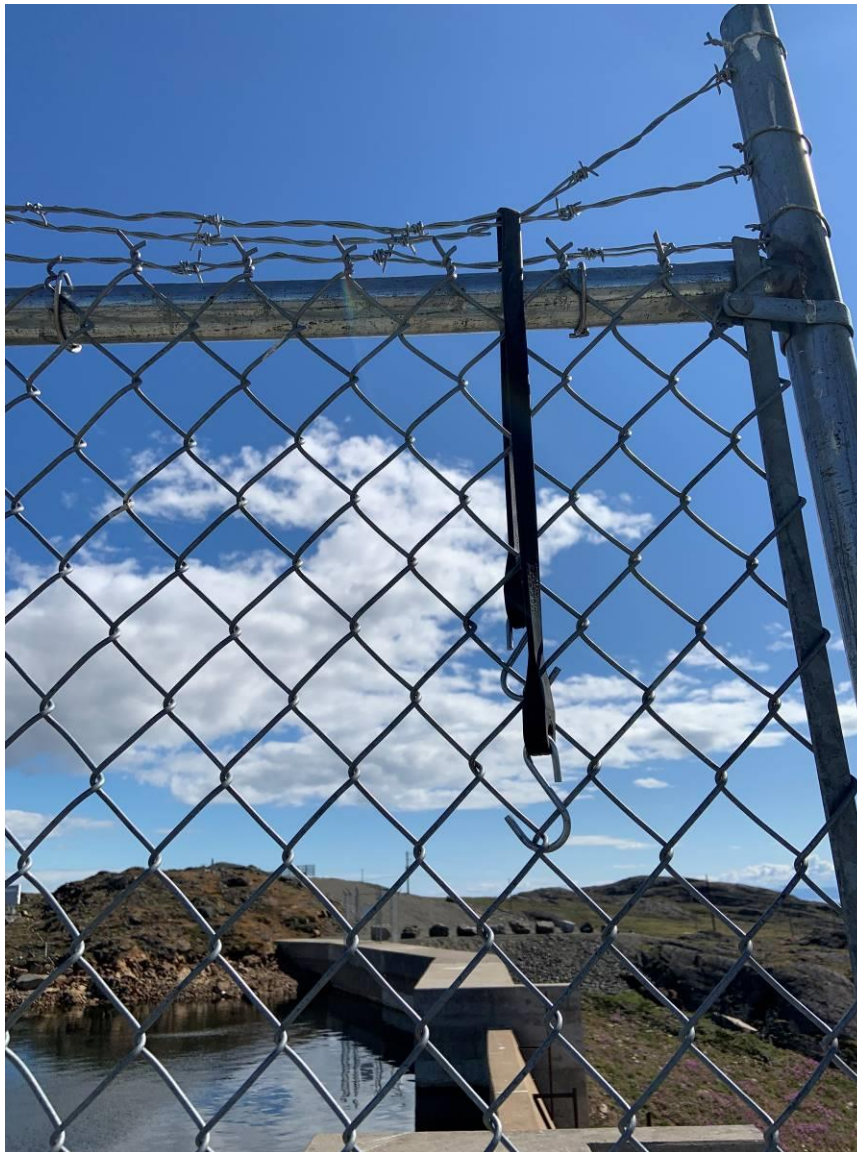
Photograph 11 – Bungee cord suppressing barbed wire
