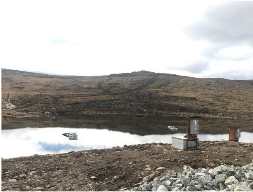
Figure 1-2: Existing pumps and fish screens in Apex River
