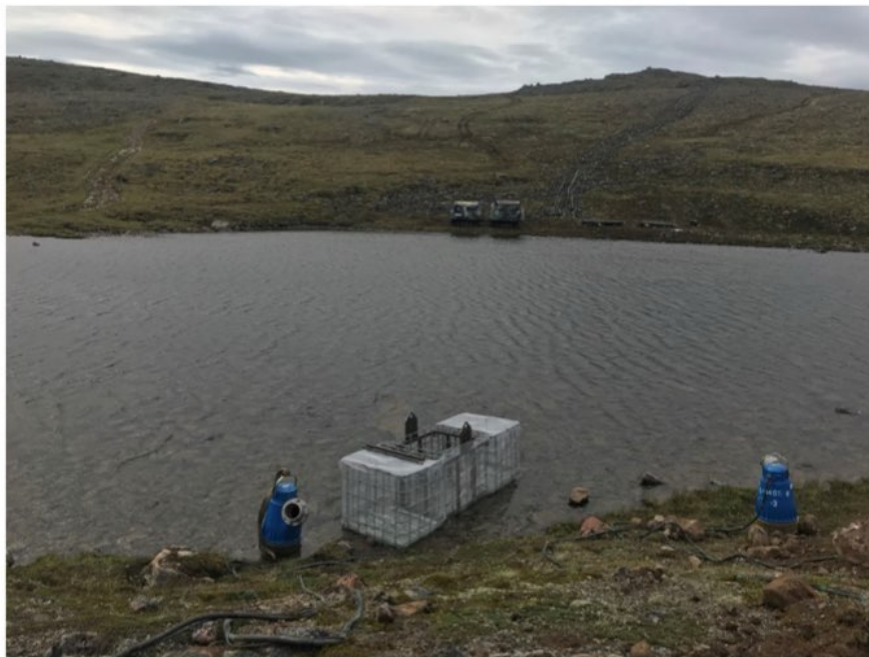
Figure 1-1: Existing submersible pumps and fish screen
