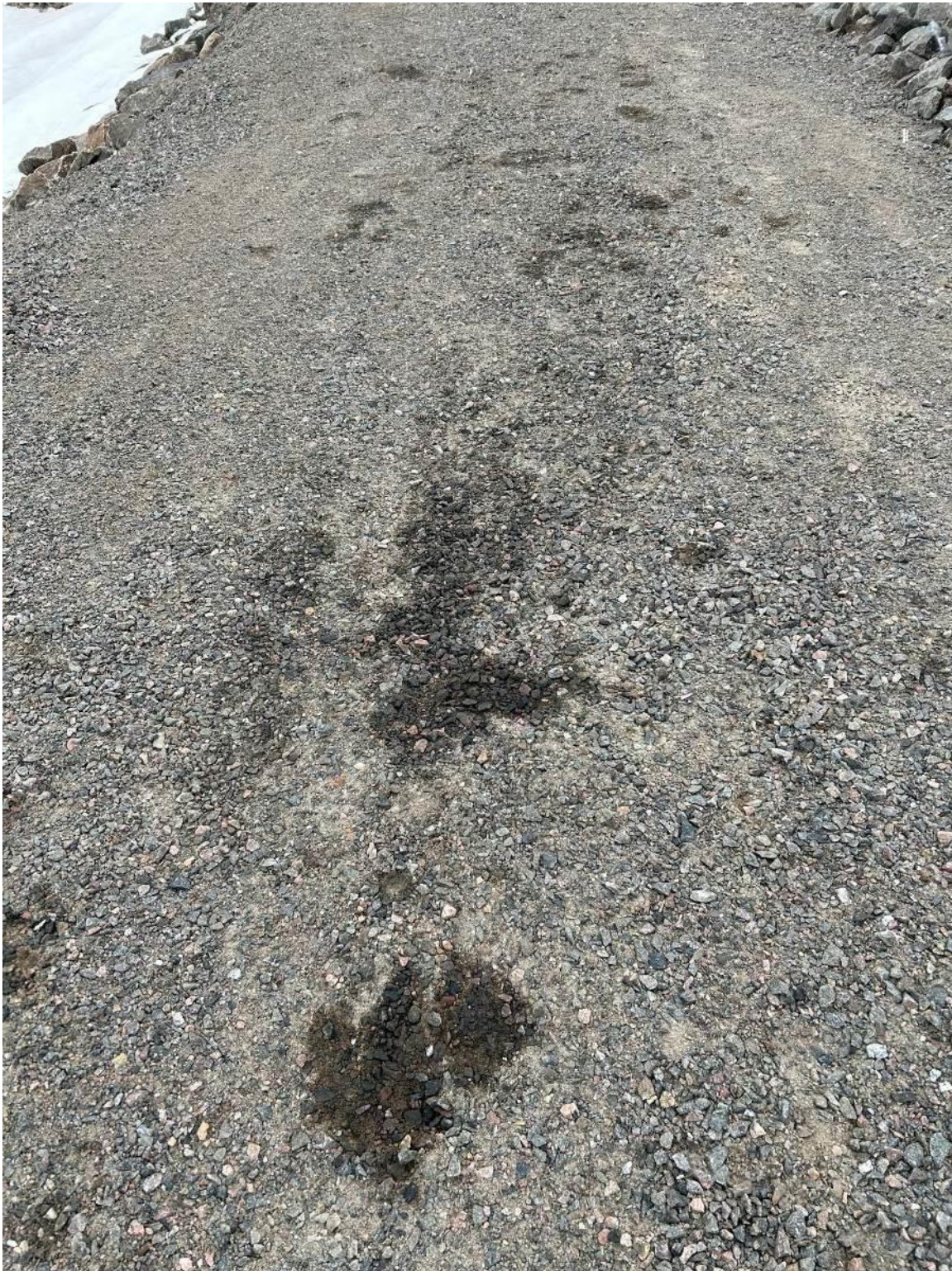
Photograph 7 – Oil residue (hydraulic fluid) atop the center berm from drill rig.
