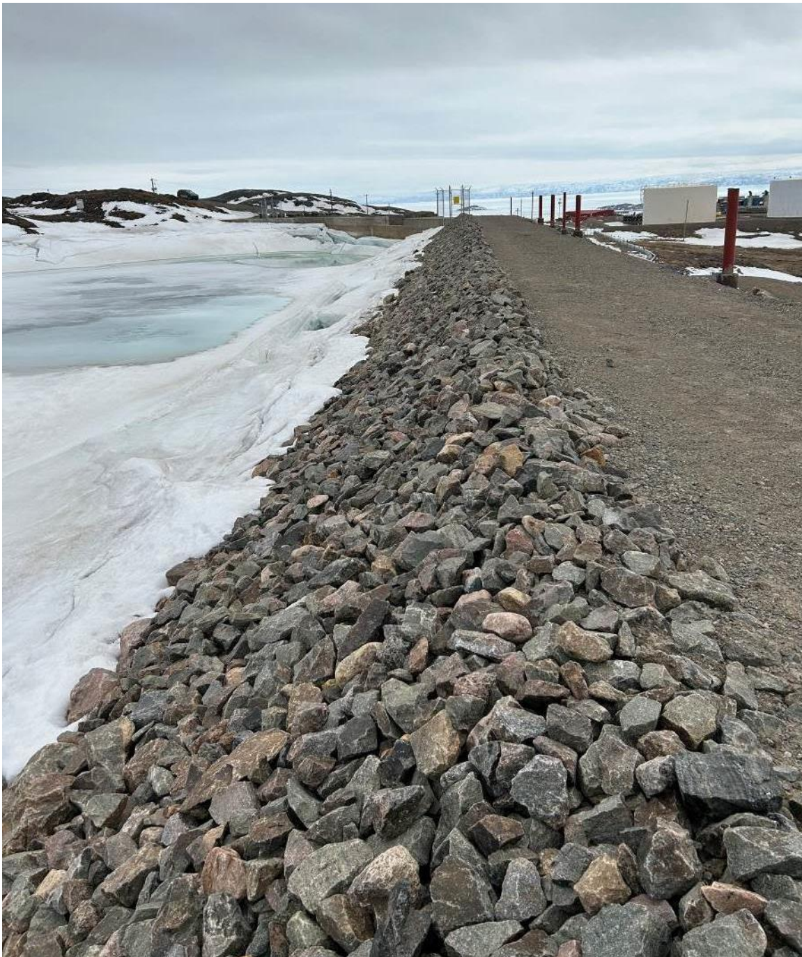
Photograph 8 – Typical condition of the rip-rap on the upstream face of the center berm.
