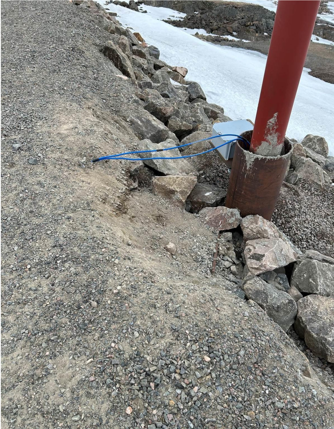
Photograph 11 – Typical data logger casing (pile), note a large section of the earthen berm has been moved during the installation of the pile. The contractor has been advised by Concentric to correct this issue at all impacted locations.
