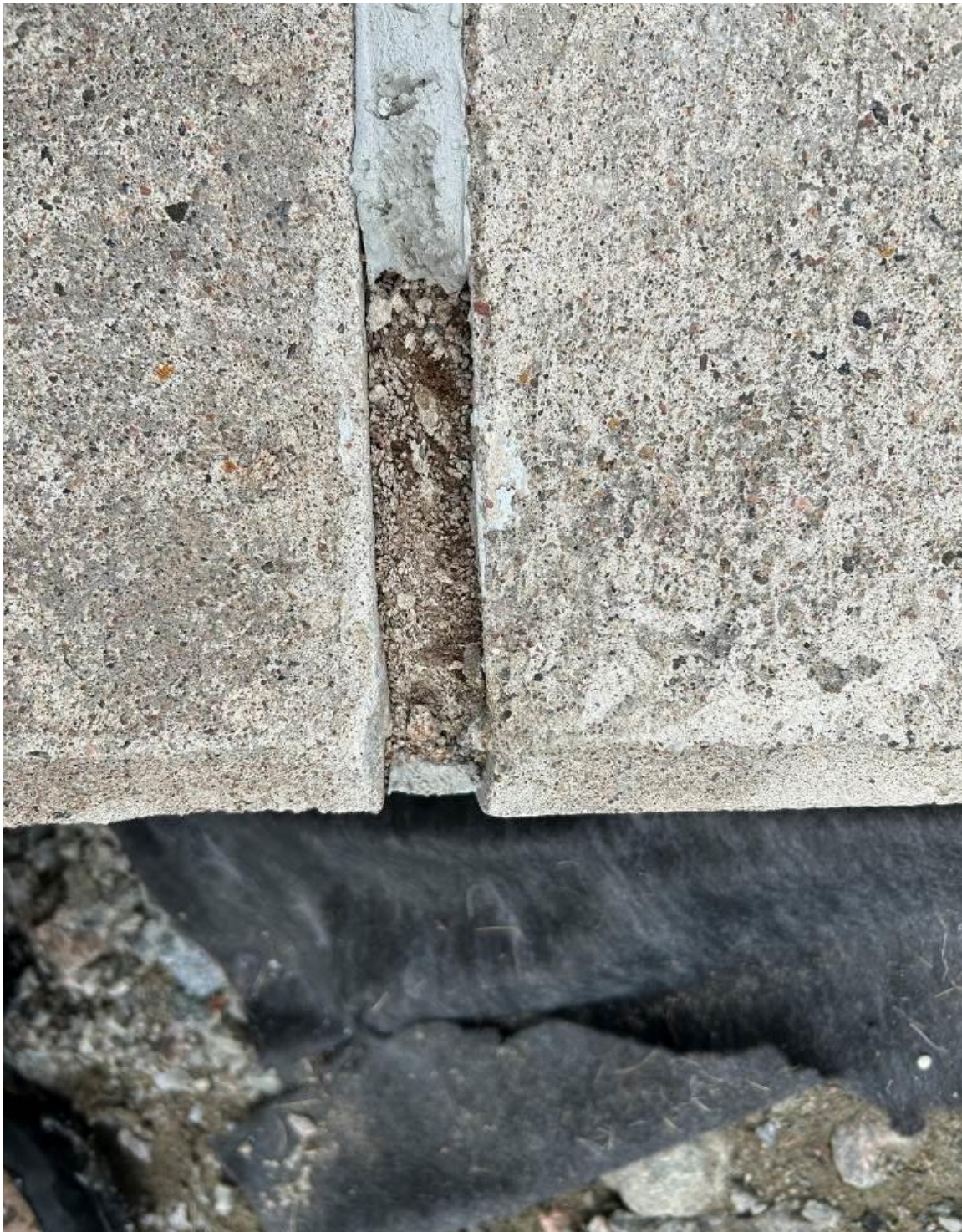
Photograph 9 – Deteriorated section of the expansion joint sealant (top of dam).
