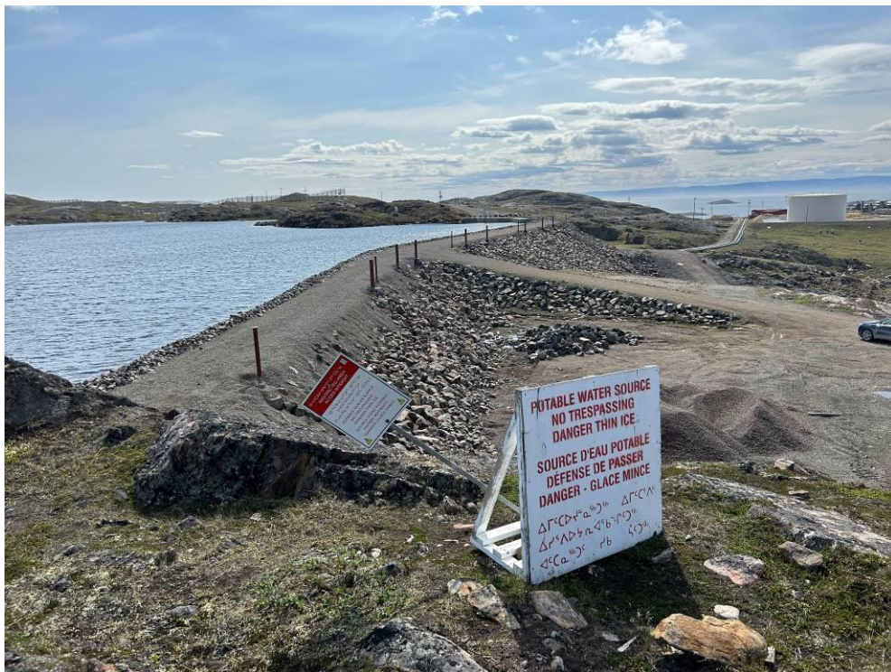
Photograph 18 – Signage at the North end of the North berm is falling over.
