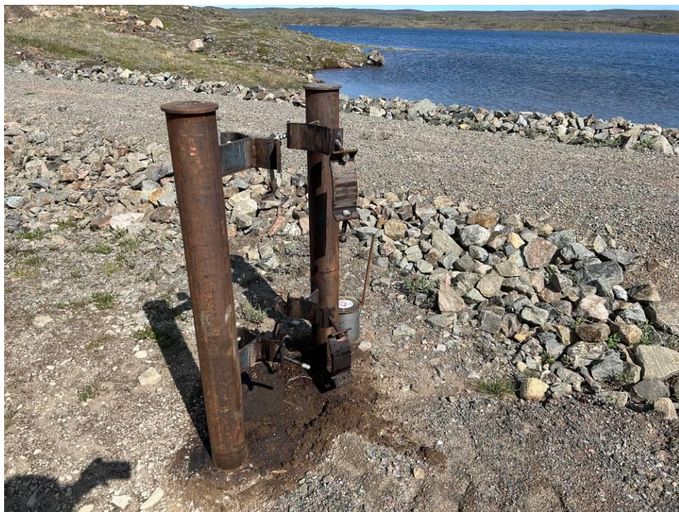
Photograph 8 – Hydro pole removed from pile braces at the downstream face of the South Berm. Note creosote contamination in the soil.
