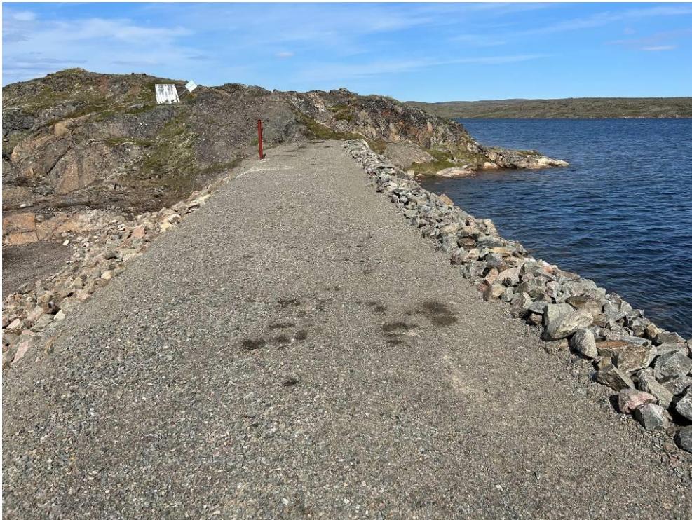
Photograph 10 – Oil residue (hydraulic fluid) atop the center berm from drill rig.
