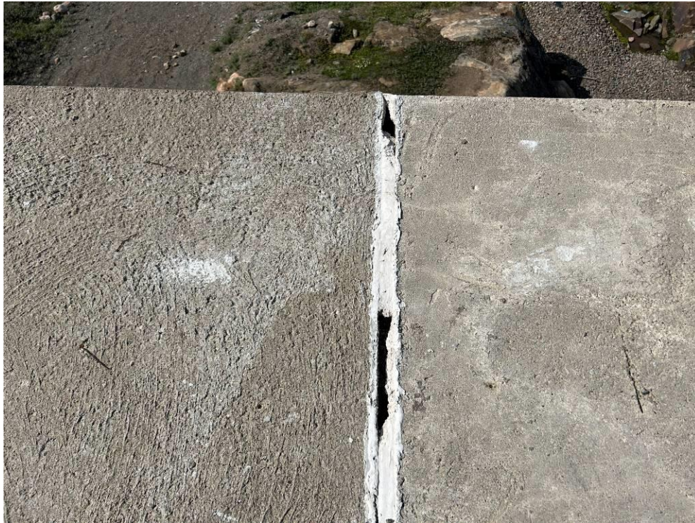
Photograph 11 – Deteriorated section of the expansion joint sealant (top of dam).
