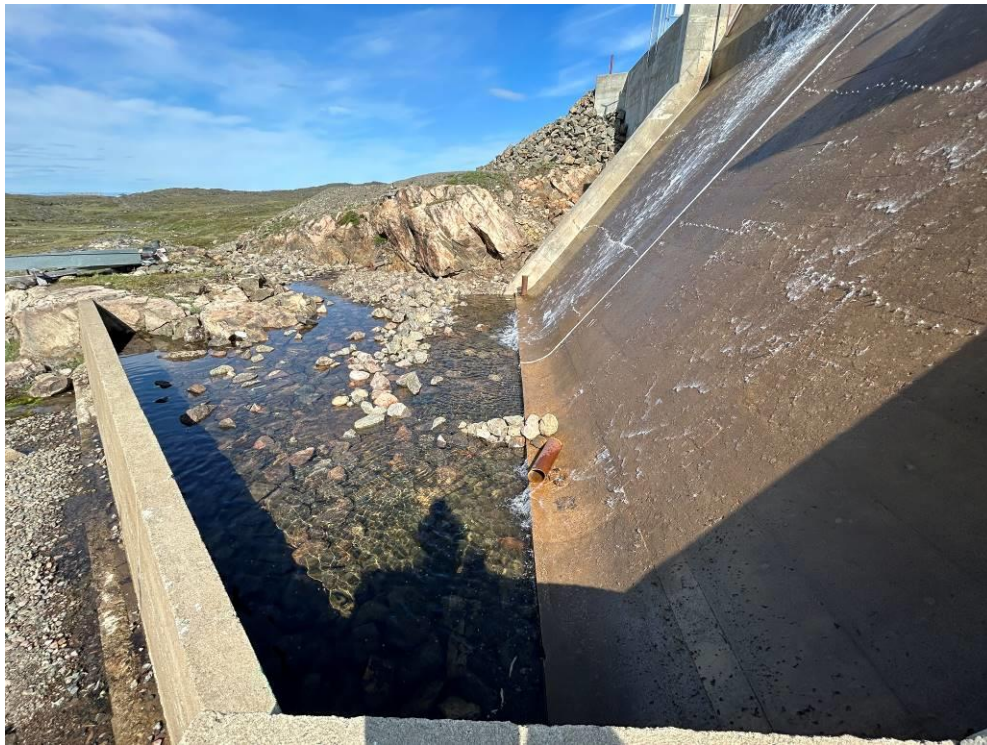
Photograph 13 – Piezometer cap is knocked off of its base at the South end of the spillway.
