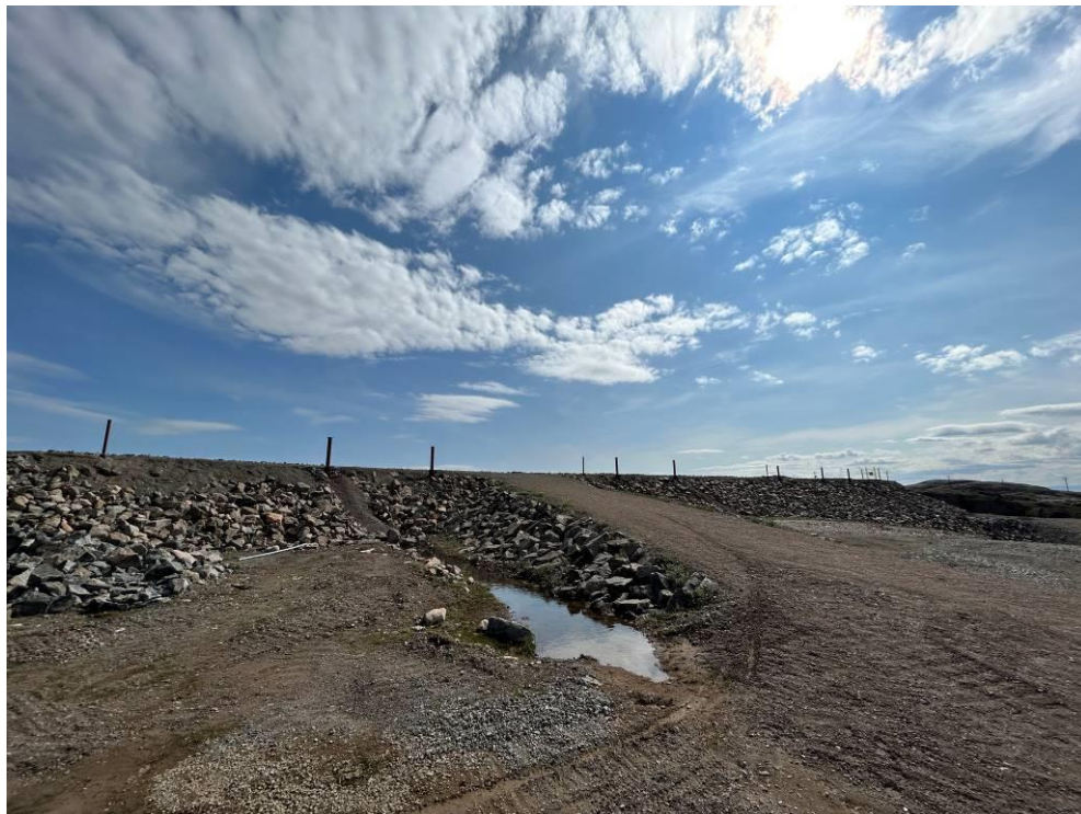
Photograph 16 – Ponding at the North side of the access ramp to the North and Centre berms.
