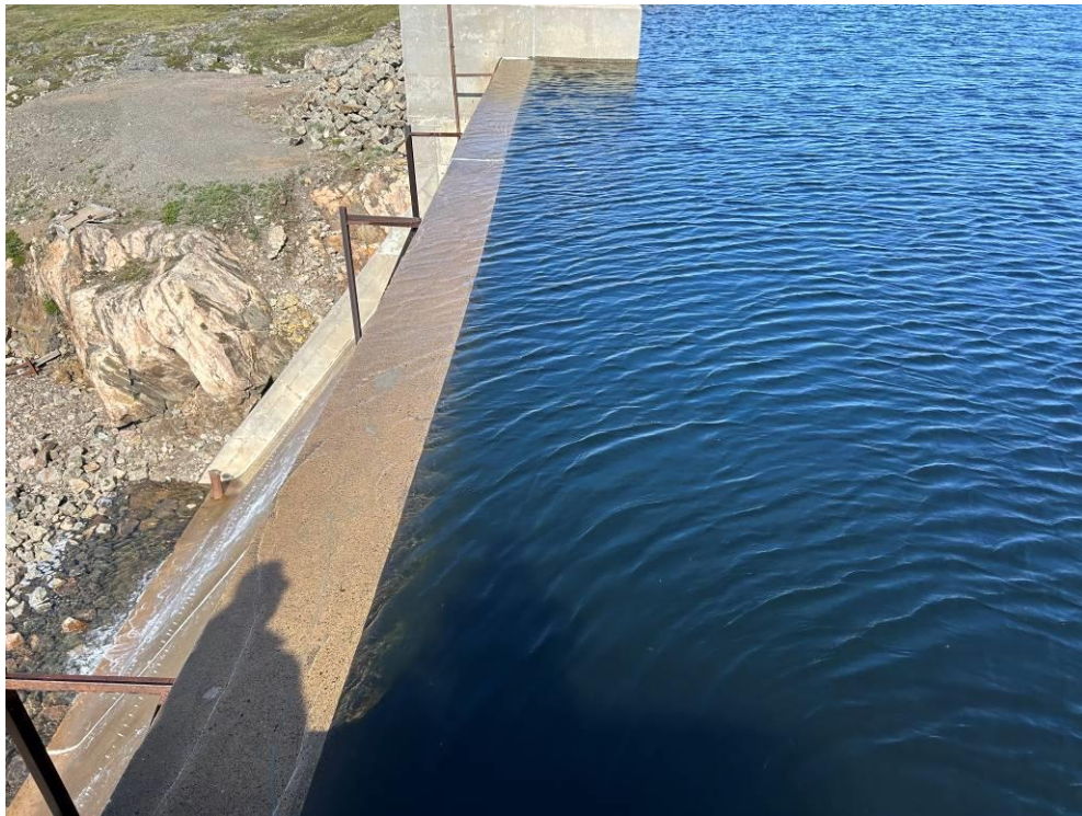
Photograph 15 – Water level spilling over the spillway.
