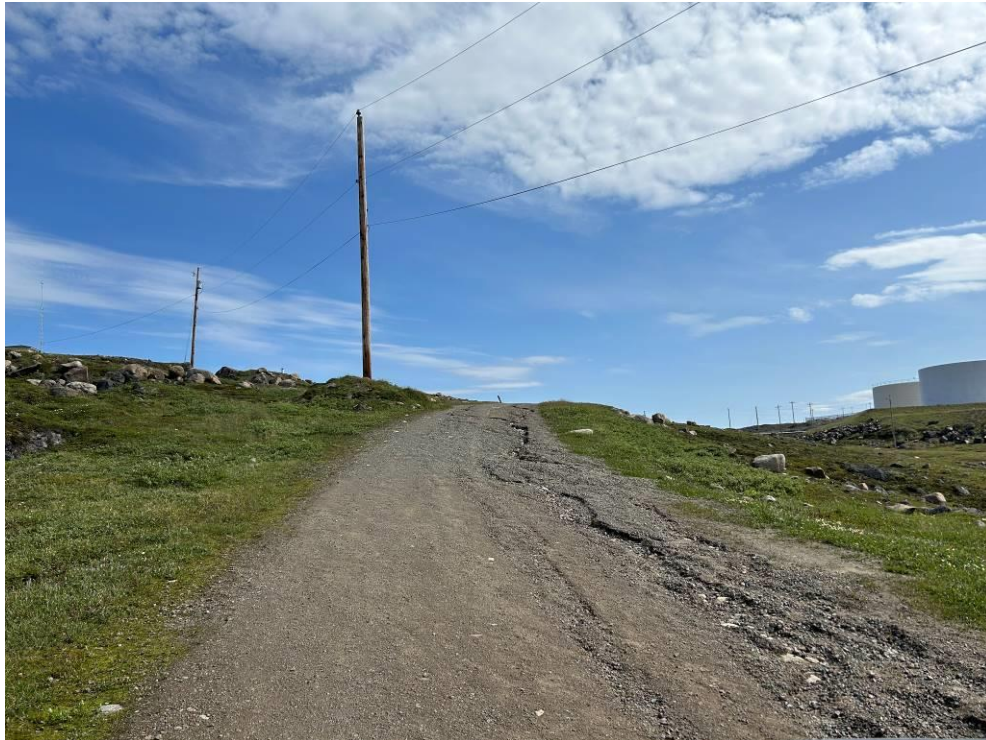
Photograph 17 – Erosion on the North access road due to spring melt.
