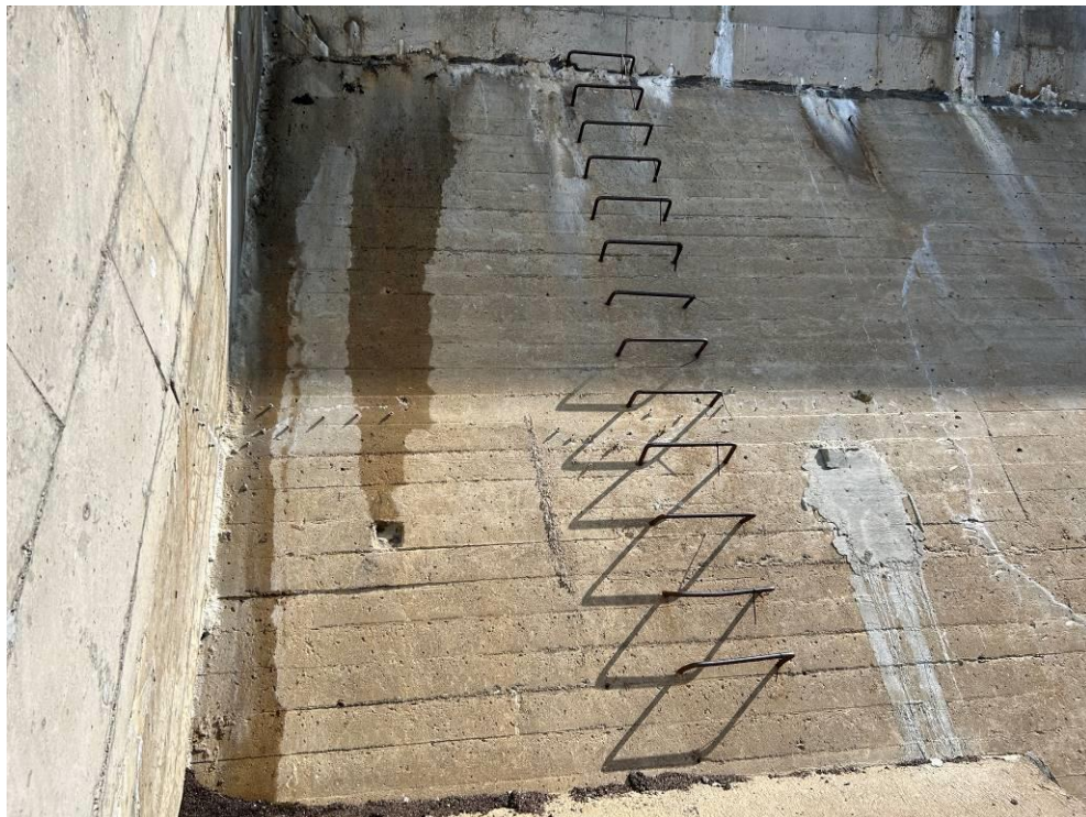
Photograph 14 – Seepage adjacent to buttress along Gridline I.
