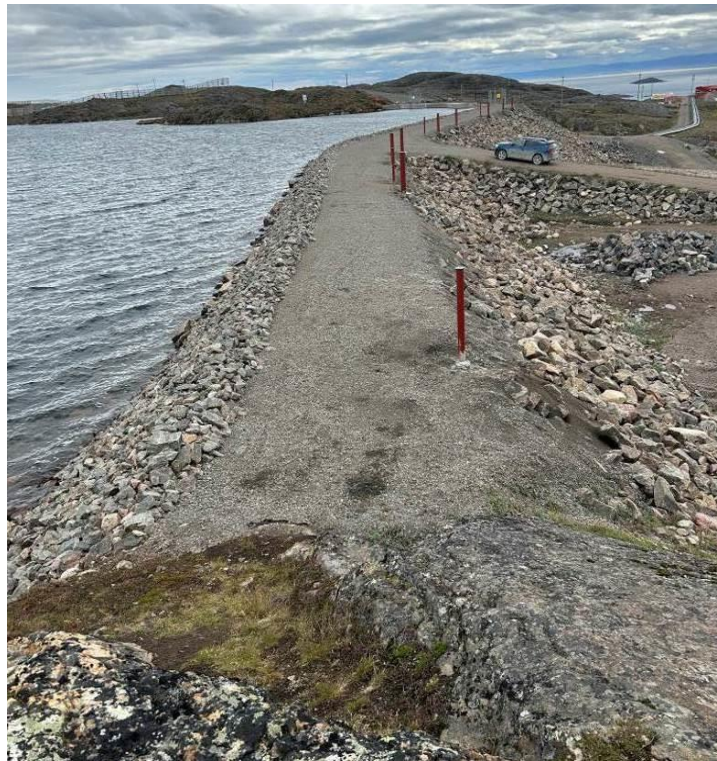
Photograph 3 – Typical north and center berm condition at the time of our review. Note the soil contamination in the foreground atop the berm.
