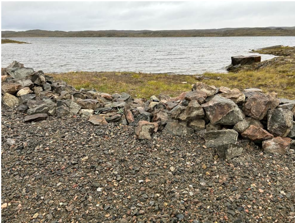
Photograph 6 – Section of the south berm where the rip-rap material on the upstream face of the dam has been displaced.
