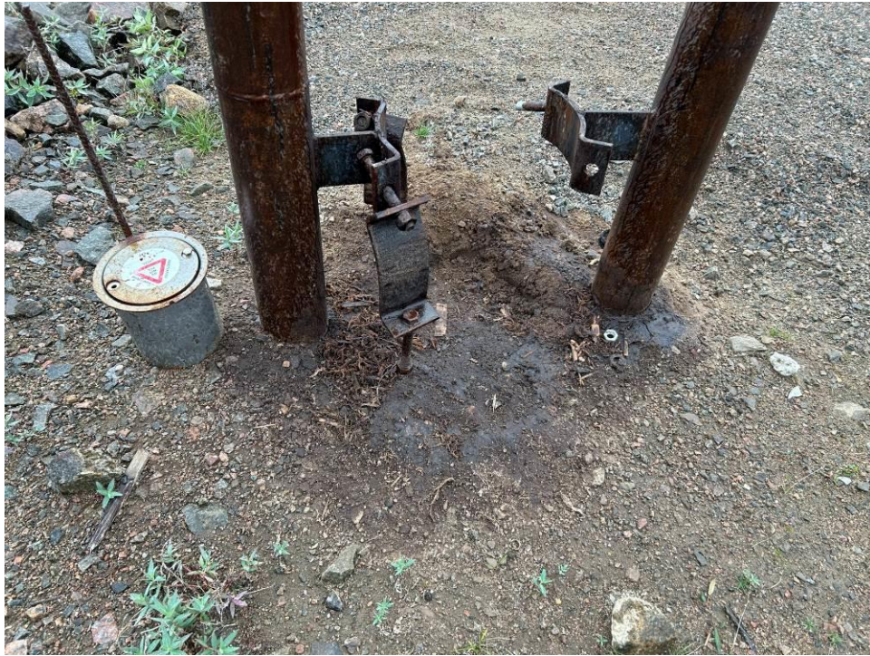
Photograph 5 – Oil residue on the ground from the hydro pole, that had been previously installed and removed.
