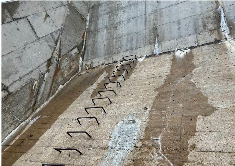
Photograph 9 – Seepage through the concrete dam.
