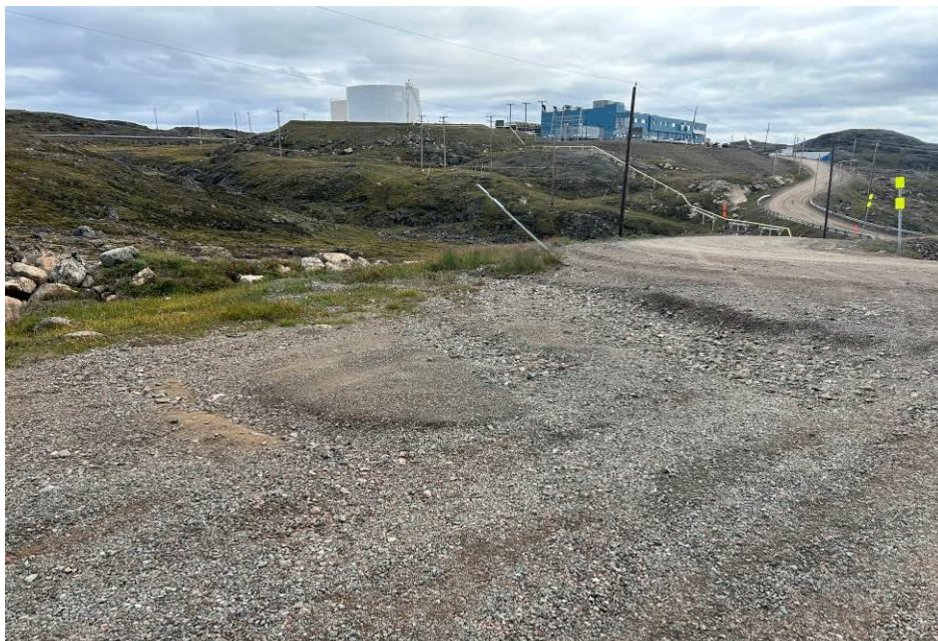
Photograph 4 – erosion of the north access road at the intersection with Takuminaqtuq Avenue.
