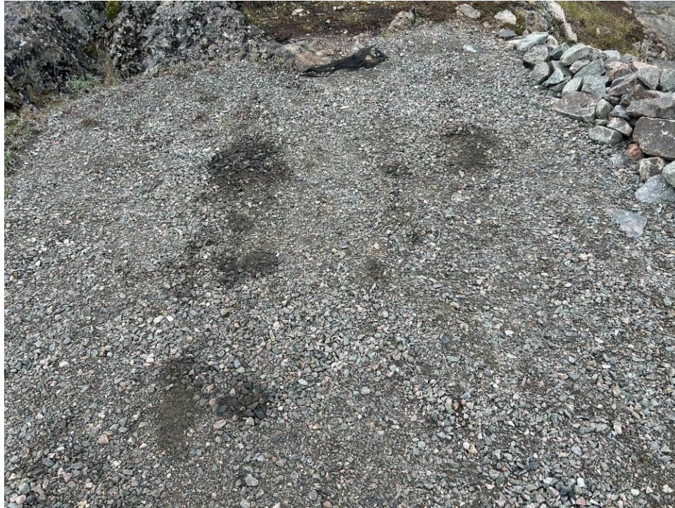
Photograph 7 – VOC contamination atop the north and center berms. The contractor responsible has been directed to remove and replace the contaminated material.
