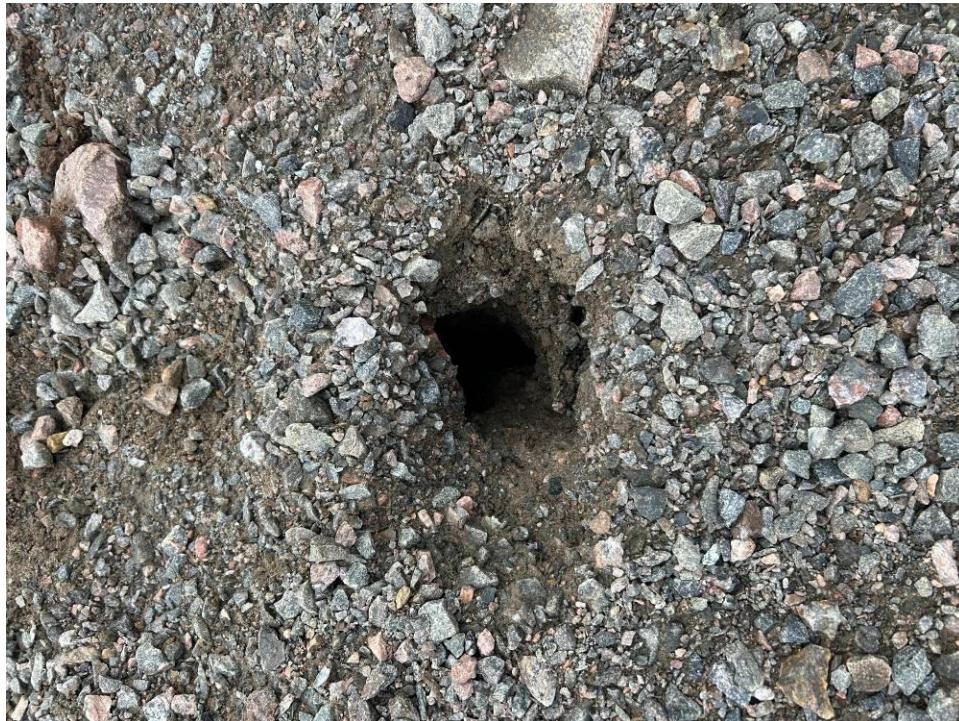
Photograph 8 – Small sink hole found in the top of the center berm.
