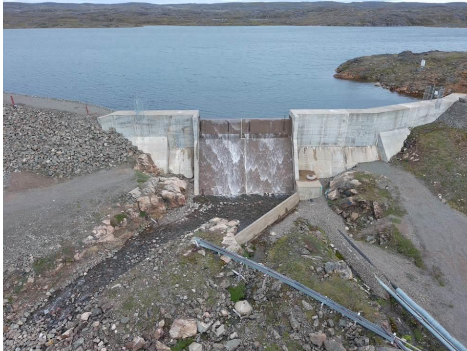
Photograph 1 – Overview of concrete dam and spillway.
