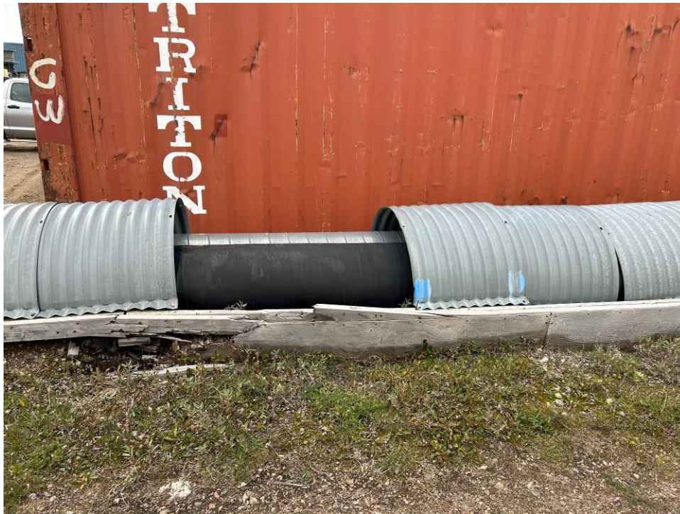
Photograph 11 – Section of the supply pipe from the dam with the corrugates metal enclosure removed.
