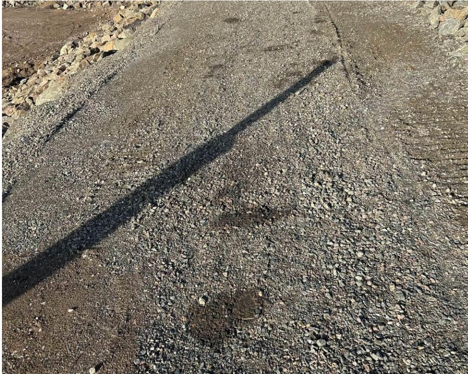
Photograph 8 – VOC contamination atop the center berm. The contractor responsible has been directed to remove and replace the contaminated material.
