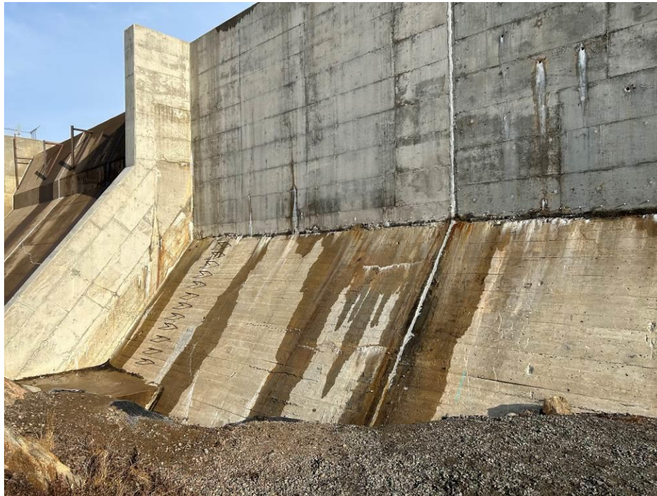
Photograph 10 – Seepage through the concrete dam.
