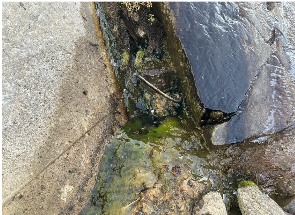
Photograph 11 – Seepage at the base of the concrete dam, note the water flow through the drainage tube.
