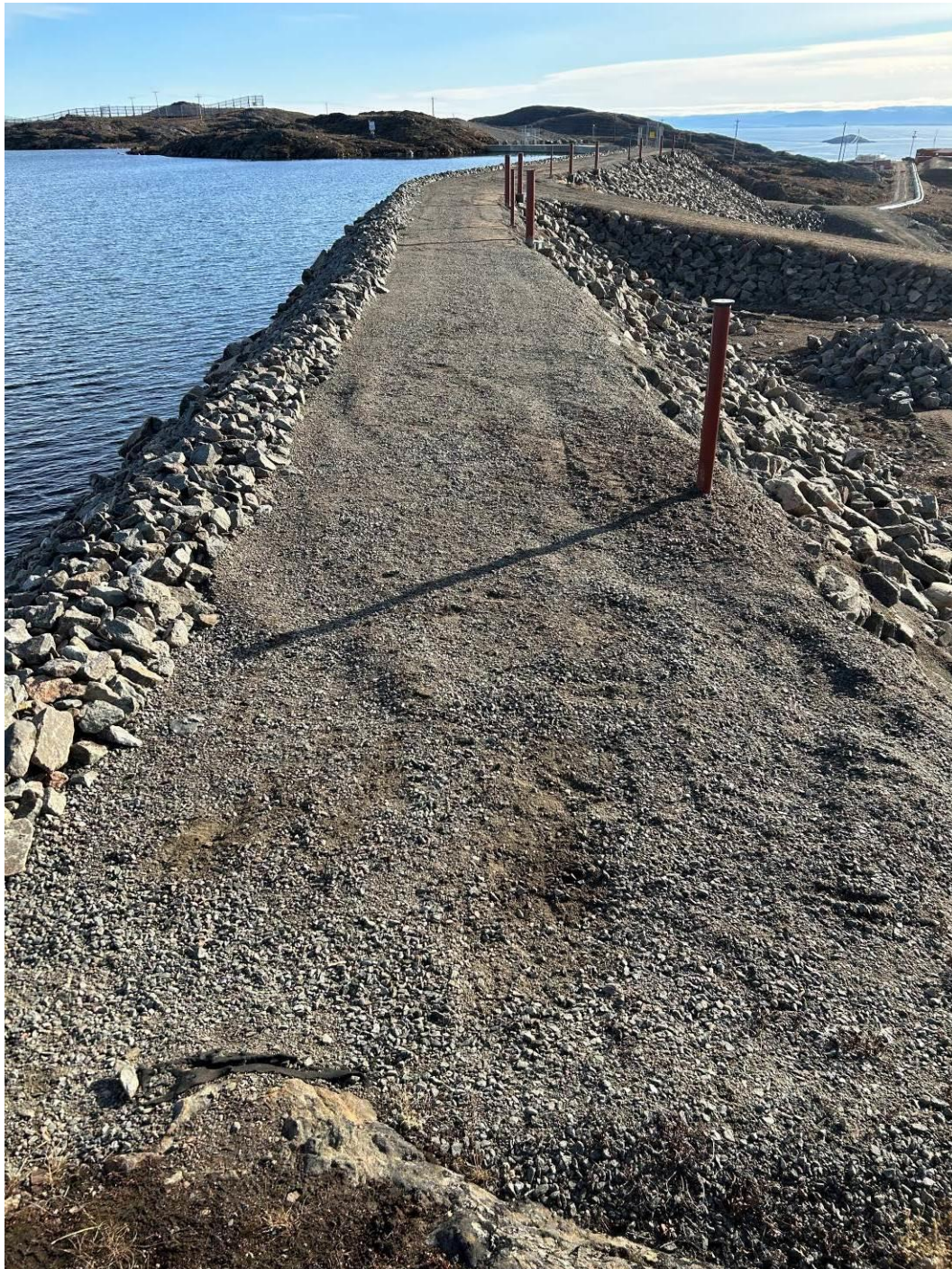
Photograph 3 – Typical north and center berm condition at the time of our review. Note the soil contamination in the foreground atop the berm.
