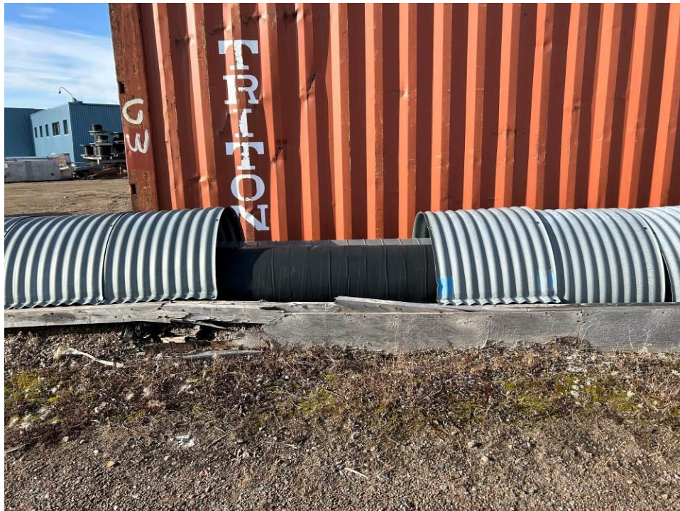
Photograph 15 – Section of the supply pipe from the dam with the corrugates metal enclosure removed.
