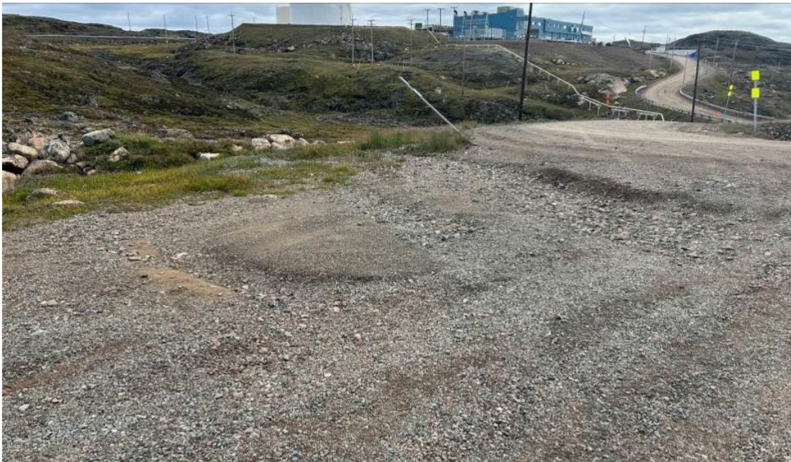
Photograph 4 – Erosion of the north access road at the intersection with Takuminaqtuq Avenue.
