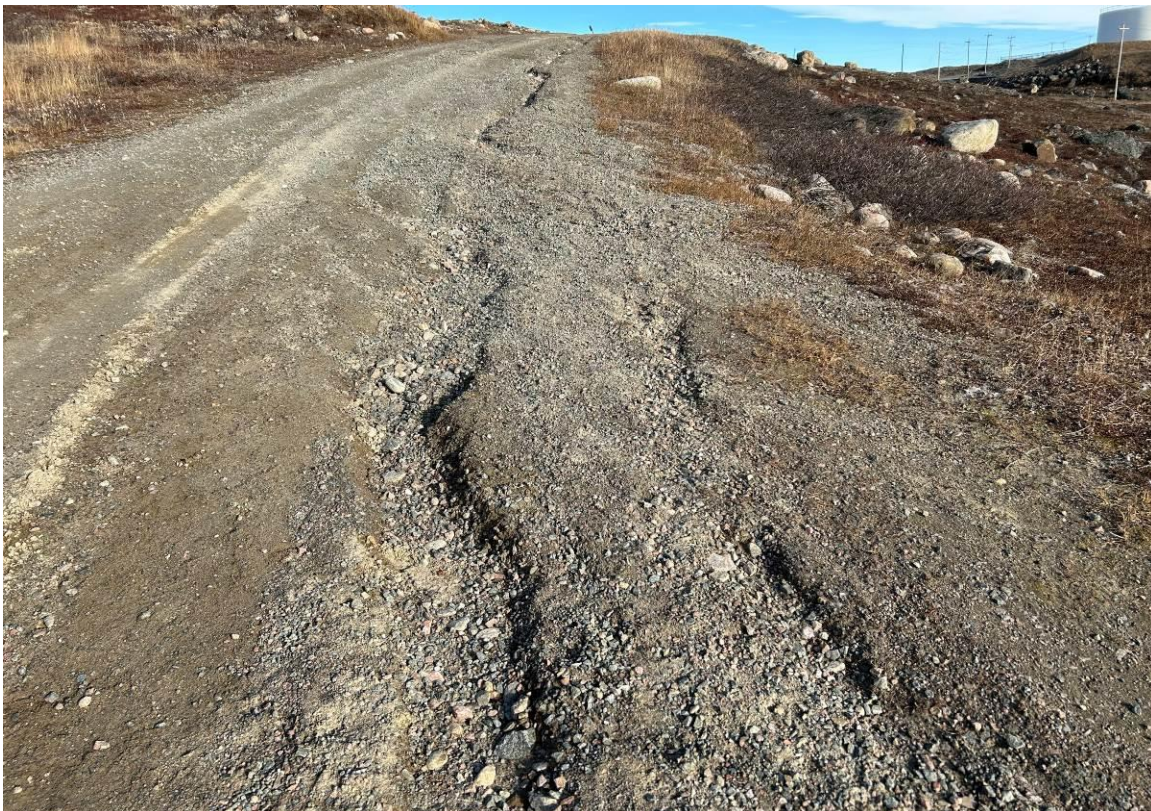
Photograph 5 – Erosion within the north access road.
