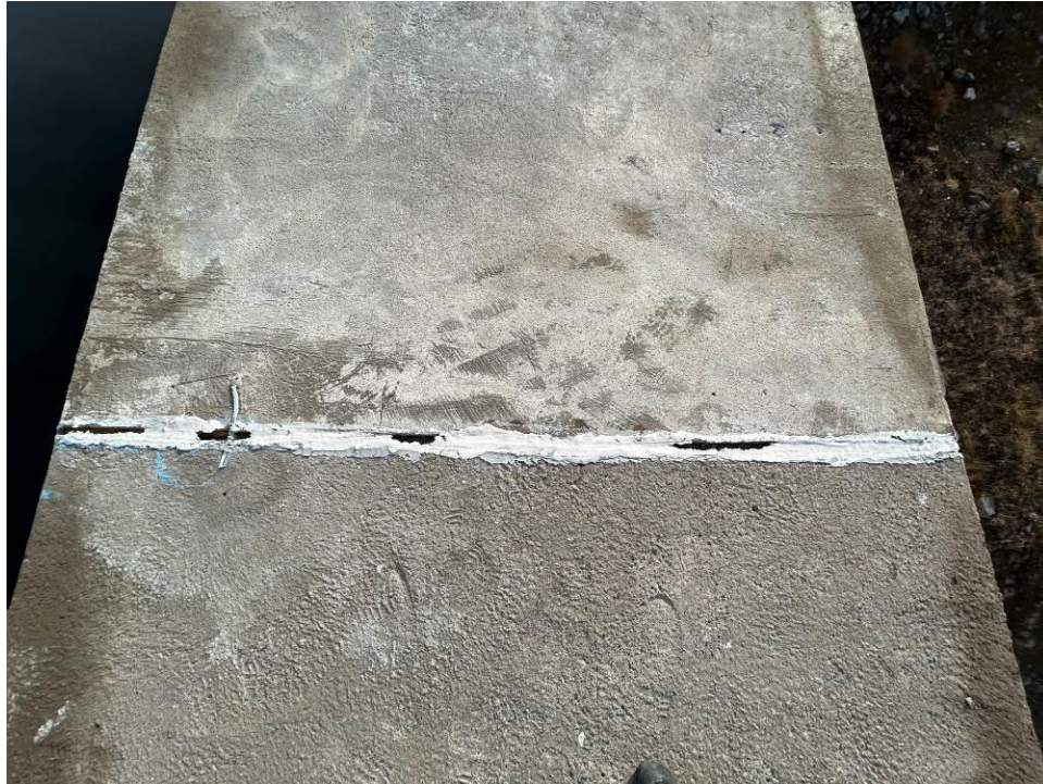
Photograph 12 – Deteriorated sealant material at the expansion joint.
