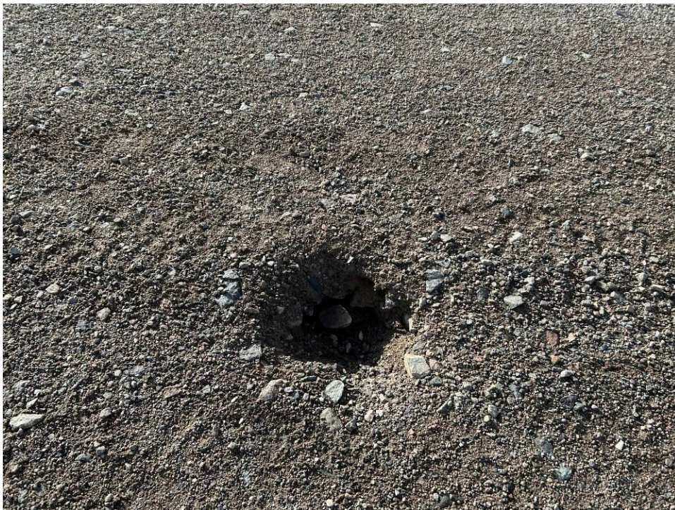
Photograph 9 – Small sink hole found within the south access road to the south berm.
