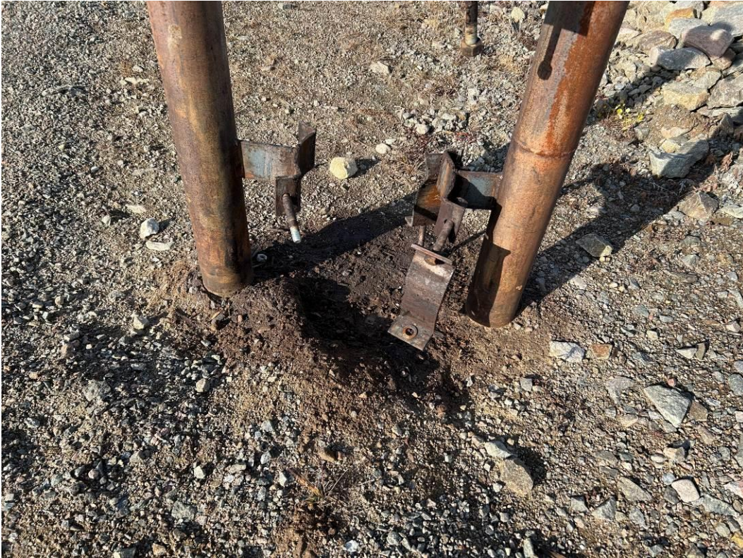
Photograph 6 – Oil residue on the ground from the hydro pole, that had been previously installed and removed.
