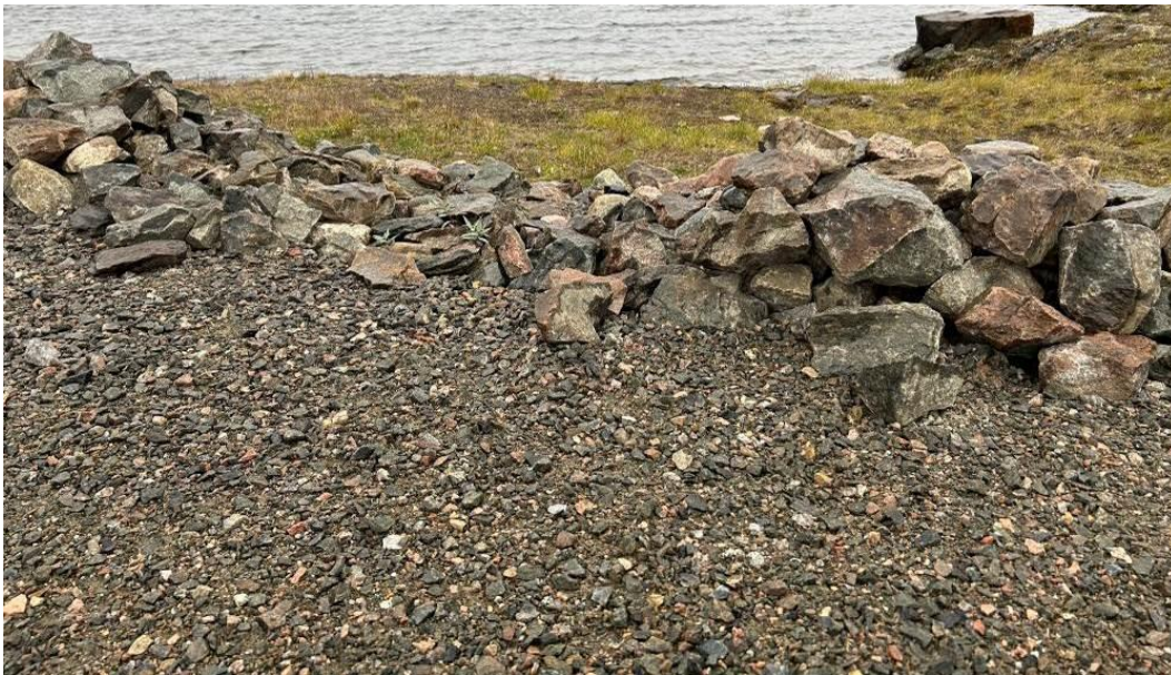
Photograph 7 – Section of the south berm where the rip-rap material on the upstream face of the dam has been displaced.
