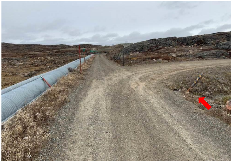
Photograph 13 – Corner marker at the junction of the south access road and the road to the south berm has been knocked over.
